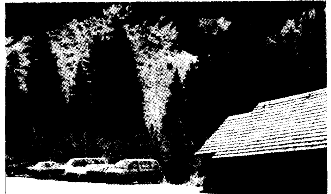
Paint Shed (formerly a comfort station).
