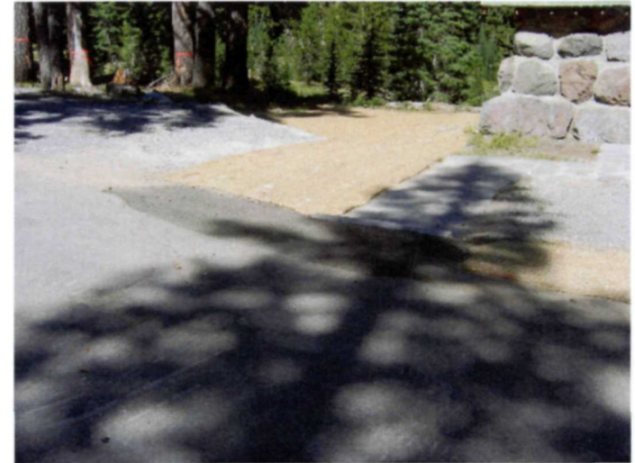
Photos 53-54 Extensive regrading, fill and asphalt removal is needed between the Naturalist's Residence and road. The gravel parking area should be removed, the road narrowed and moved away from the building, the flagstone path straightened and step removed, and the ground mounded and planted between building and road.
