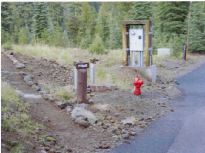
Photo 70 Fill and smooth transitions to conceal trail edge, utility vaults and concrete foundation of electricity meter.
