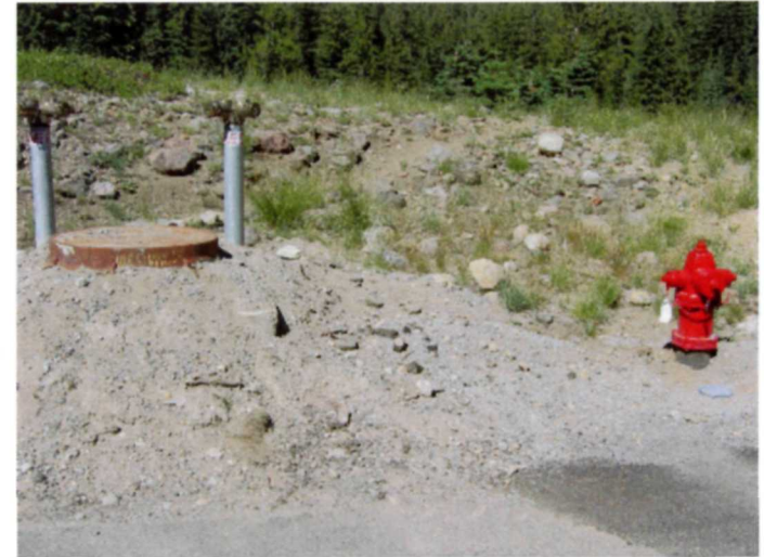
Photo 71 Exposed rim of manhole and crushed rock attract attention to an object that should be as unobtrusive as possible
