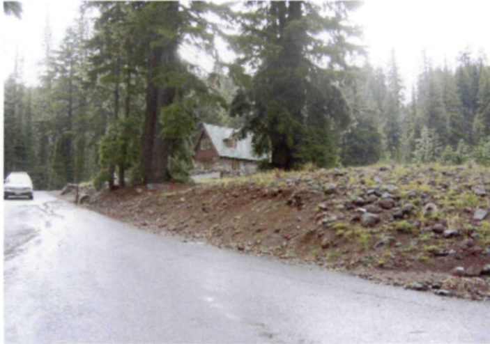
Photo 14 Cut bank along road at upper end of Historic District. Regrading banks such as this provided fill material for use throughout the district and eases the slope to merge with surrounding grades.
