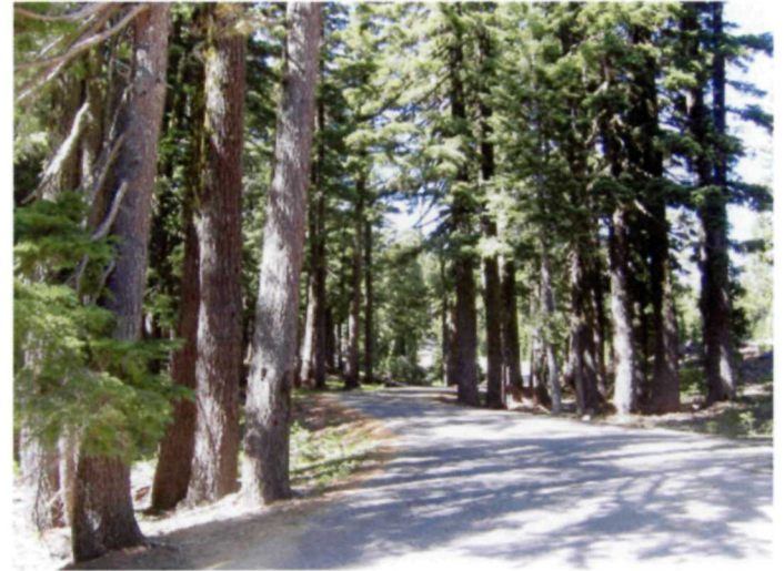
Photo 67 Road through forest shows well-graded profile of shoulders.
