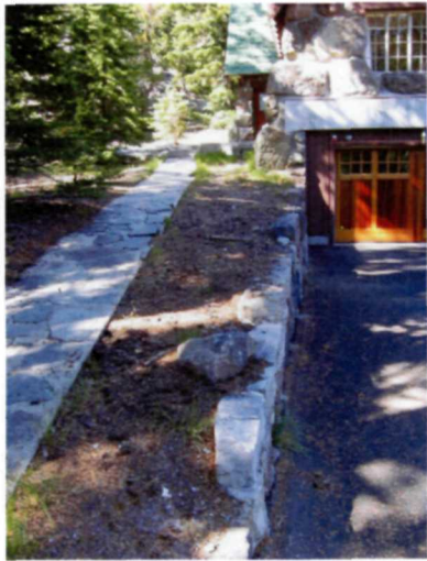
Photo 65 Mound along length of bed to redirect runoff across path and away from retaining wall.
