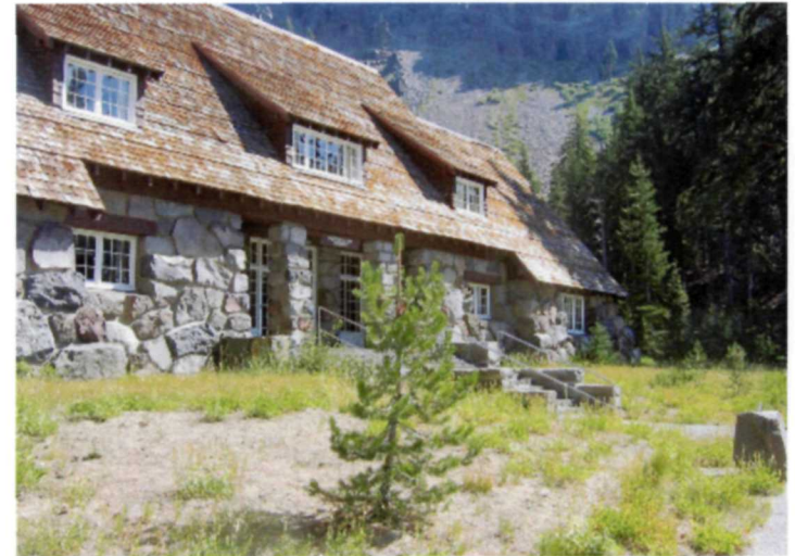
Photo 38 Firs at the corner of the Administration building effectively integrate it with the adjacent hemlock fir forest. Lodgepole pines in front of the building appear to be self-sown. Much of the bare ground is the result of gopher activity.
