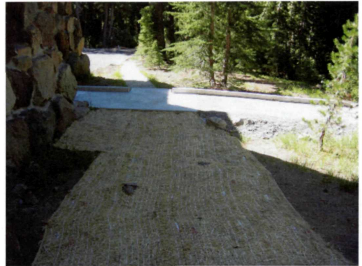
Photos 63 Extensive fill, in some locations several feet deep, and carefully placed large boulders adjacent to steps are needed to resolve the raw grading around the new steps and handicapped access ramp.
