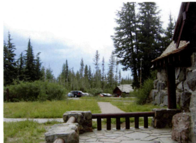
Photo 25 The view from the terrace to the start of the Historic District trail suggests that "you can't get there from here" rather than extends an invitation.
