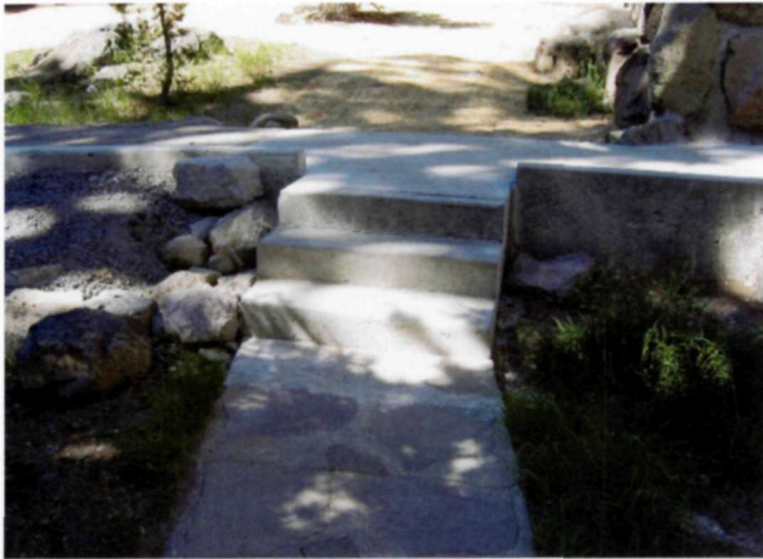
Photos 61-64 Extensive fill, in some locations several feet deep, and carefully placed large boulders adjacent to steps are needed to resolve the raw grading around the new steps and handicapped access ramp.
