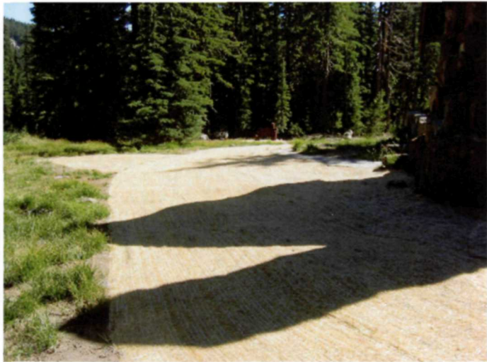
Photo 66 Erosion matting on flat surfaces is unnecessary. In this location on the meadow face, fill is needed to conceal pipes and to remove the hummocky ground surface.
