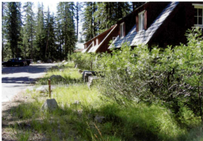
Photo 47 Cottage row along spur road note green roof of Dormitory building (old Hospital) at end.
