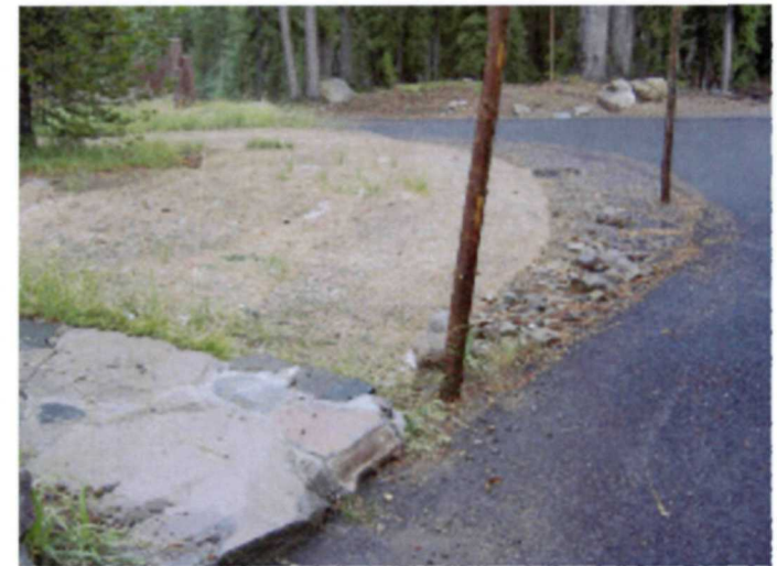
Photo 72 remove step from path to Superintendent's house and regrade swale.
