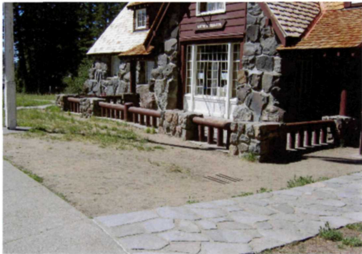
Photo 24 The bare and trampled bed in front of the Center conveys inappropriate messages about Crater Lake National Park, right on the Park's front doorstep.
