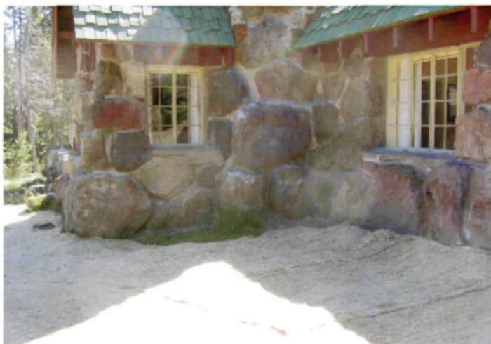
Photo 4 Superintendent's Residence: removal of grout debris, filling around base of walls and pipes, and removal of unnecessary erosion control matting will integrate the building into the surrounding landscape.
