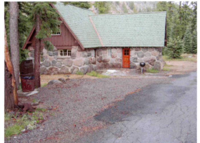
Photo 50 Arriving at the house it appears isolated from the forest and dominated by the proximity of the road and gravel parking area.
