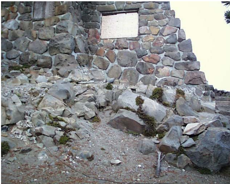
Contemporary photograph showing detail of Watchman Observation Station's foundation (CCSO 2001).
