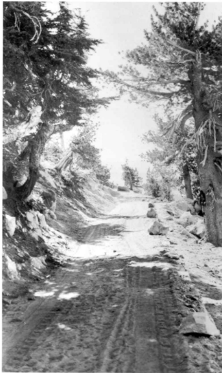
Historic photograph showing Watchman Trail is lined with rock on the down slope side of the trail, 1932 (CRLA archives).
