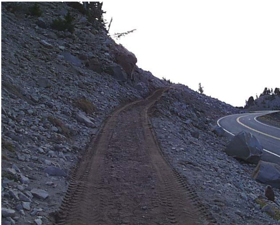
Contemporary photograph showing Watchman Trail. The trail is wider along this 200 yard segment as it traces the original alignment of Rim Road (CCSO 2001).
