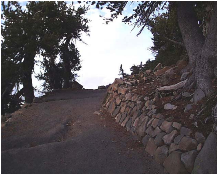
Contemporary photograph showing dry-laid retaining wall along Watchman Trail. This is a typical example of wall found along the trail (CCSO 2001).
