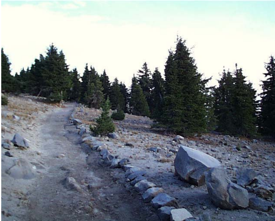
Contemporary photograph showing Watchman Trail. The trail is 5' wide and lined with stones during the historic period to mark its edge on the down slope (CCSO 2001).
