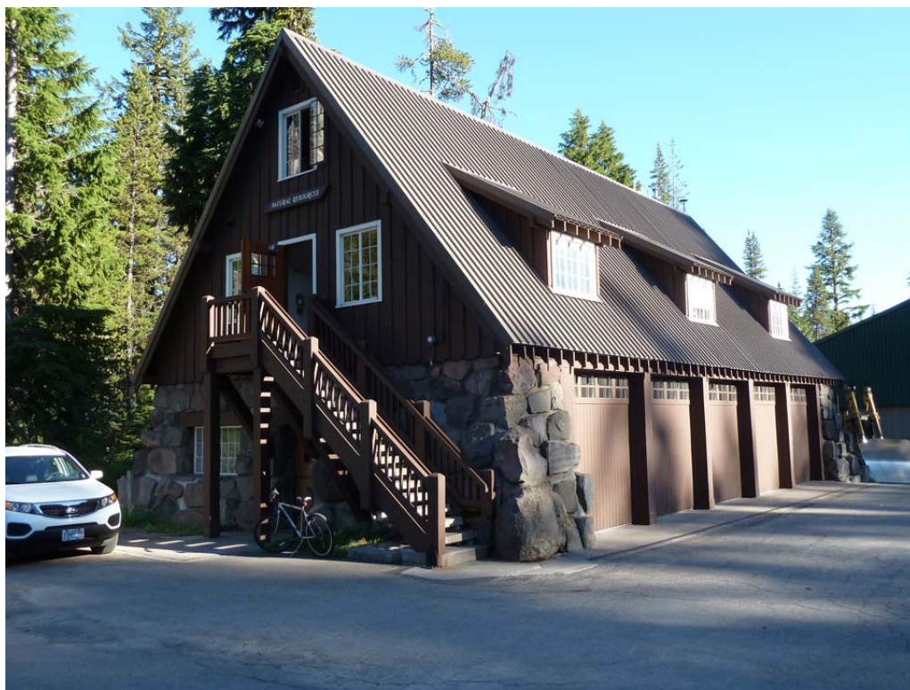
B&S #5: The Machine Shop, looking south, showing the five bays below and shed dormers upstairs (PWR, CL Program, 2012).
