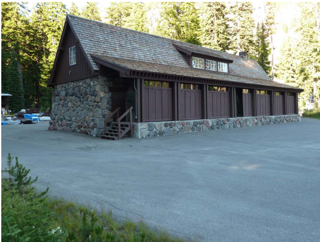
B&S #4: The Warehouse, looking northwest, showing the covered loading area now enclosed. Note the earlier use of smaller stone masonry along the first floor (PWR, CL Program, 2012).
