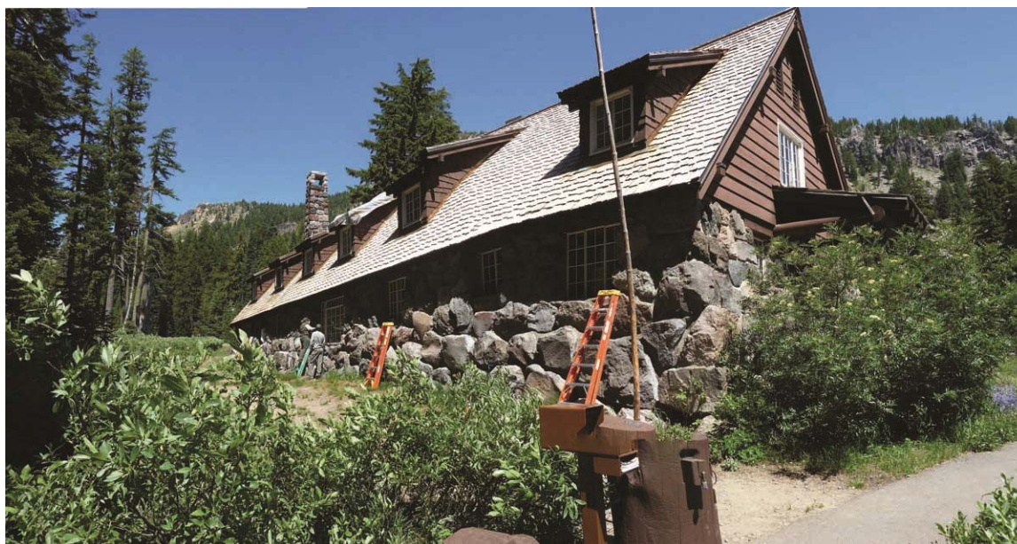
B&S #2: The back of the Ranger Dorm, looking north, showing the shed dormers and maintenance work on the windows (PWR, CL Program, 2012).
