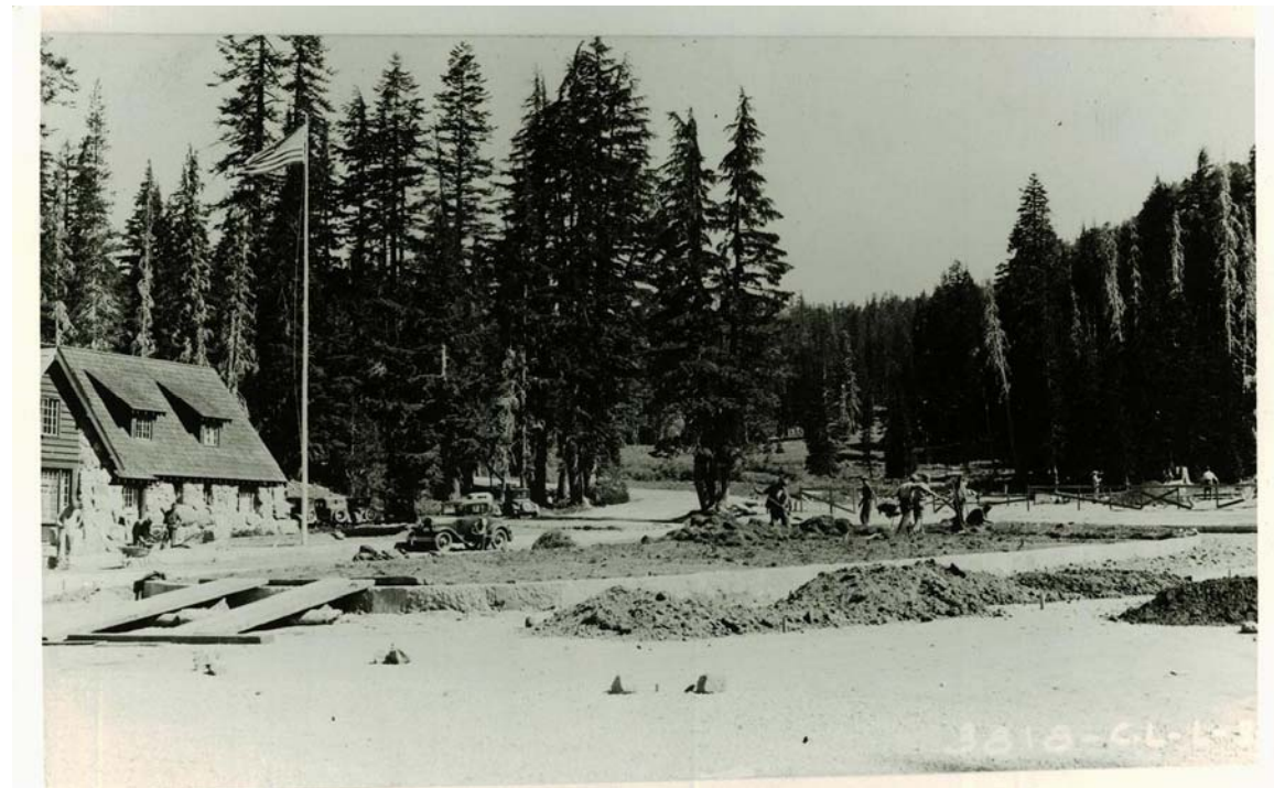
History #9: Looking north at the Parking Ellipse during construction, circa 1934. The Ranger Dorm and flag pole are located on the left. (CRLA 467502).
