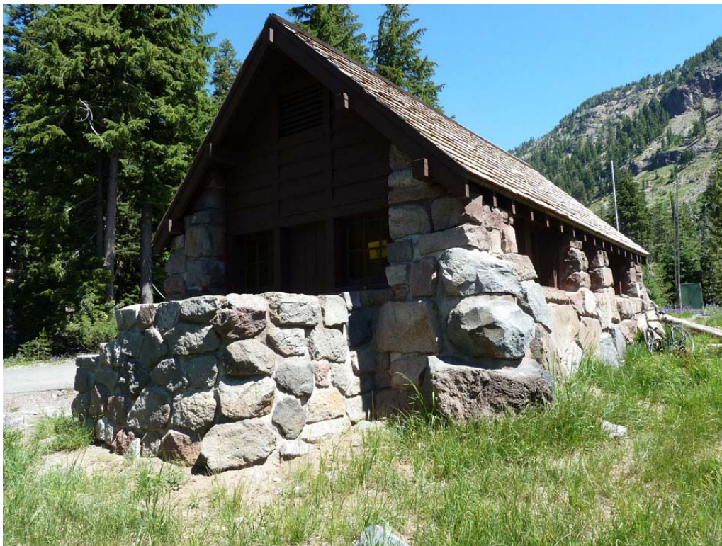
B&S #16: The Comfort Station, looking north. Note the massive stone masonry battered corners (PWR, CL Program, 2012).
