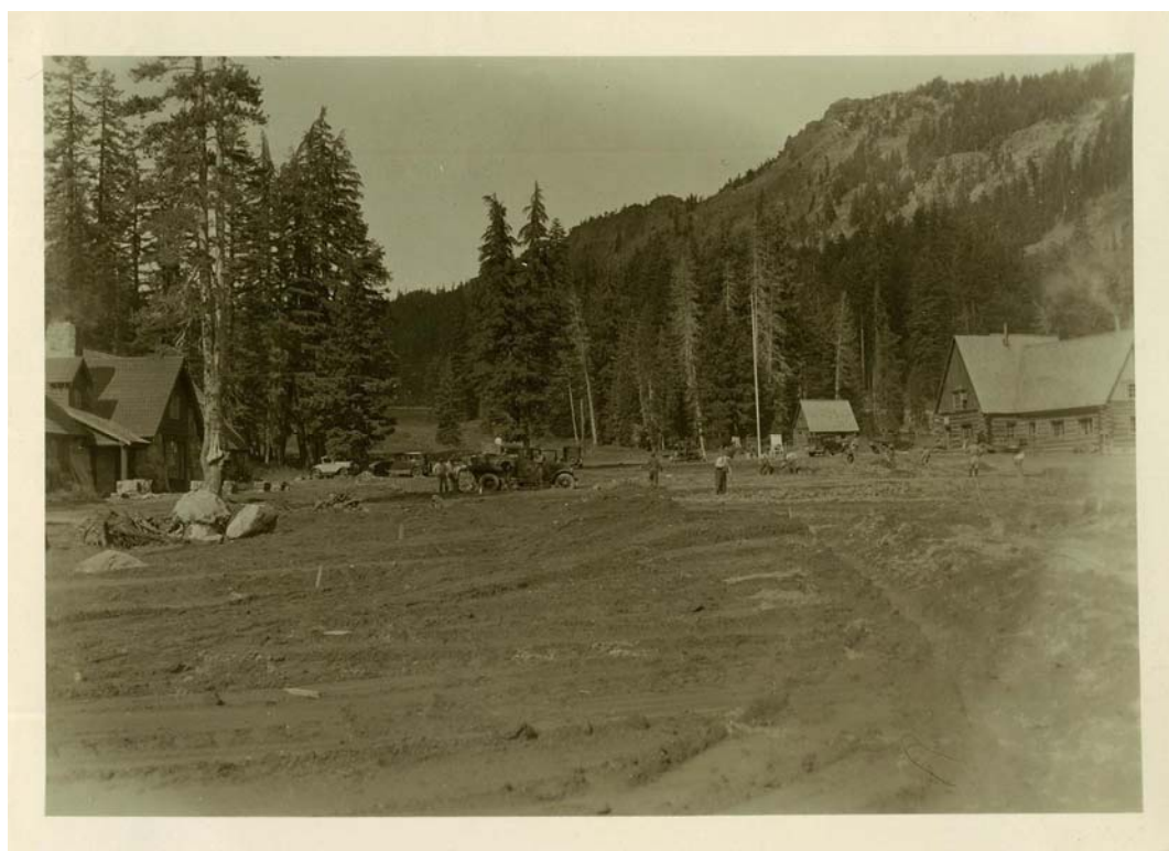
History #4: Looking north at the construction of the new headquarter's area, circa 1930s. Note the new Ranger Dorm already finished on the left and the clear view of Garfield Ridge in the background on the right (CRLA 467231).
