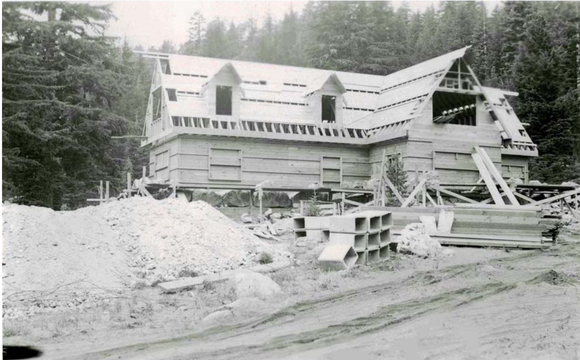
History #5: Looking northeast at the Superintendent's residence under construction, circa 1932. Note the lumber protection fence around the small conifer trees and the effort involved to ensure the residence blends in with the landscape. (CRLA 467005).
