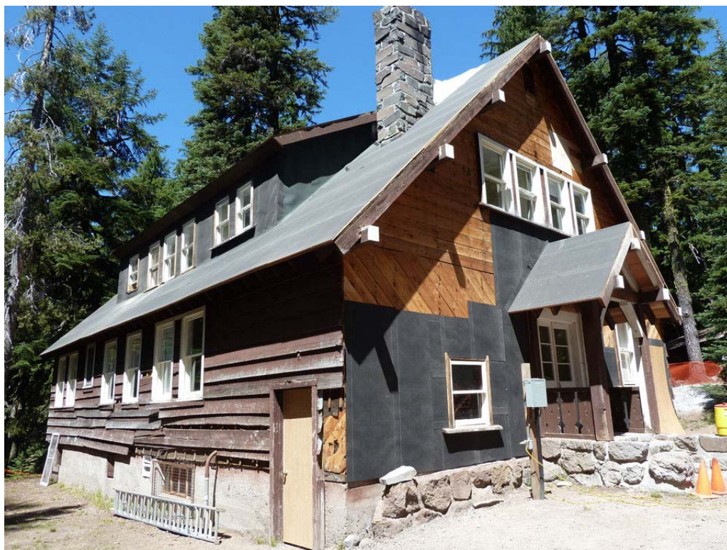
B&S #14: The Hospital under repair, looking northeast. Note the exposed concrete foundation on the left and the stone facing on the right (PWR, CL Program, 2012).
