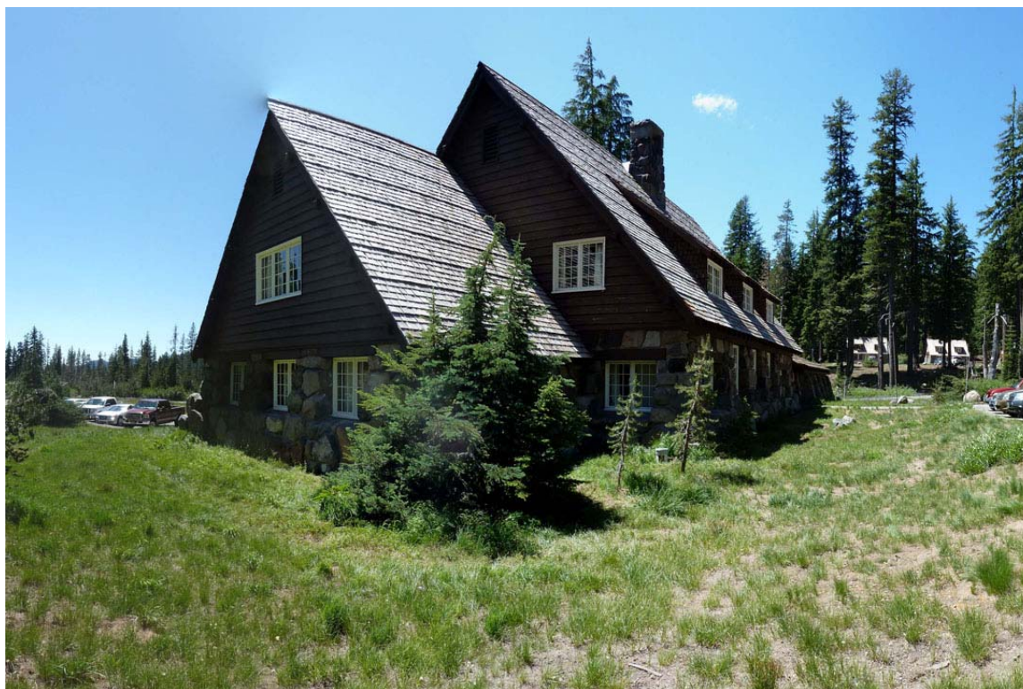
B&S #1: The back side of the Administration Building, looking southeast, showing the roof line and shed roof dormers (PWR, CL Program, 2012).
