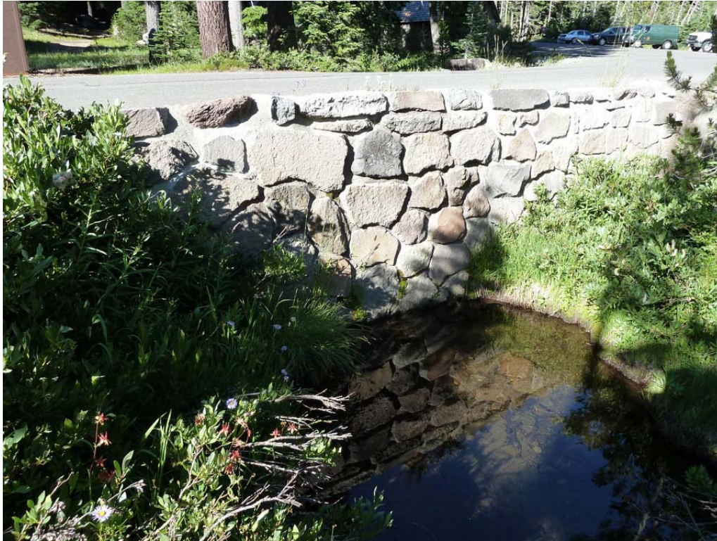
Small-Scale Features #2: The culvert located southwest of the Mess Hall featuring a large masonry headwall, looking northwest. Note the outfall is below water level (PWR, CL Program, 2012).
