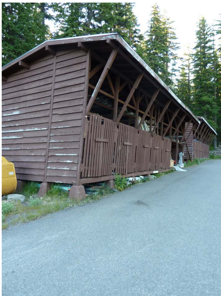
B&S #17: The Lumber Sheds, looking north, building 9 is in the center of the photograph and building 10 is in the background on the right (PWR, CL Program, 2012).
