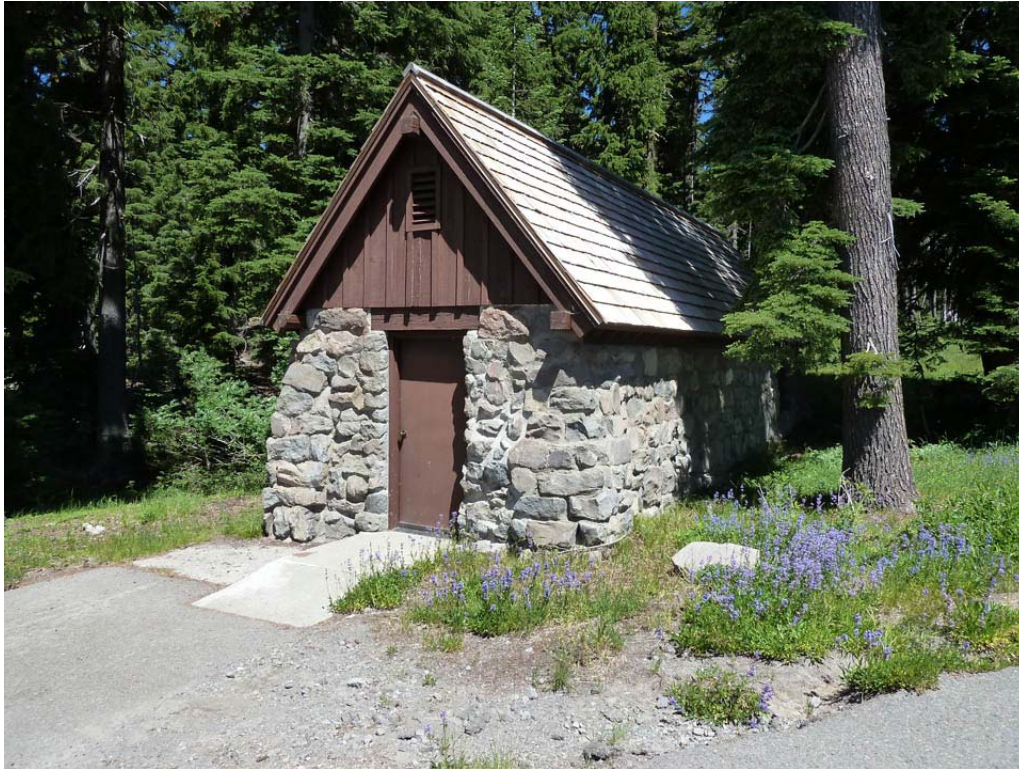
B&S #15: The Transformer Building, looking northeast. Note the battered small stone masonry and corners, a characteristic of rustic architecture. (PWR, CL Program, 2012)
