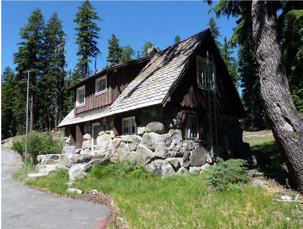
B&S #11: Employee Residence #28, looking northeast, showing the main entrance and stone patio to the left (PWR, CL Program, 2012).
