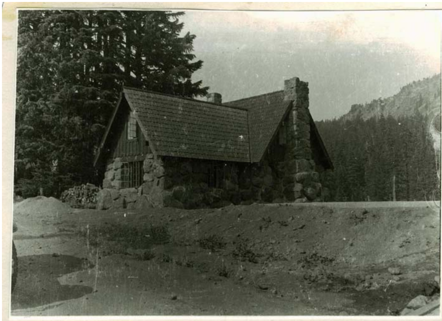
History #6: Looking north at the Naturalist's residence after construction and just before planting of the landscape, circa 1933. Note the orientation of the residence toward the view of Garfield Ridge, seen in the background on the right (CRLA 467289).
