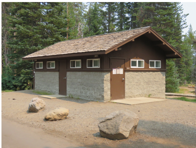
Comfort Station 62, view northeast.
