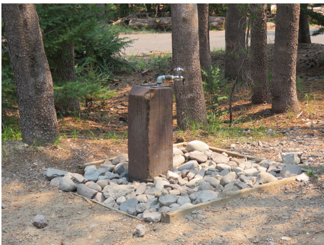
Typical water station in Mazama Campground (this example located in Loop B), view east.
