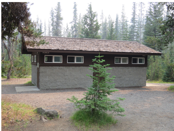
Comfort Station 63, view south.
