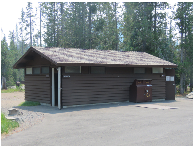
Comfort Station 58, view south.
