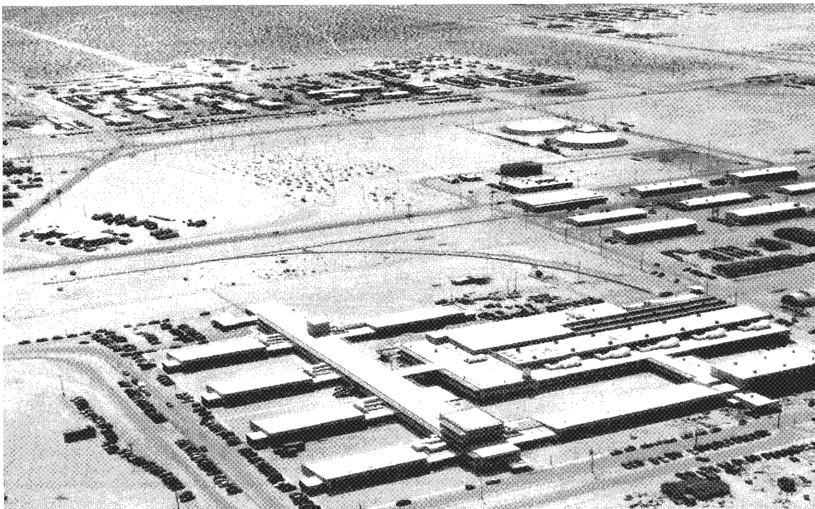
Figure 32. Michelson Laboratory, NAWS China Lake. Completed in 1948, it set the standard for integrated laboratories at the Navy, as well as other branches. Architecturally, the Michelson Laboratory plan, with a long central corridor and projecting wings, was copied on other bases. (Source: the National Archives.)
