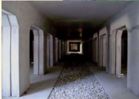
Figure 7. Top: Sun Valley Park vegetated swales. Bottom: underground infiltration gallery. (Source: Los Angeles County Flood Control District)
