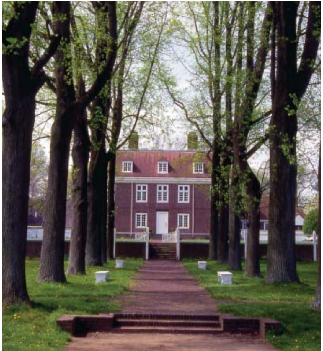
William Penn's Delaware River home was reconstructed in the late 1930s.
