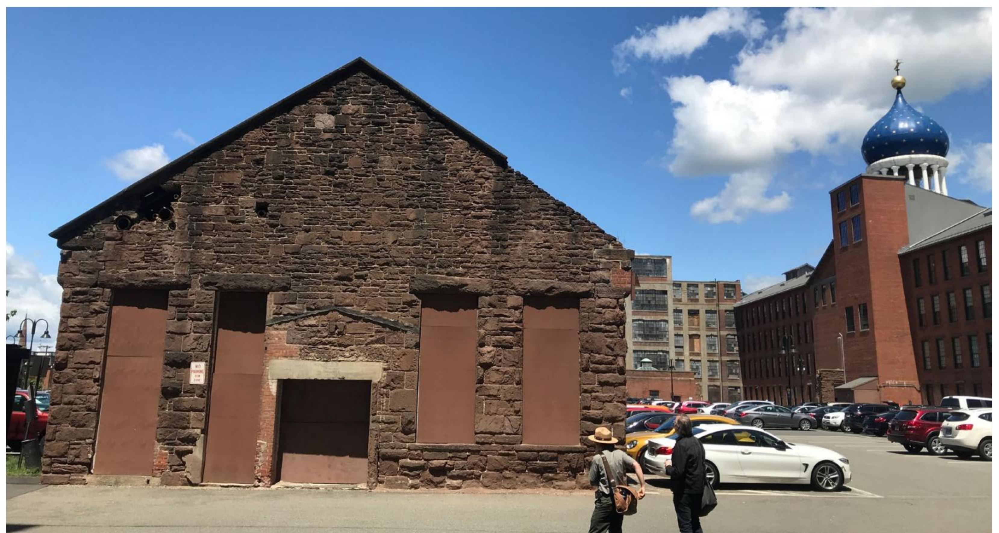
Site visit, Building 10 Colt Armory, Hartford, CT, June 2018
