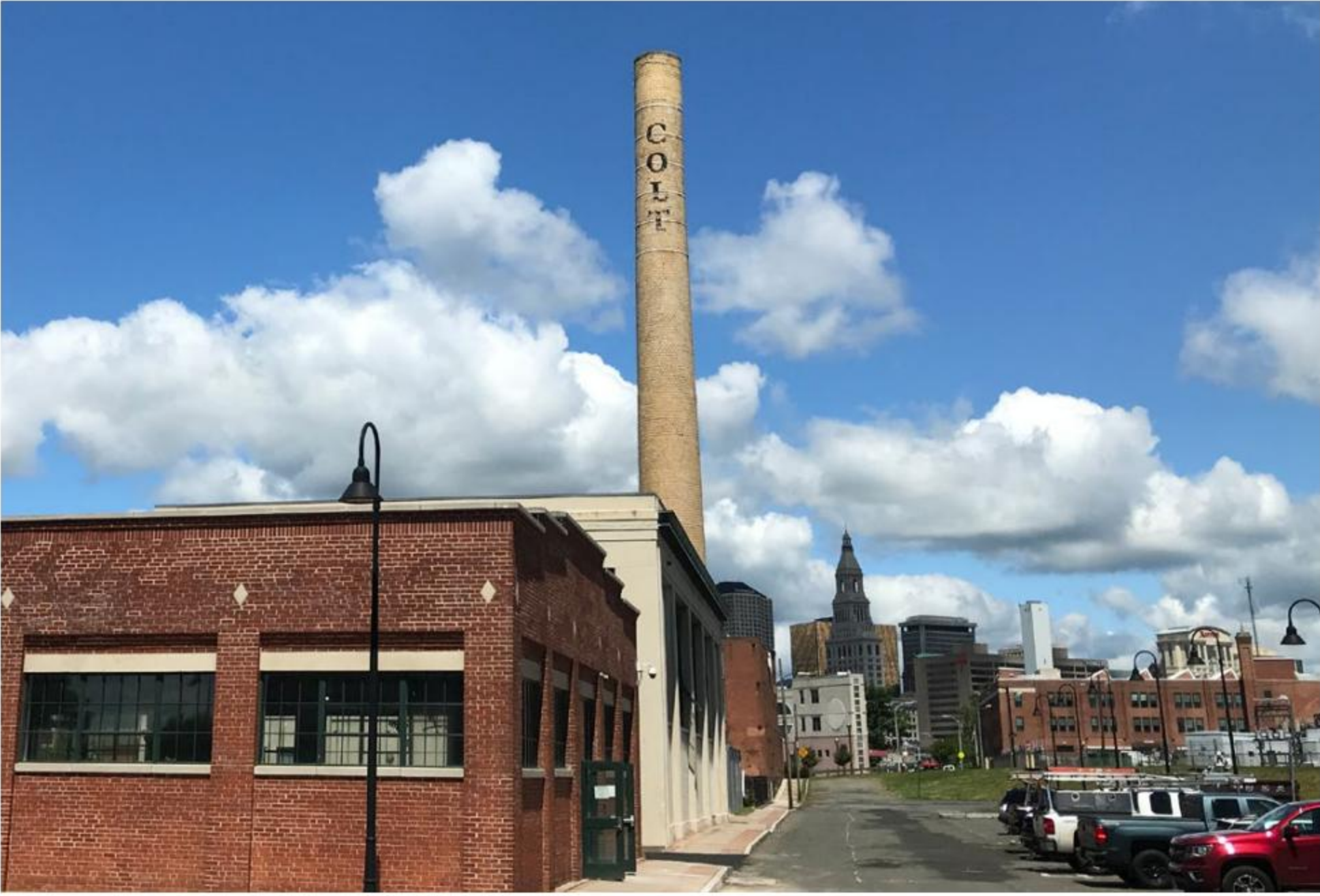
COLT Power Plant
