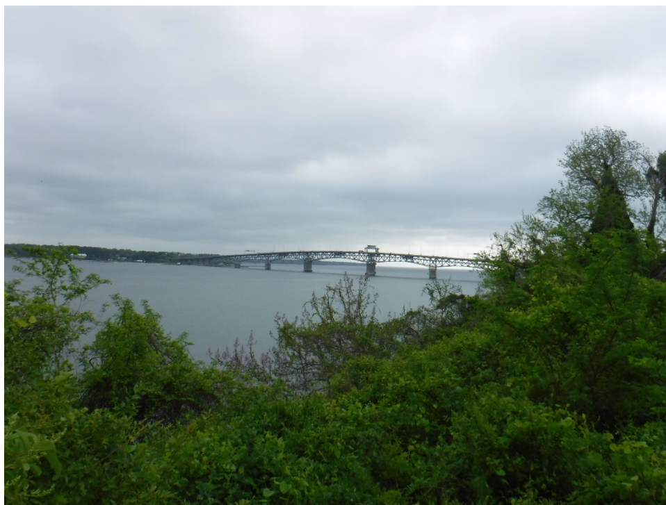
View from Welsh Fusiliers Redoubt towards Coleman Bridge (Wes Stewart, 4/20/2017)
