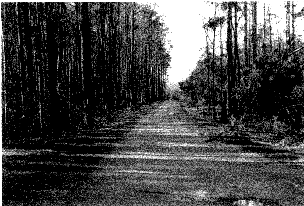
Monticello Avenue extension under construction in 1999 (NPS 1999).
