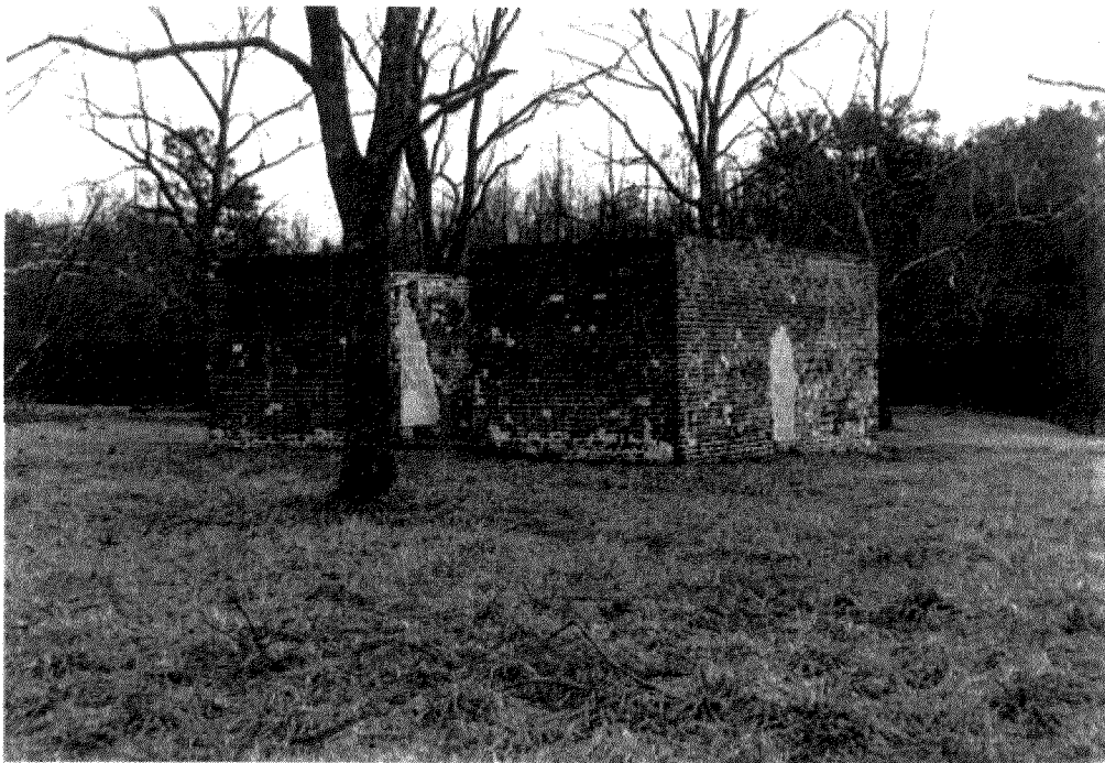
Standing ruin of brick outbuilding or 'jail' (NPS 1999).
