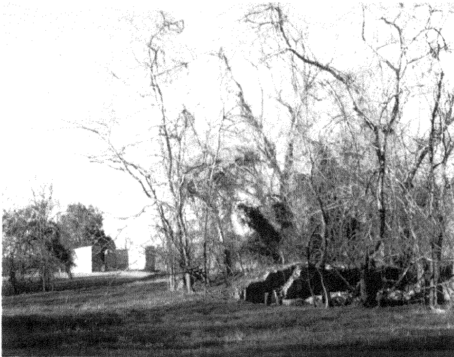
Standing ruin of orangery in foreground and ruin of brick outbuilding or 'jail' in background (NPS 1998)
