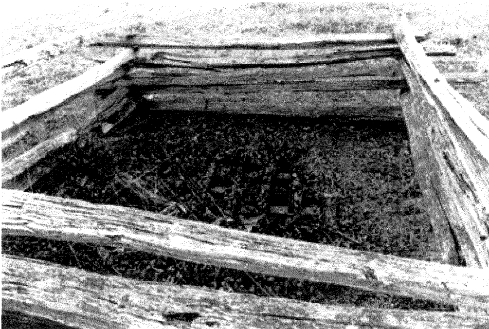
Wooden fence and metal grate used to protect the well (NPS 1999).
