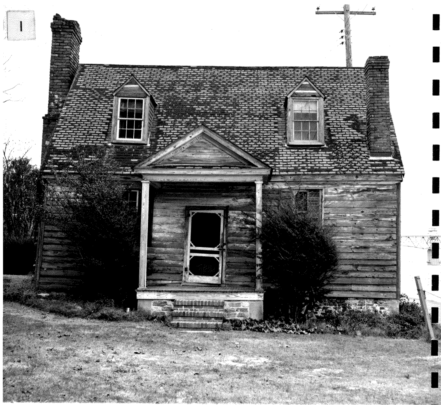
The south front elevation may have been the "entrance" since the door opening on north front appears to have been added, at least it is not framed like the above. The "modern" porch and riverside chimney were removed during the architectural investigation (middle of April 1958).
