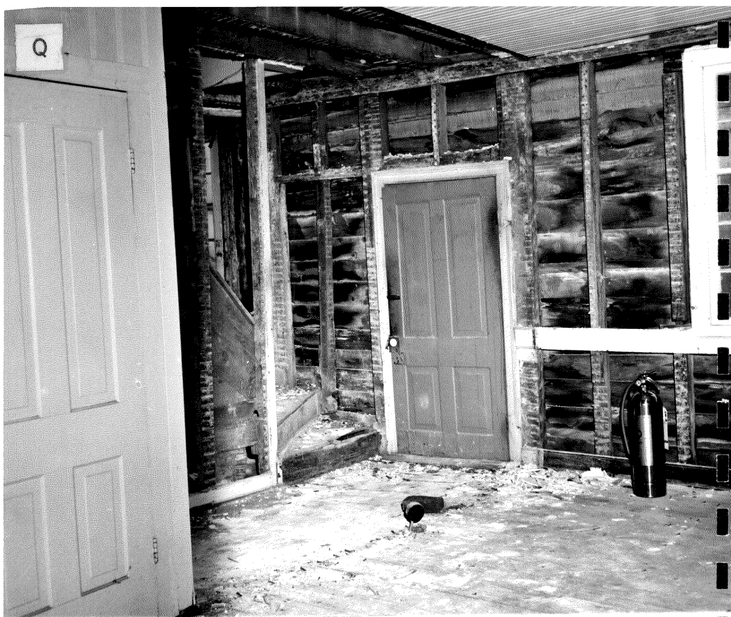
West room, looking toward entrance door, the partition and door at left are of the 1913 remodelling.
