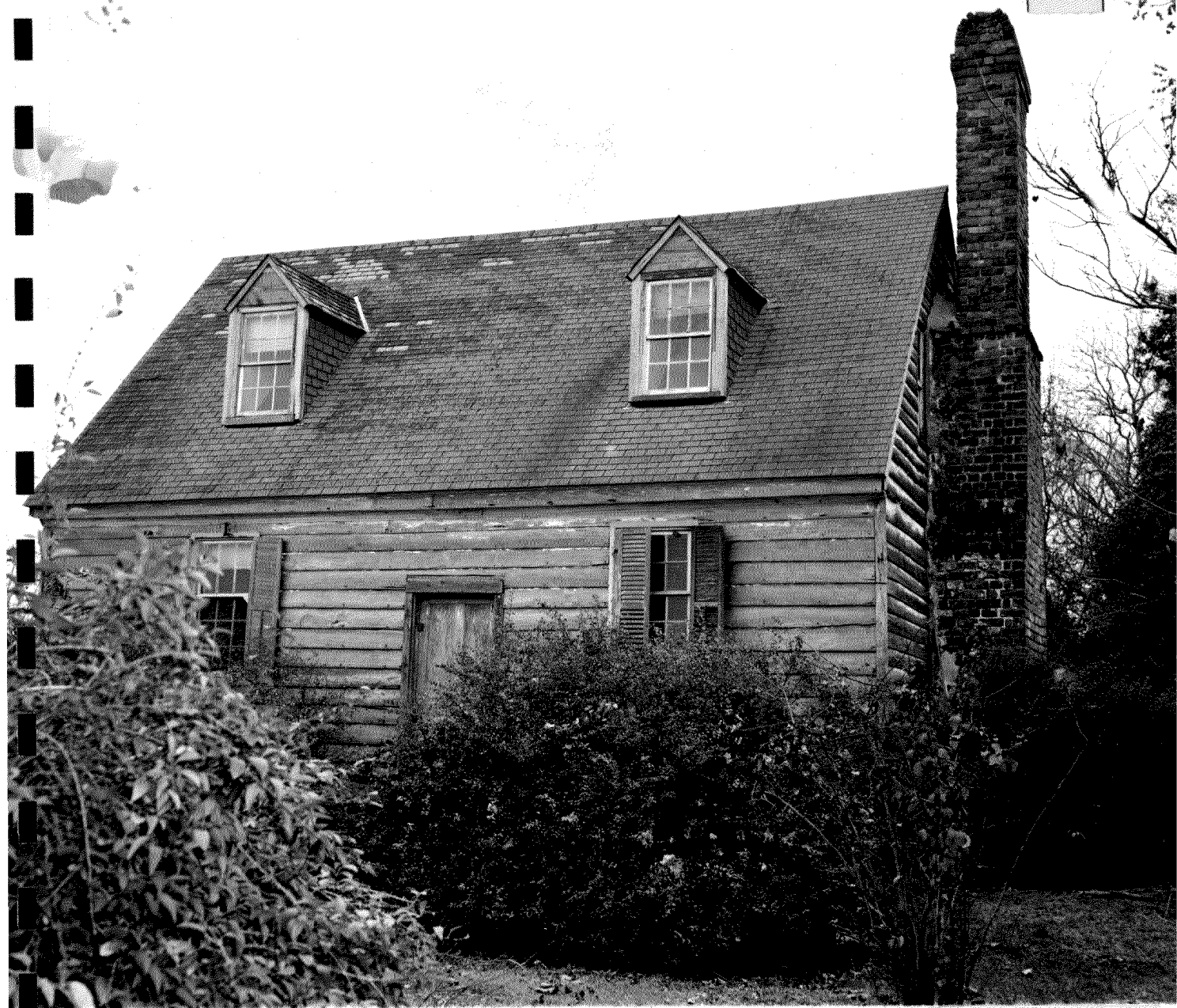
The west end and north front elevations present a pleasing composition typical of the small house dating from late 18th century to first quarter of the 19th century. The historical records and architectural research indicates the whole structure above ground was built after the fire of 1814 on an earlier foundation of about same dimensions.
