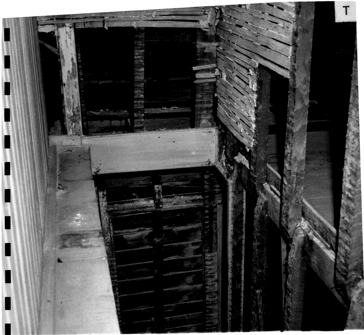
At left evidence remains of the original "hand rail."
