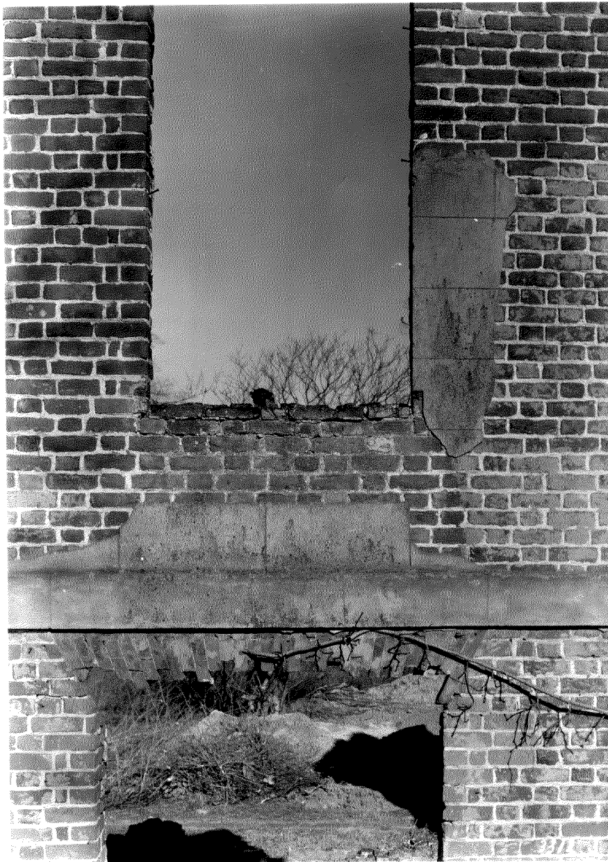
Photograph #15 - Ambler House, Jamestown Island -
