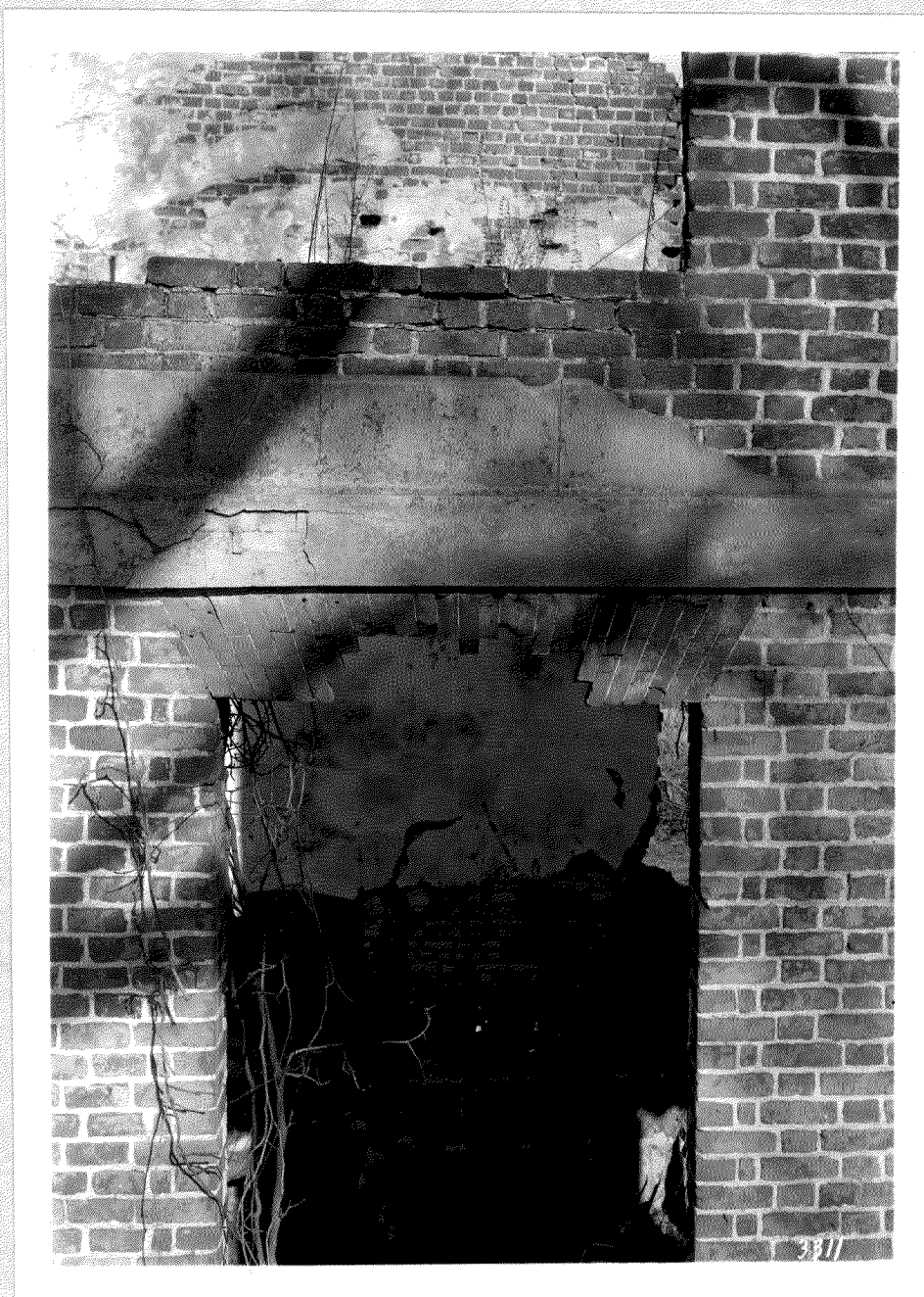
Photograph #14 - Ambler House, Jamestown Island - Detail of arch above the window and the lower part of the second floor window.
