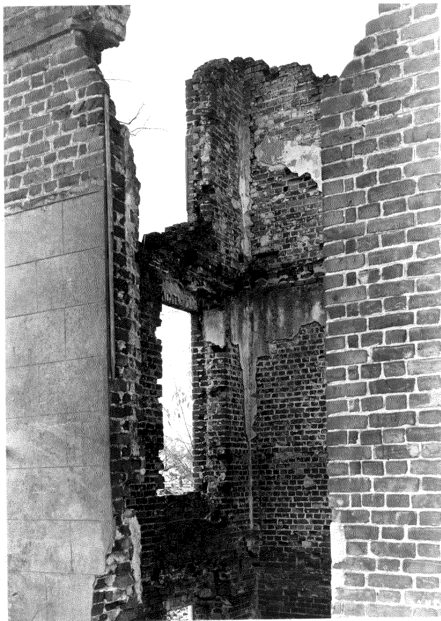
Photograph #13 - Ambler House, Jamestown Island -
