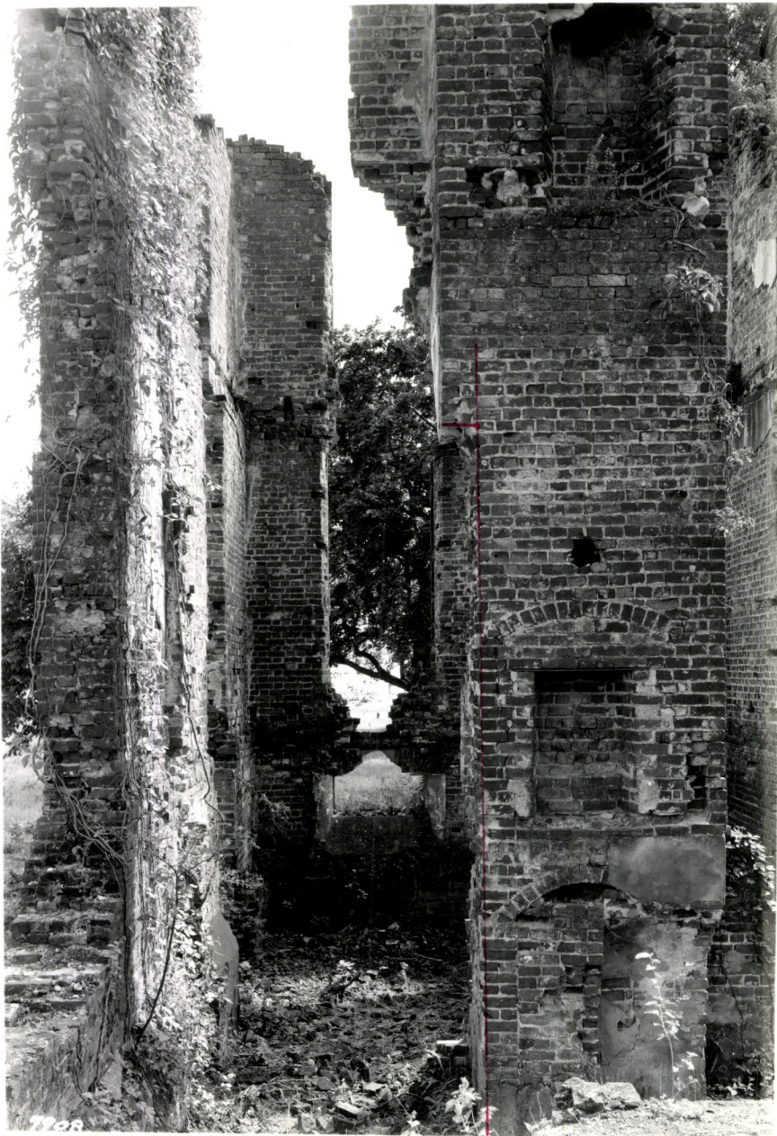
Photograph #20 - Ambler House, Jamestown Island -
