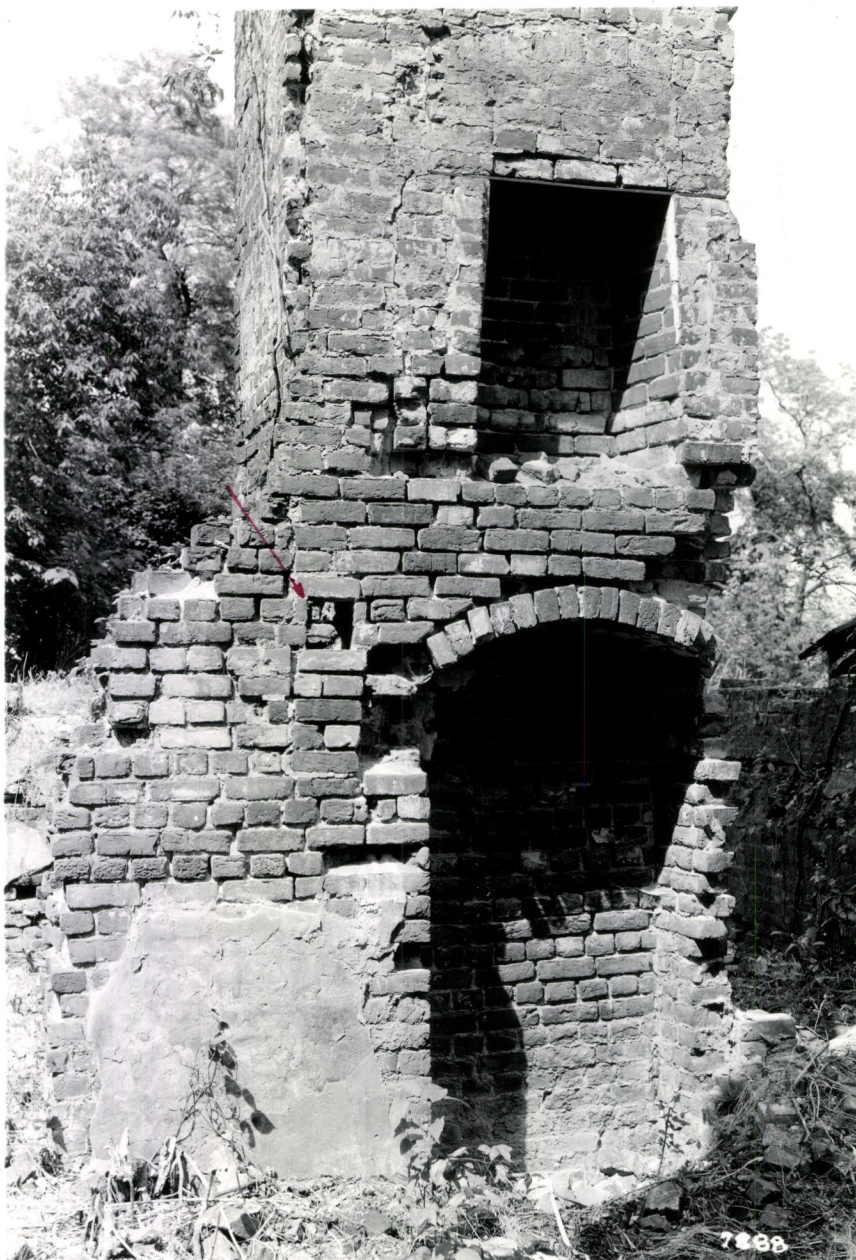
Photograph #23 - Ambler House, Jamestown Island -
