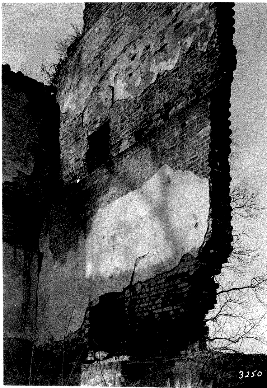
Photograph #28 - Ambler House, Jamestown Island -
