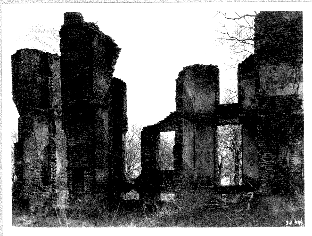
Photograph #7 - Ambler House, Jamestown Island - Interior view of rear. Taken from northwest corner.
