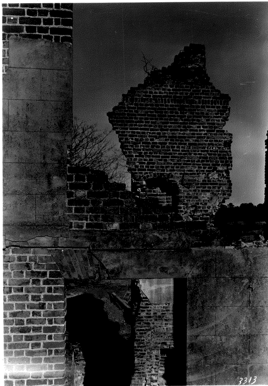
Photograph #25 - Ambler House, Jamestown Island -
