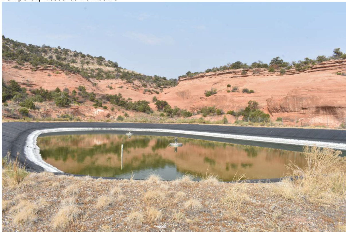
9_3. South Wastewater Lagoon, view southwest, July 12, 2021.
