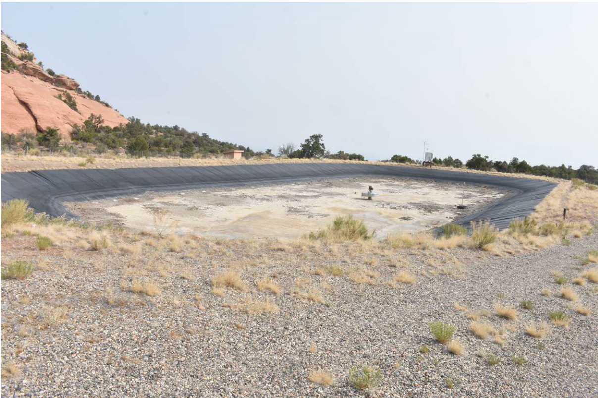
9_2. North Pumphouse and North Wastewater Lagoon, view north, July 12, 2021.
