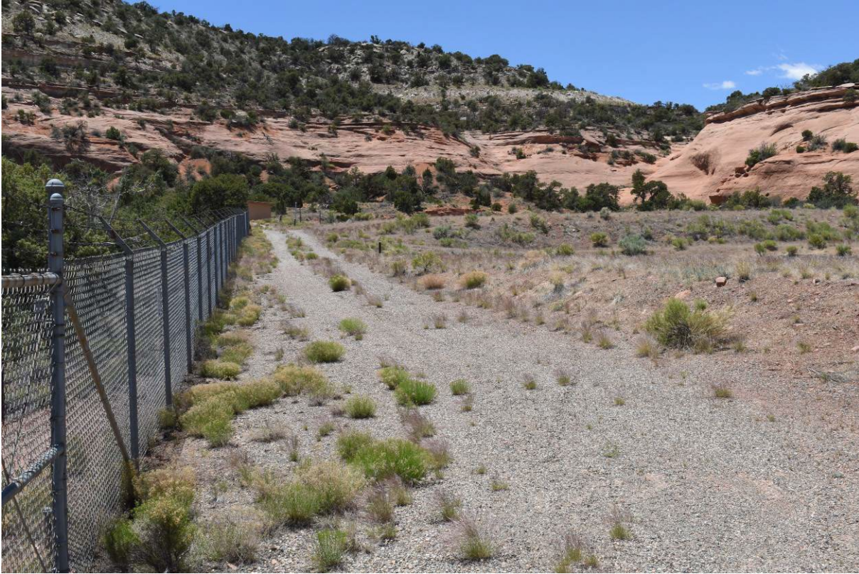
9_1. South Pumphouse and South Wastewater Lagoon, view southwest, June 4, 2024.
