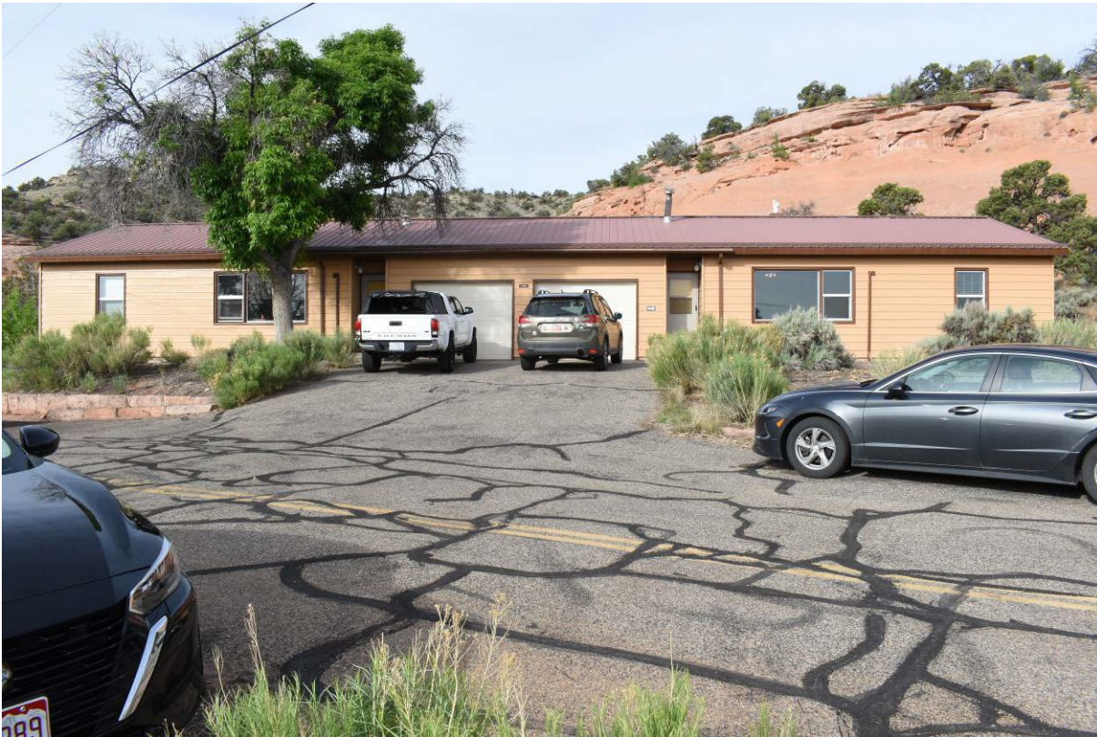
Photo 7. Building #51, view southwest.
