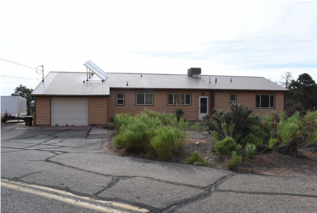
Photo 5. Residence #40, view east.
