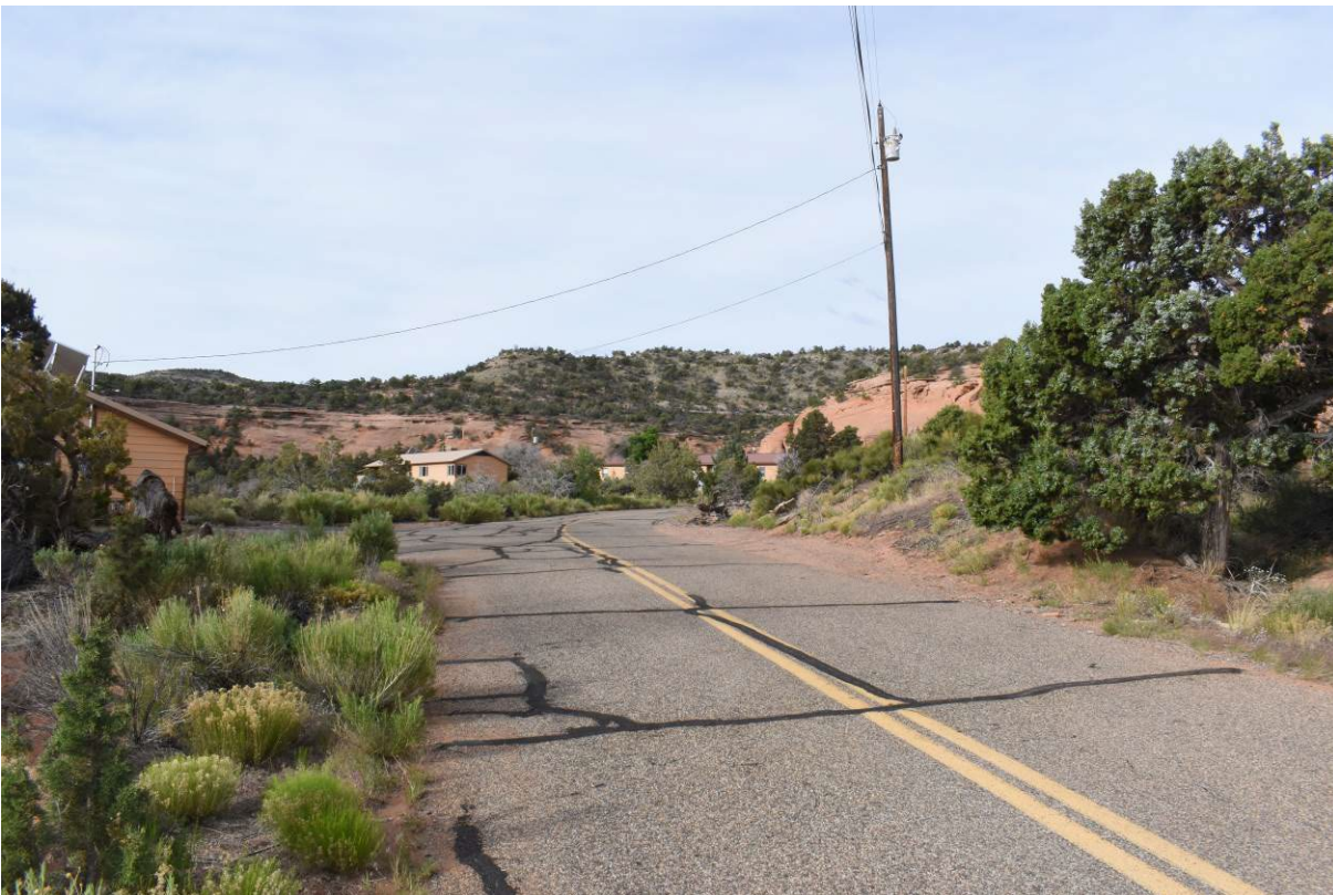
Photo 2. Saddlehorn Maintenance/Residence Road, view southwest. Visible from left to right: Residence #40, Residence #42, and Building #51.
