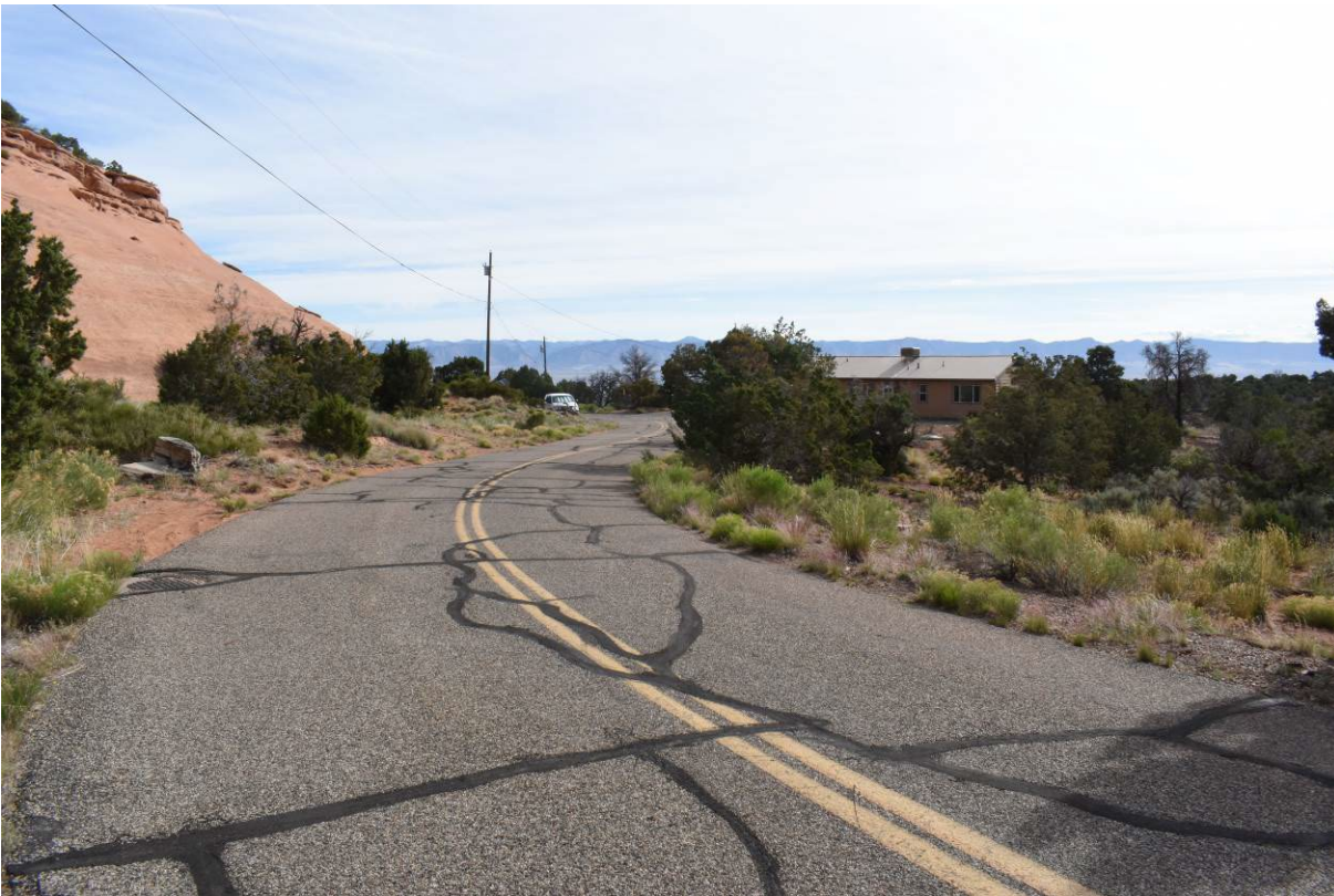
Photo 3. Saddlehorn Maintenance/Residence Road, view northeast toward Residence #40.
