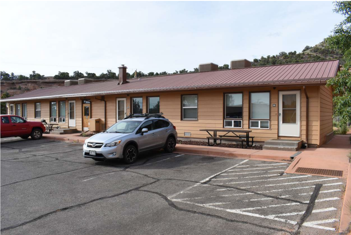
Photo 8. Building #43, view southeast.
