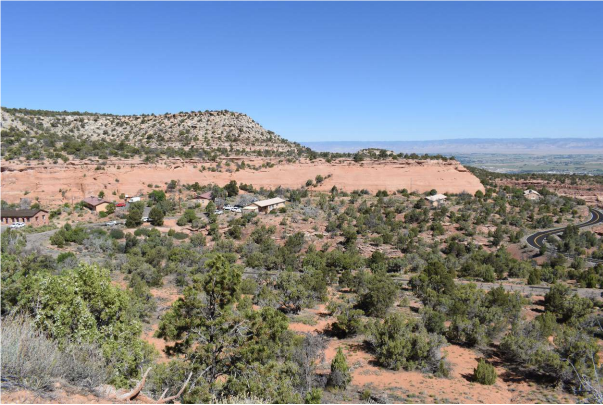
Photo 1. Saddlehorn Mission 66 Residential Area, view north from Water Tank Road/Black Ridge Trail with Saddlehorn Maintenance/Residence Road near foreground. Visible from left to right: Saddlehorn Utility Area Historic District, Building #51, Building #43, Residence #42, Residence #40, Residence #37, and Rim Rock Drive.
