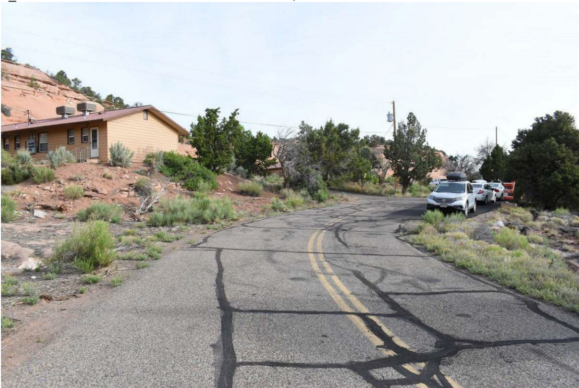
1_2. Saddlehorn Maintenance/Residence Road, view north from south end of road just north of Saddlehorn Utility Area.
