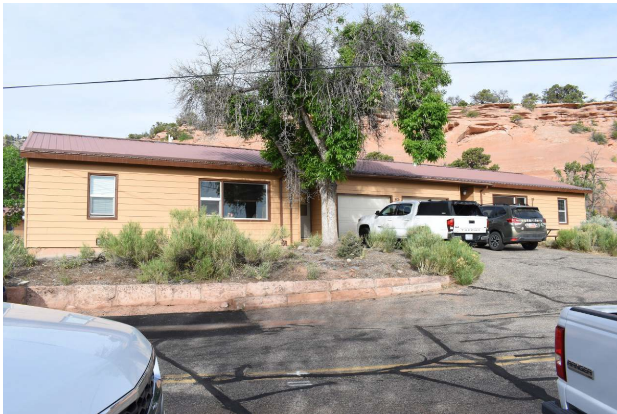
5ME21287_1. Northeast elevation, view west.
