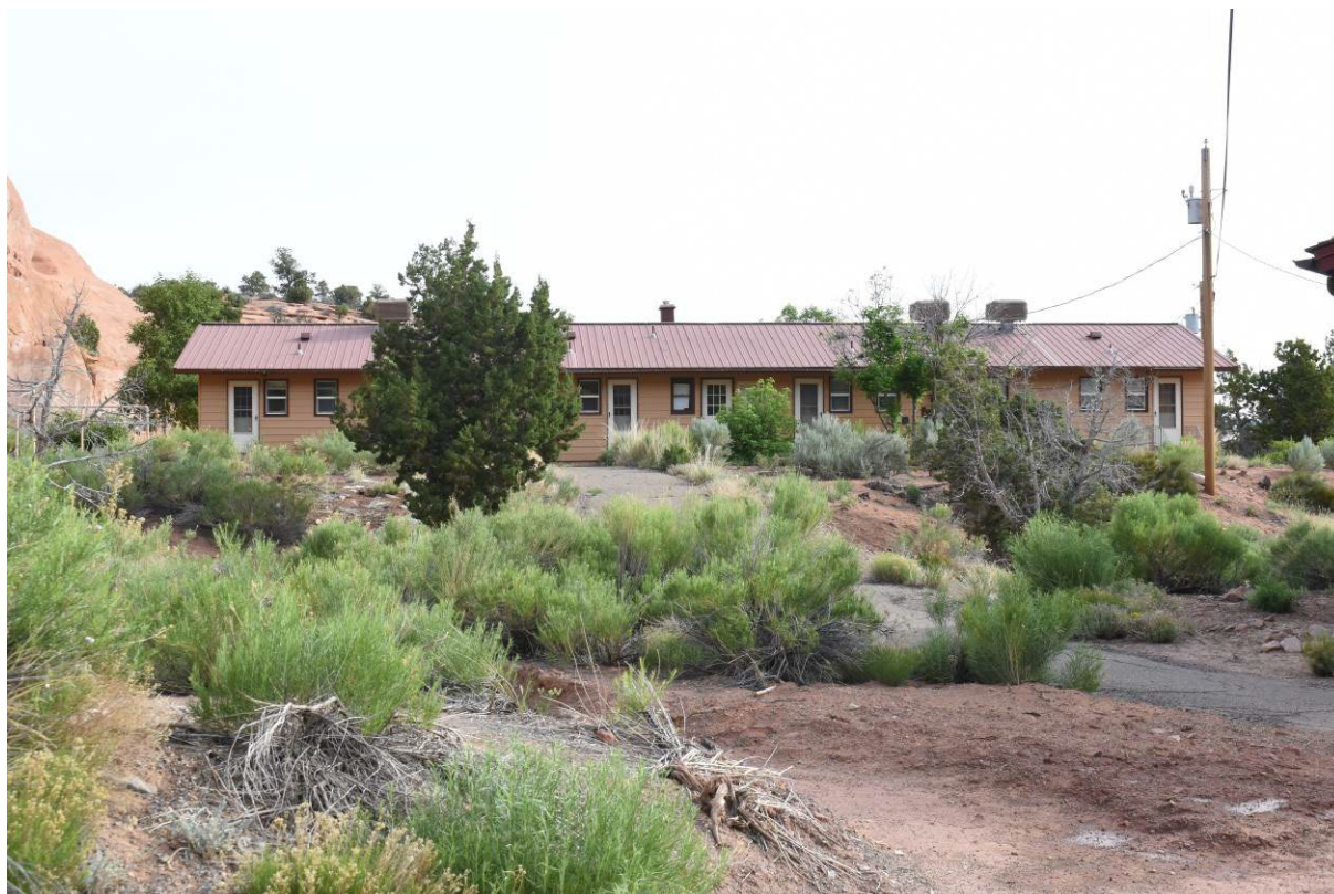
5ME21288_2. South elevation, view north.
