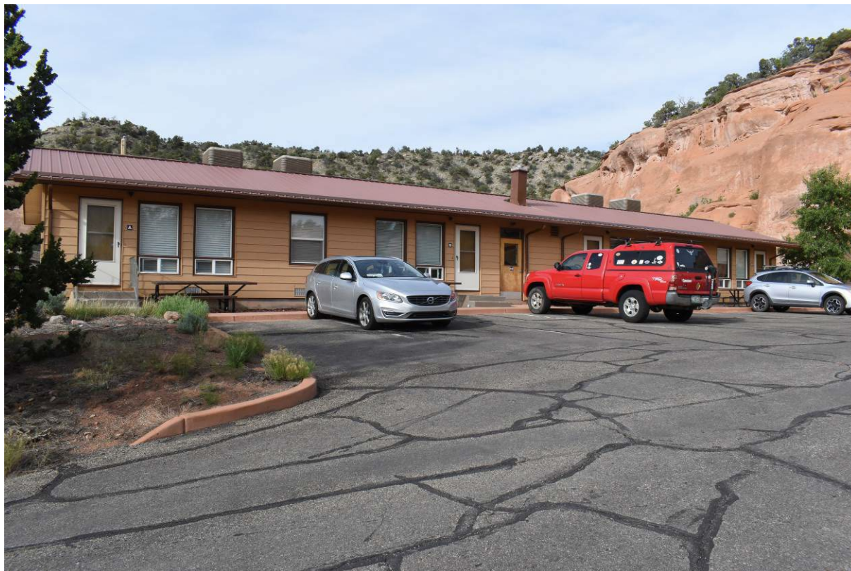
5ME21288_1. North elevation, view southwest.
