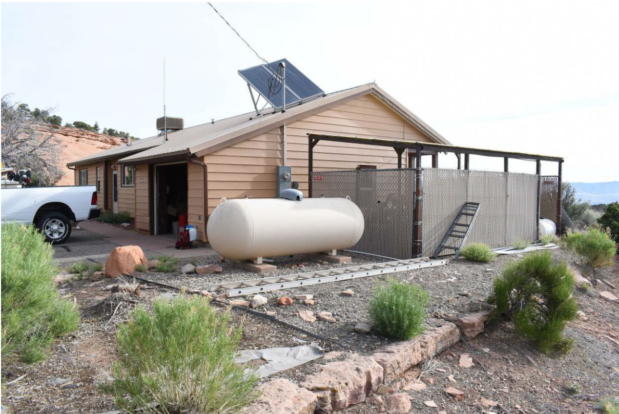
5ME21286_2. West and south elevations, view northeast.
