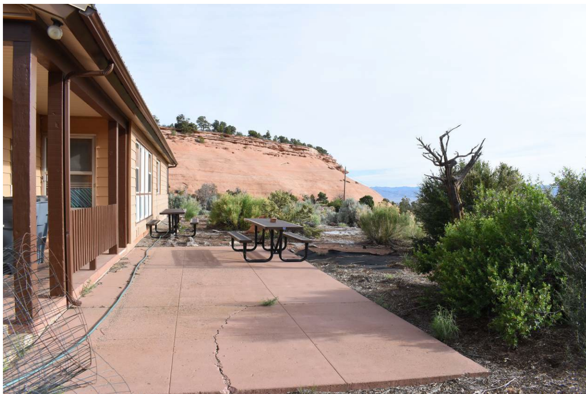
5ME21286_3. East elevation, view north.
