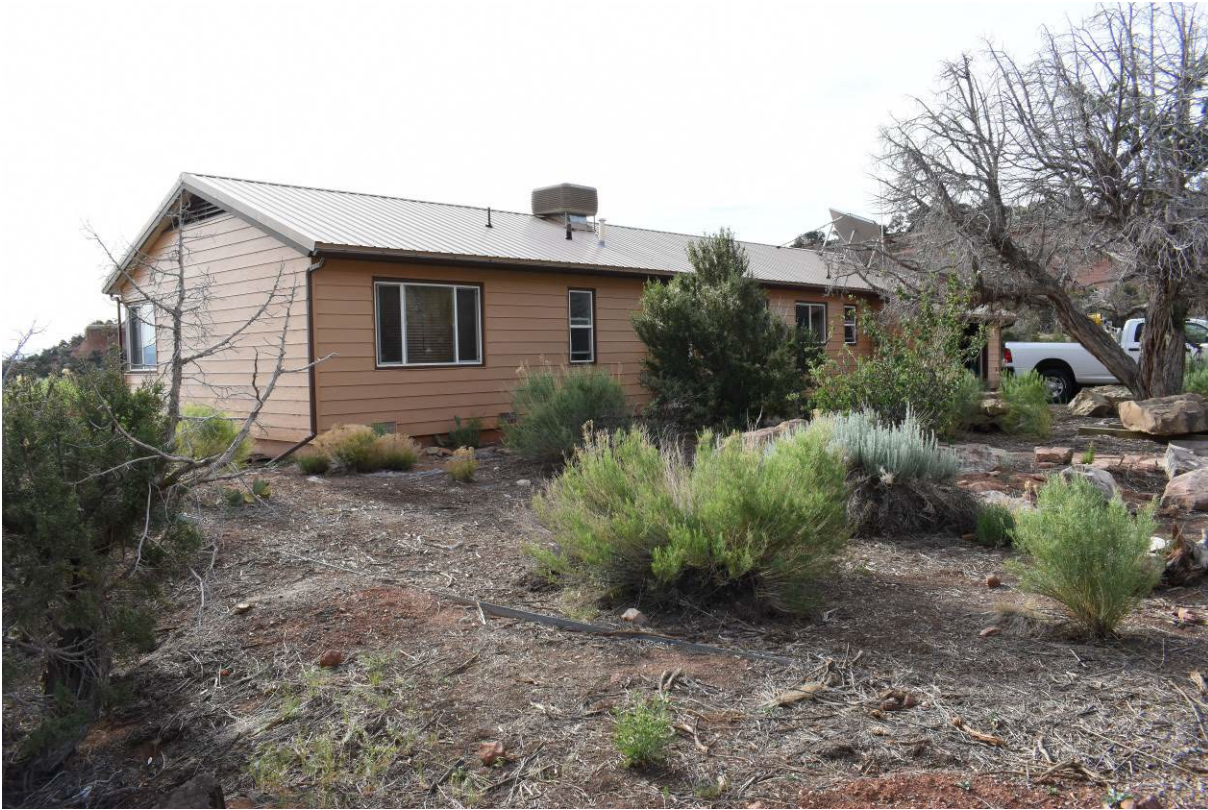
5ME21286_1. North and west elevations, view southeast.
