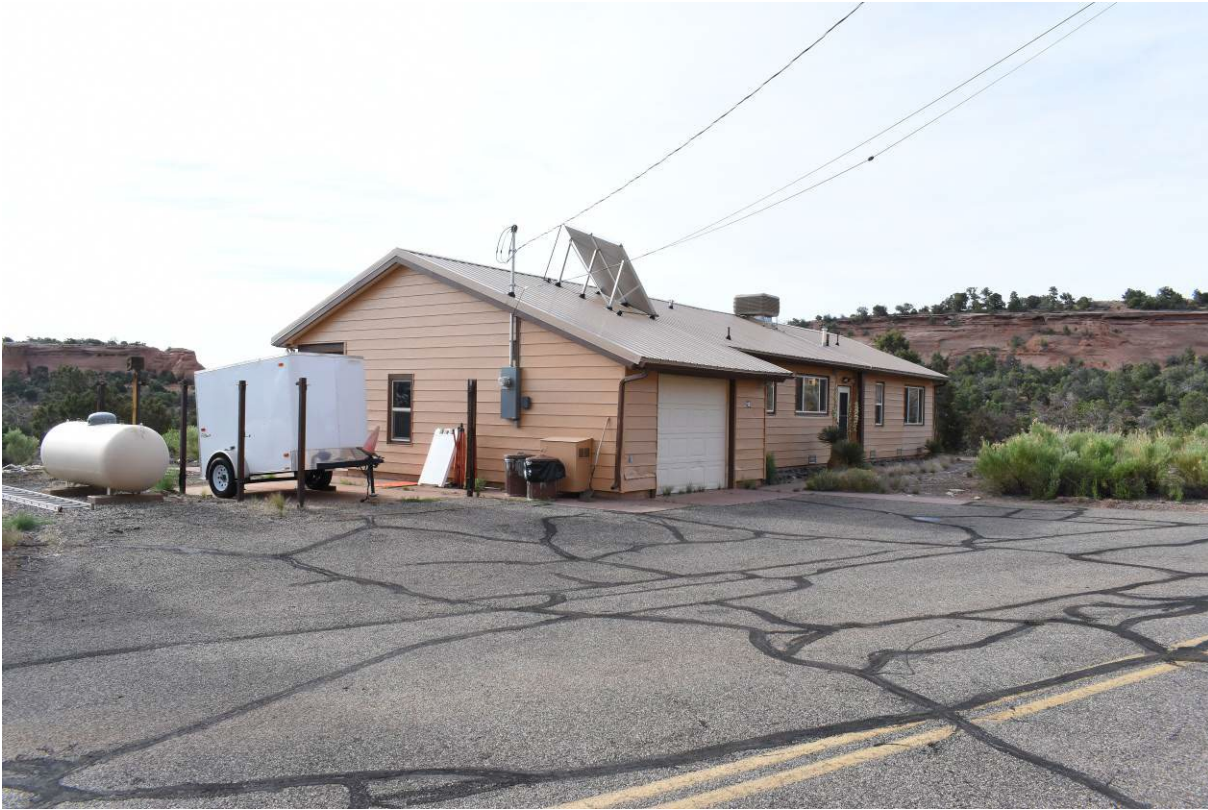
5ME21285_1. North and west elevations, view southeast.
