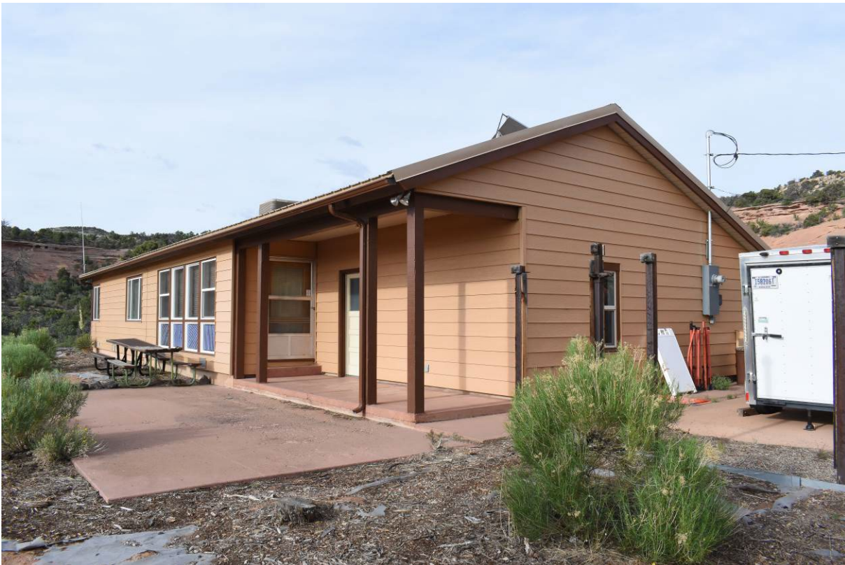
5ME21285_2. East and north elevations, view southwest.
