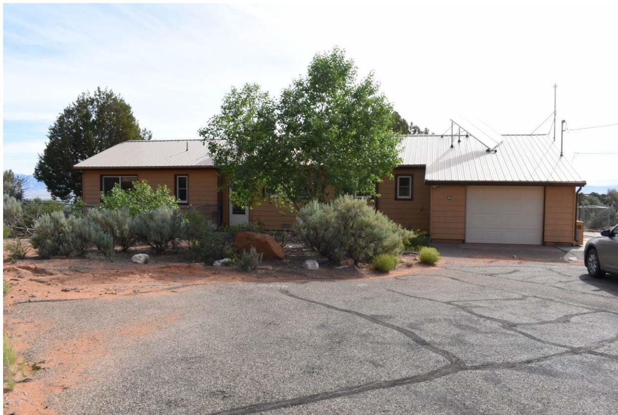
5ME21284_1. West elevation, view northeast.
