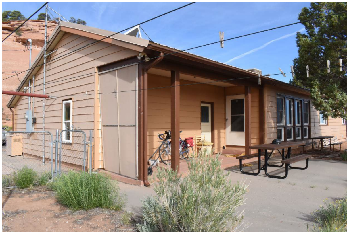
5ME21284_2. South and east elevations, view northwest.
