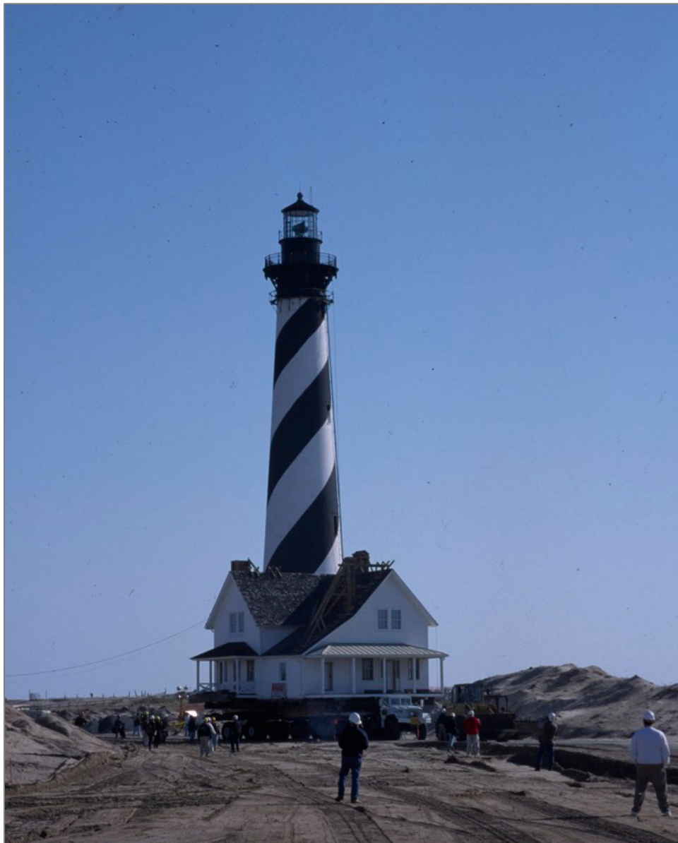
Relocating the Cape Hatteras Lighthouse Principal Keeper's Quarters at Cape Hatteras National Seashore, March 23, 1999.
