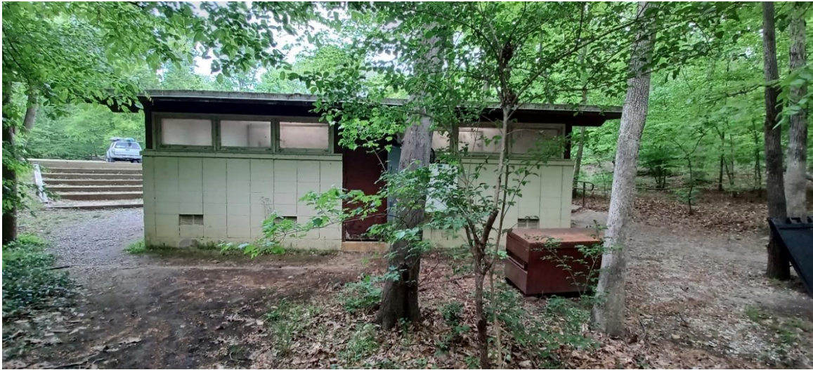
West Comfort Station - West Elevation.
