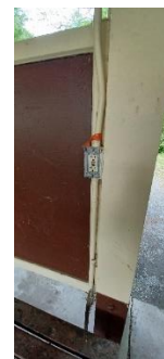
Carderock Pavilion - wood trim around north wooden panel.
