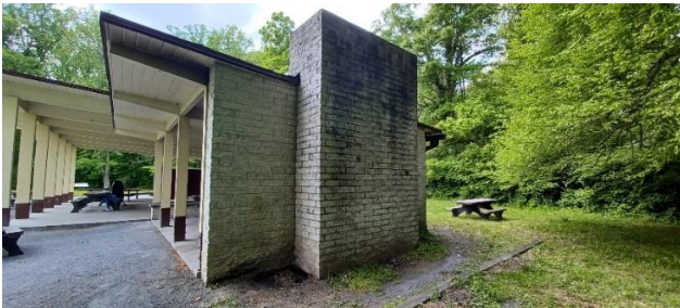
Pavilion – southeast brick wall.
