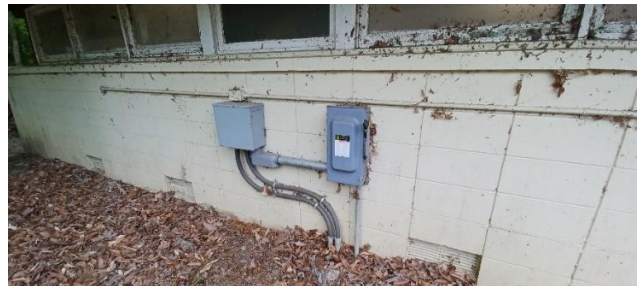
West Comfort Station – east wall.
