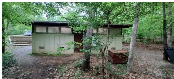
West Comfort Station – west elevation.
