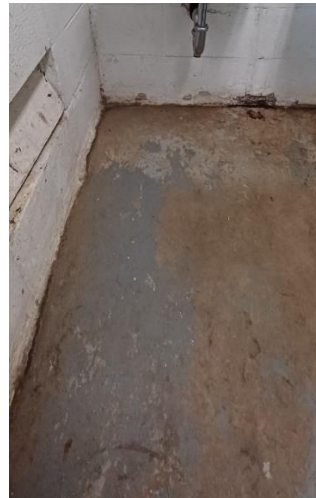
West Comfort Station (Women's Room) slab on grade.
