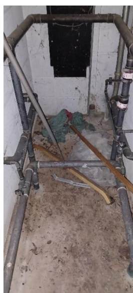
East Comfort Station, Closet showing plumbing and waste pipes.
