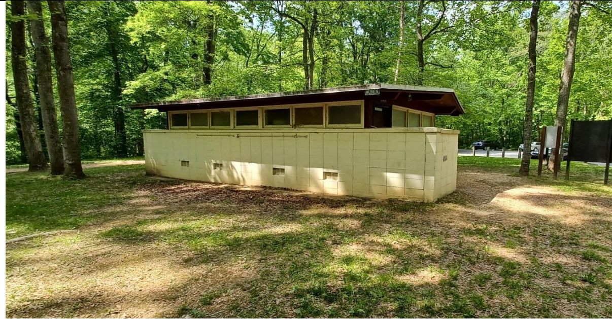
East Comfort Station – Southwest Oblique.
