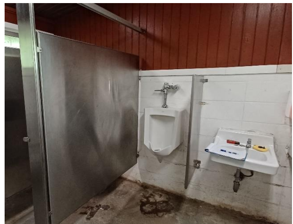
West Comfort Station men's room.
