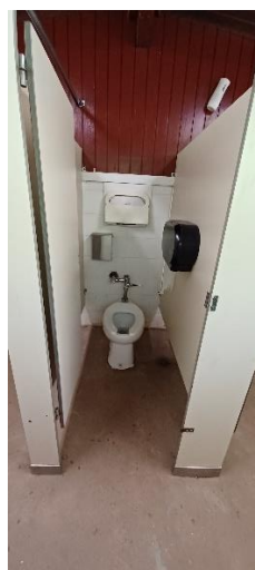
East Comfort Station, Women's Room.
