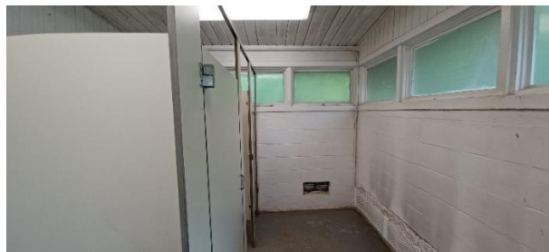
West Comfort Station – women's room.
