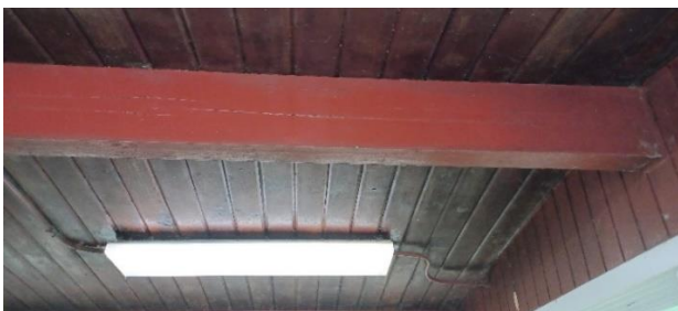
East Comfort Station, men’s room ceiling stain & paint in good condition.
