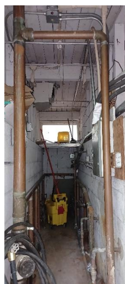
West Comfort Station, Closet showing plumbing and waste pipes.
