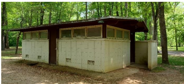
East Comfort Station – southwest oblique.
