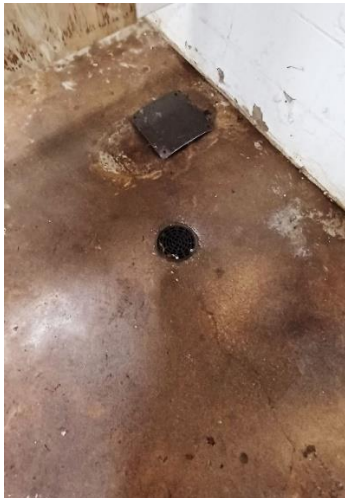
East Comfort Station (Men's room) foundation slab on grade.
