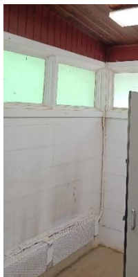
East Comfort Station, Men's Room wall.
