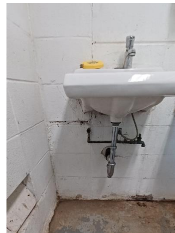
West Comfort Station, Women's Room.
