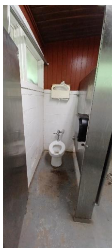
West Comfort Station, Men's Room.
