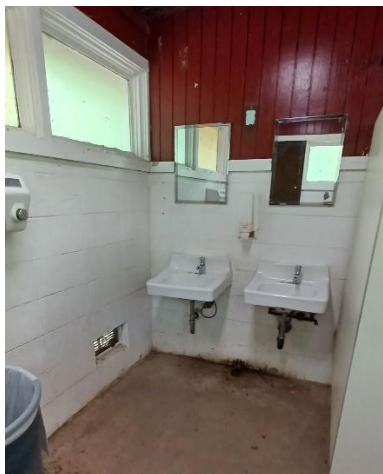
East Comfort Station, Women's Room.
