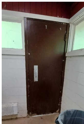
East Comfort Station, Women's Room Door Interior.
