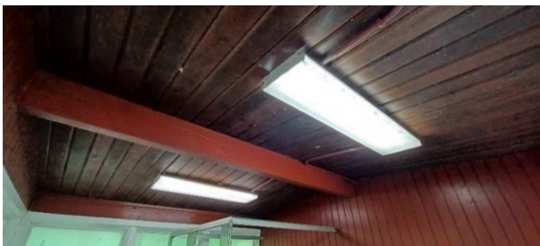
West Comfort Station, men’s room, ceiling stain & paint in good condition.
