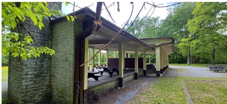
Carderock Pavilion gutters and downspouts on northeast corner.
