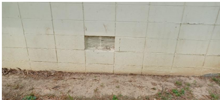
East Comfort Station – west wall.
