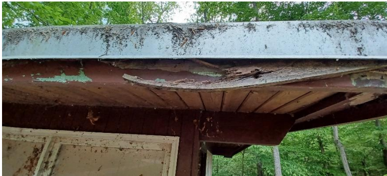
West Comfort station wood soffit deterioration.
