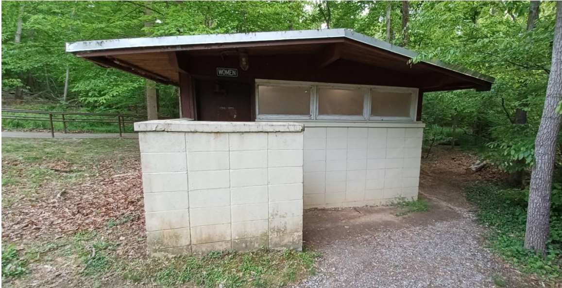
West Comfort Station - North Elevation.
