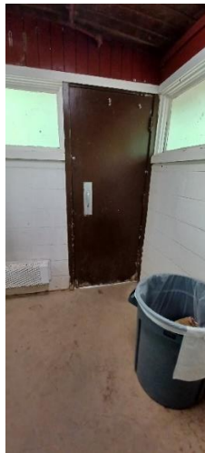
East Comfort Station (Women's Room) slab on grade.
