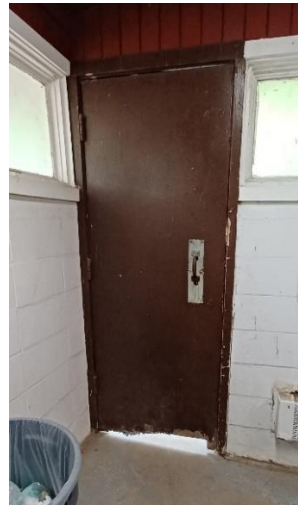
West Comfort Station, Men's Room Door, Interior.
