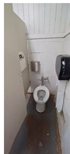
West Comfort Station, Women's Room.
