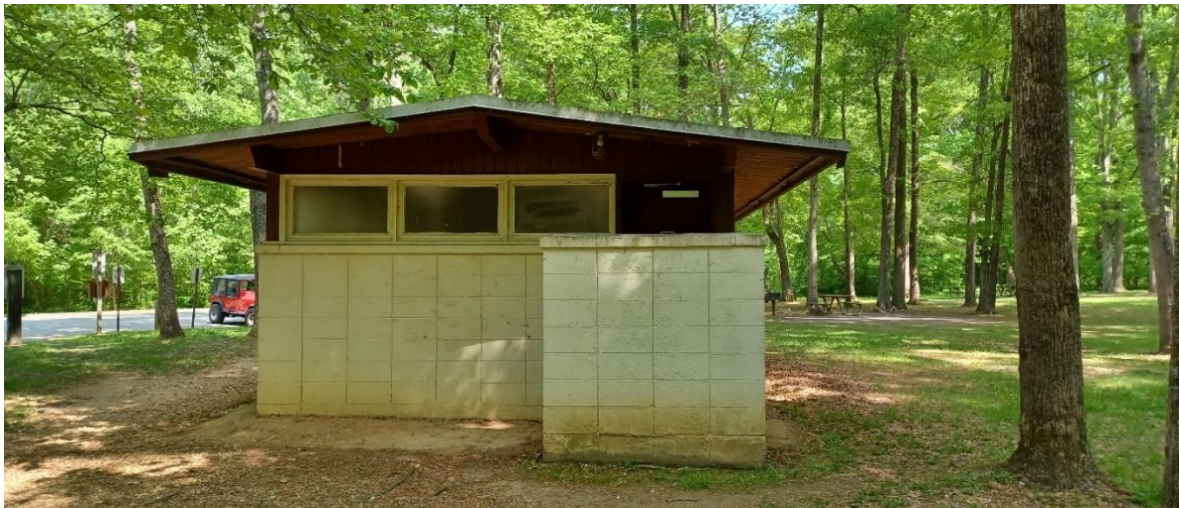
East Comfort Station – North Elevation.
