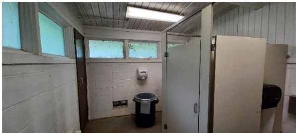
West Comfort Station – Women's room dividing walls.
