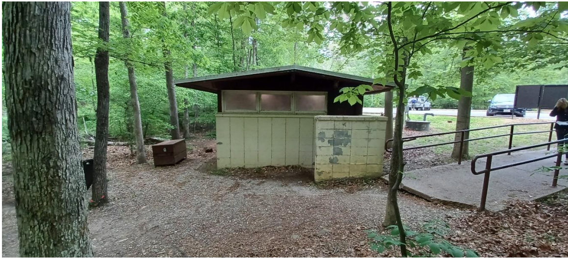
West Comfort Station – South Elevation.
