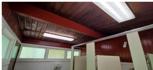
East Comfort Station, women’s room, ceiling stain and paint in good condition.
