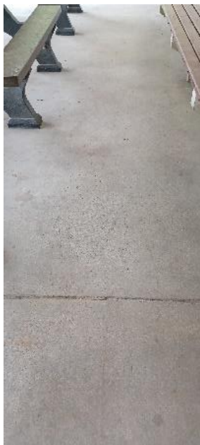
Pavilion slab foundation/floor.
