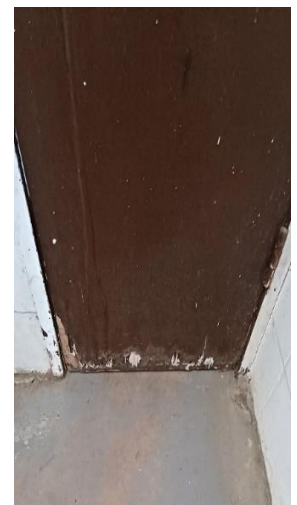
West Comfort Station, Women's Room Door, interior.
