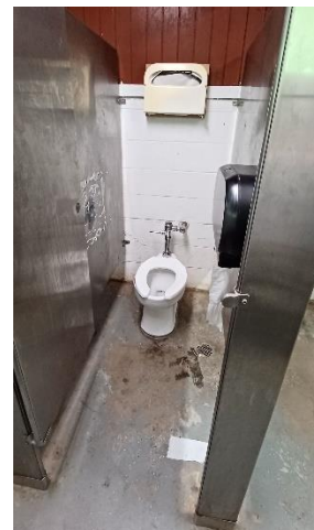
West Comfort Station, men's room stall walls.
