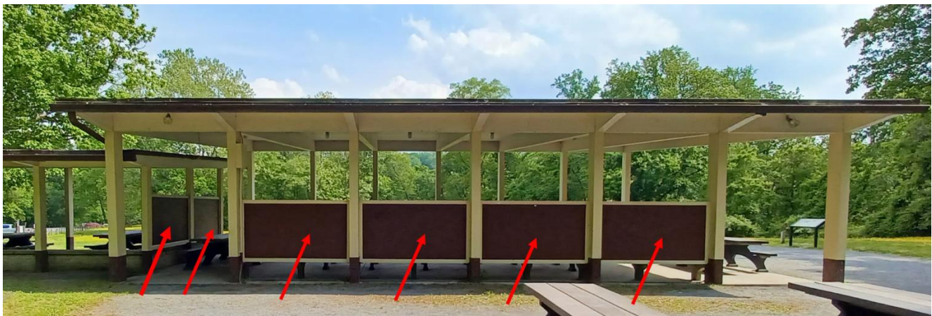
Carderock Pavilion, wood screening on north and east walls.
