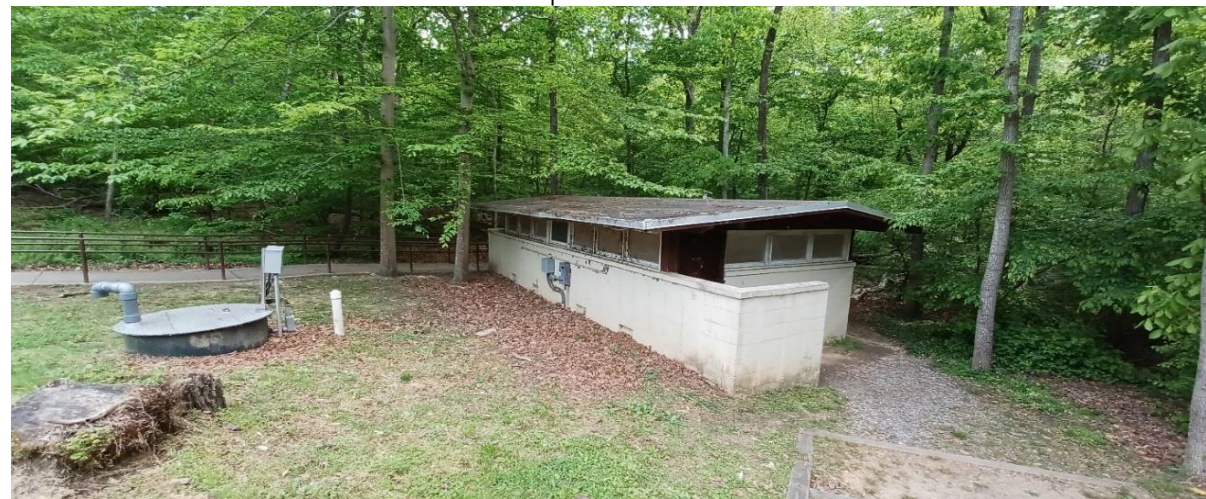
West Comfort Station – Northeast Oblique.
