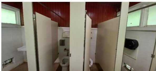
East Comfort Station – Women's room dividing walls.
