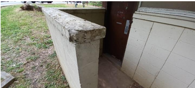
West Comfort Station – Privacy wall at Women's Room.
