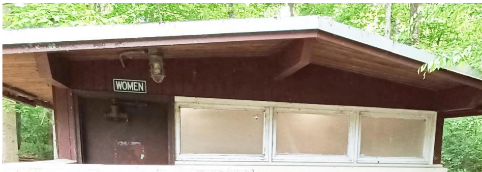
West Comfort Station – North elevation.
