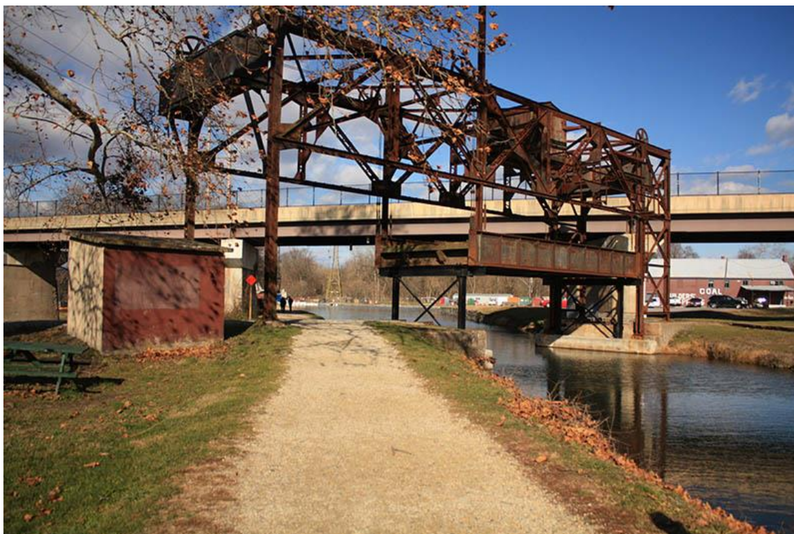
Railroad Lift Bridge (NCR CLP 2018).
