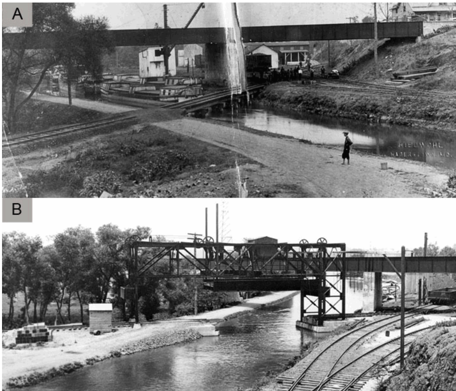
A: 1922. Temporary track over canal (CHOH Historic Photo Collection)
