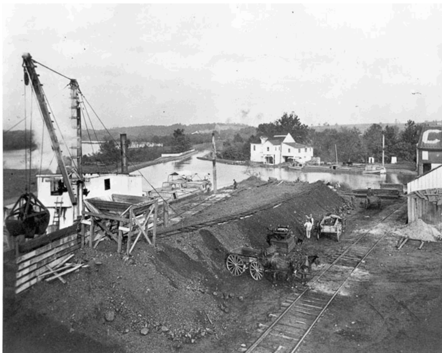
c.1900's. View of Williamsport Basin and wharf on an average work day. (CHOH Historic Photo Collection)
