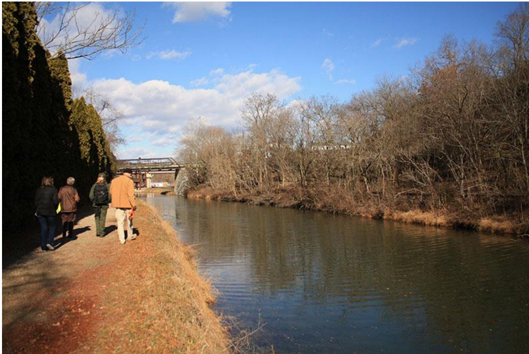
The condition of the vegetation lining the canal prism (NCR CLP 2018).
