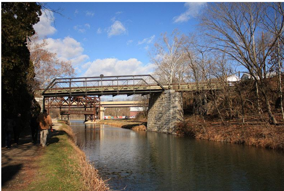
Bollard Bridge (NCR CLP 2018).
