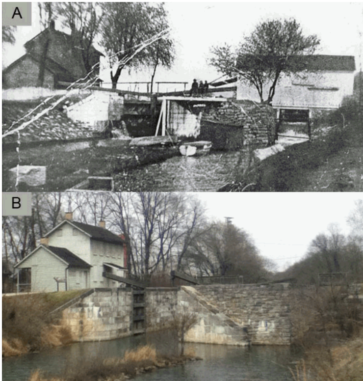
A: c.1919. Upstream view of Lock 44, bypass flume, lockhouse, and the carpenter's shop (CHOH Historic Photo Collection)
