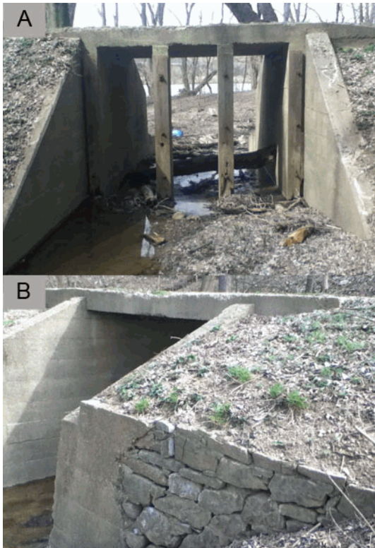
A: 2012. View of wastew weir (mile 98.90) looking toward Potomac River (NPS/NCR)
