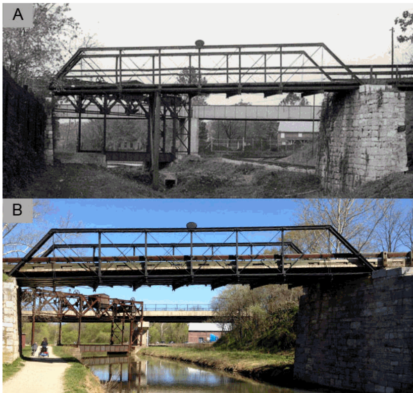
A: Post 1924. View of Bollman Bridge from towpath looking upstream (CHOH Historic Photo Collection)
