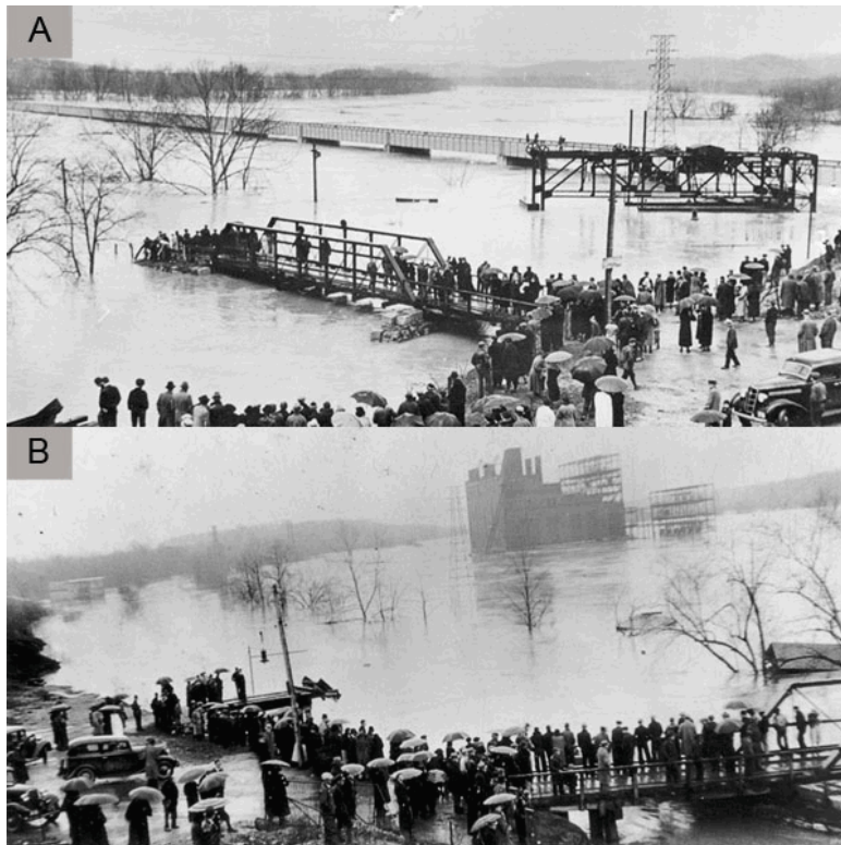
A: 1936. Foreground: Bollman Bridge; Right-Center: Lift Bridge; Background: Washington-Berkeley Bridge (CHOH Historic Photo Collection) B: 1936. Bottom-Right: Bollman Bridge; Background: Potomac Edison's industrial building (CHOH Historic Photo Collection)
