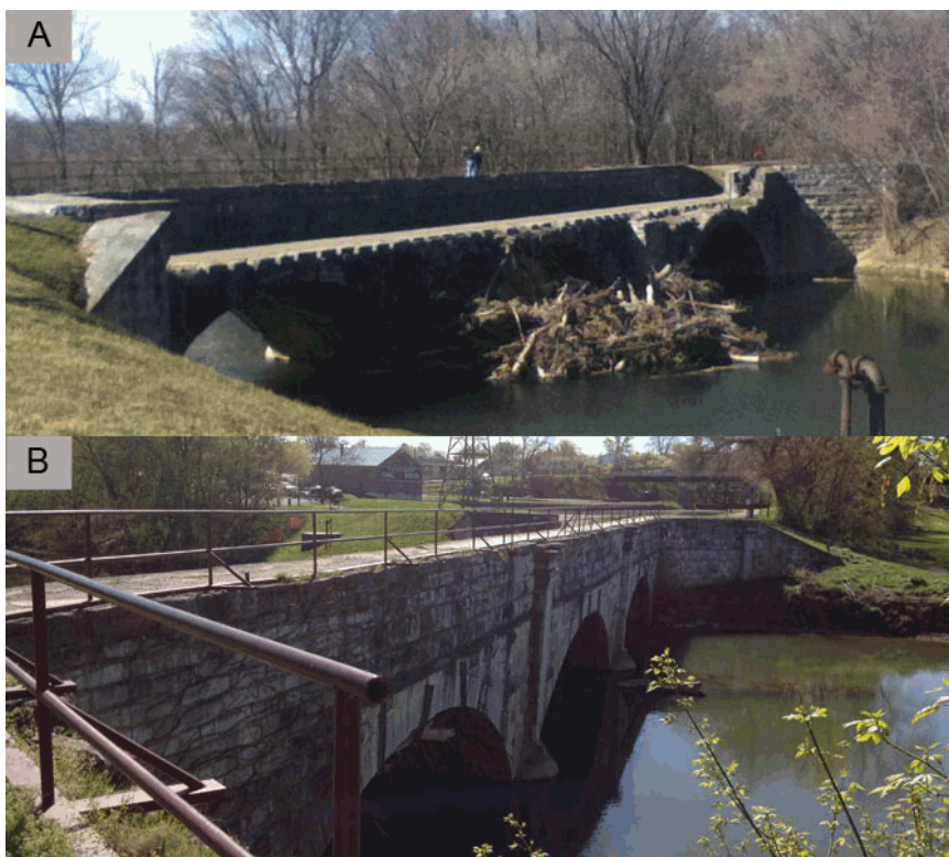
A: 2012. Berm side of aqueduct looking upstream (NPS/NCR)
