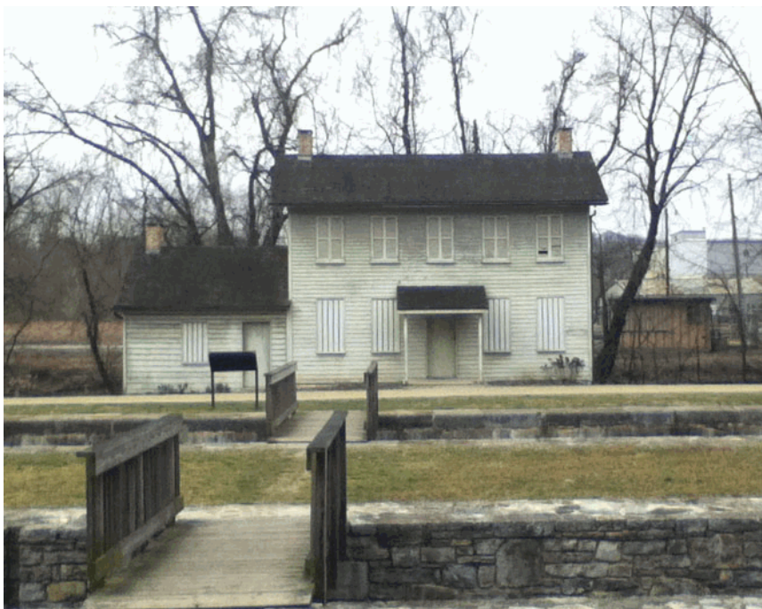
2012. Lockkeeper's house at Lock 44. View of front façade from berm side. Note bypass flume in foreground and lock in the center (NPS/NCR)
