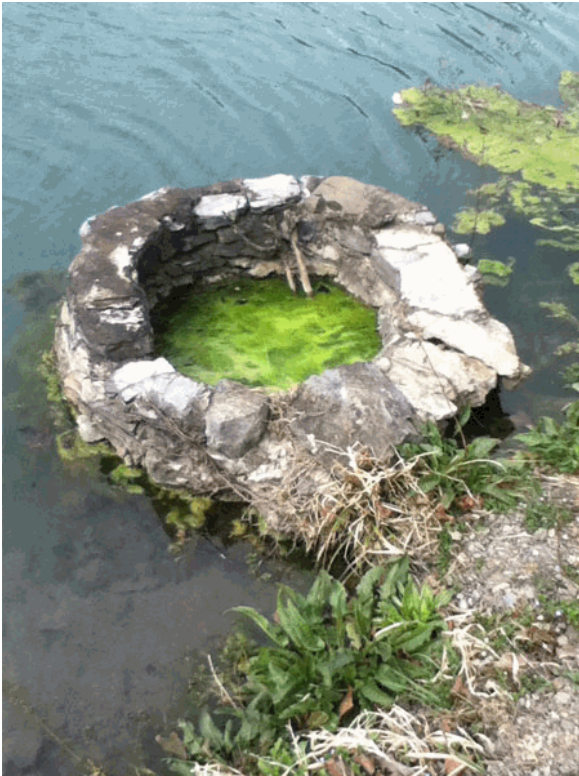
2012. Compatible stone feature downstream of Lock 44 on berm side (NPS/NCR)
