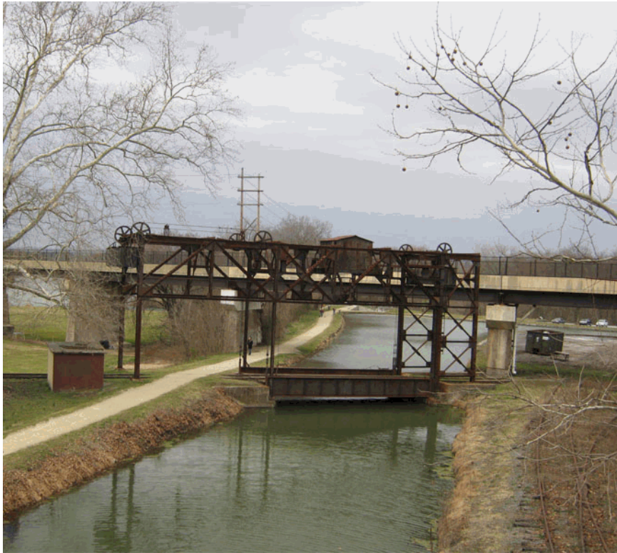
2012. Railroad lift bridge in its closed/lowered position. View looking upstream from Bollman Bridge (NPS/NCR)
