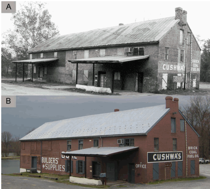
A: Post 1924. Cushwa Warehouse from Potomac Street looking toward canal (CHOH Historic Photo Collection)
