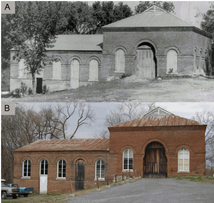
A: Post 1924. View of power generating station from Potomac Street looking upstream (CHOH Historic Photo Collection)
