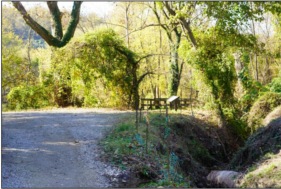
Figure 3-33. View 3 emerging from the culvert, enclosed by vegetation (Quinn Evans, 2021).
