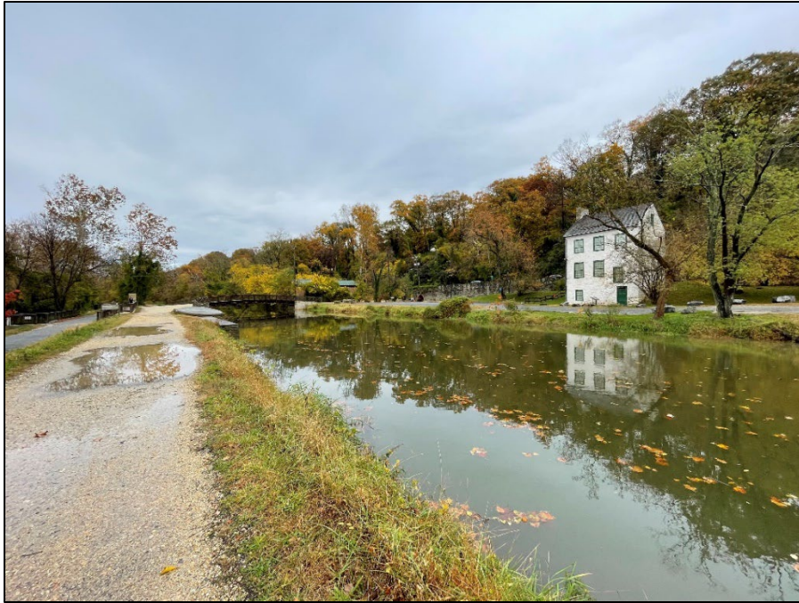
Figure 3-8. The C&O Canal, Towpath Trail, and Abner Cloud House facing north (Quinn Evans, 2021).
