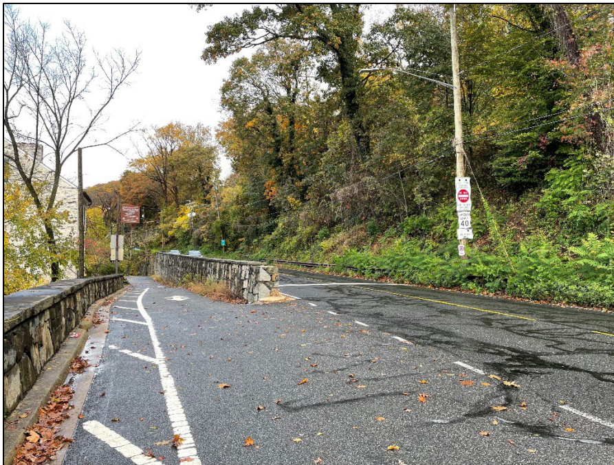
Figure 3-23. Site access at the intersection of Canal Road NW and Fletcher's Road (Quinn Evans, 2021).
