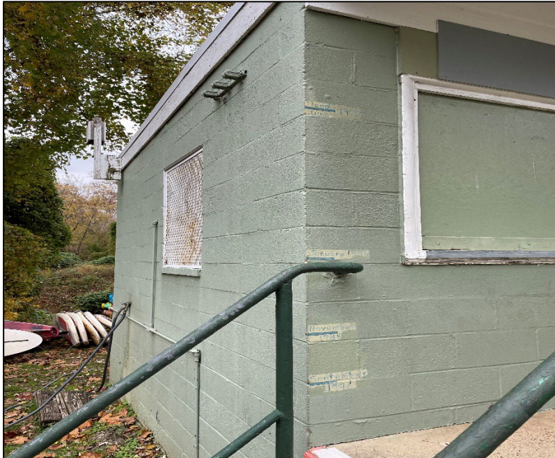
Figure 3-58. Historic flood lines marked on the southwest corner of the refreshment stand (Quinn Evans, 2021).
