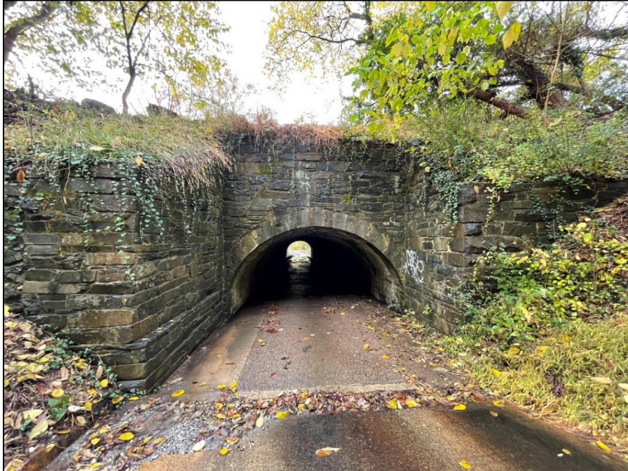
Figure 3-32. View 2 approaching the Fletcher's Road Culvert (Quinn Evans, 2021).
