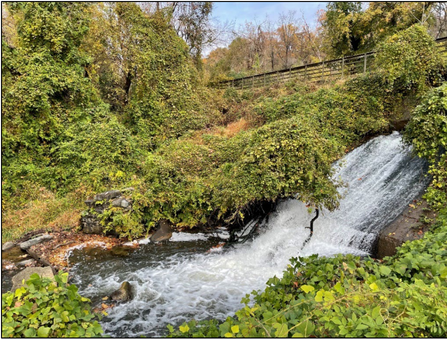
Figure 3-12. Wasteweir 3 conveying water from C&O Canal (Quinn Evans, 2021).
