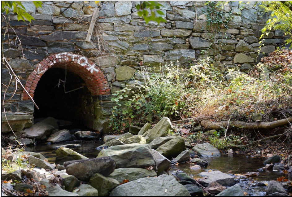
Figure 3-19. Historic Culvert 159-C conveys water under Canal Road NW across from Mile Marker 3 (Quinn Evans, 2021).
