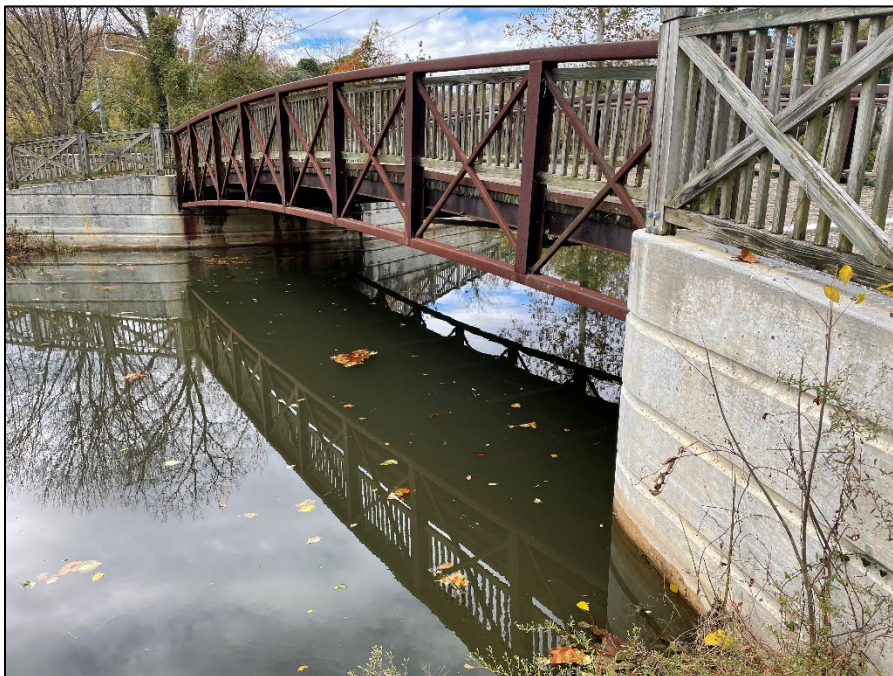
Figure 3-55. The pedestrian bridge spanning the C&O Canal (Quinn Evans, 2021).
