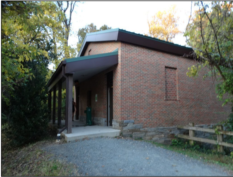
Figure 3-52. The south and west facades of the comfort station/odor control facility with porch and restroom access (Quinn Evans, 2021).
