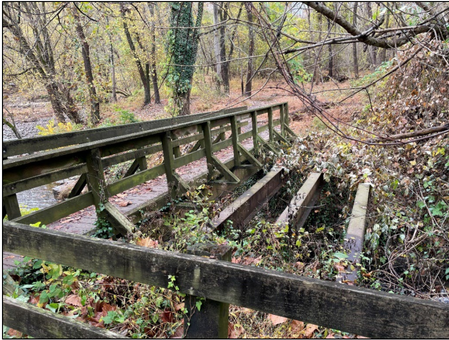
Figure 3-48. A wooden pedestrian bridge provides access to the North Woods and is constructed on repurposed steel I-beams (Quinn Evans, 2021).
