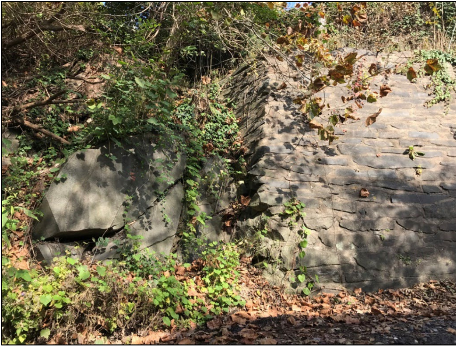
Figure 3-4. Exposed bedrock meets the Canal Road retaining wall on Fletcher's Road (Quinn Evans, 2021).
