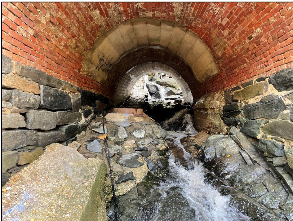
Figure 3-18. The Maddox Branch Culvert under Canal Road NW, Potomac Interceptor lateral line access manhole in the foreground (Quinn Evans, 2021).
