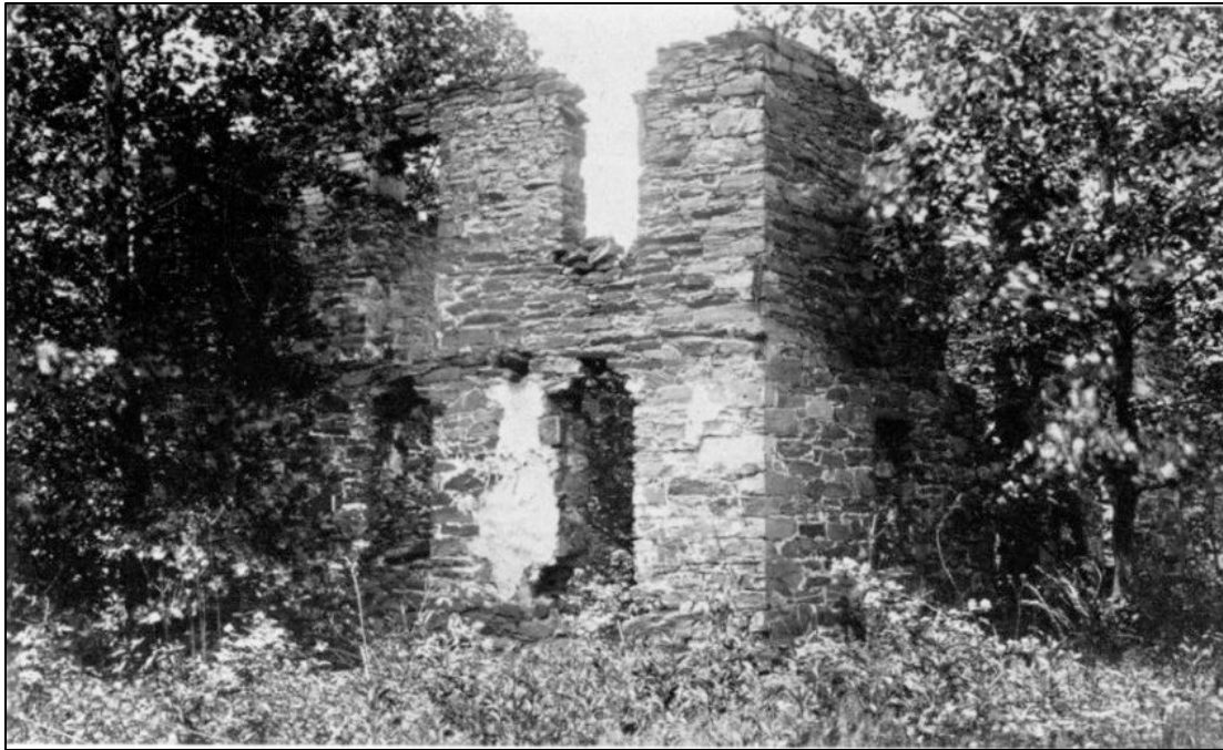
Figure 2-16. Photograph of ruinous structure mistakenly labeled the "Cloud-Edes Mill," 1930 (Allen C. Clark, "The Old Mills," Records of the Columbia Historical Society, Washington, DC).
