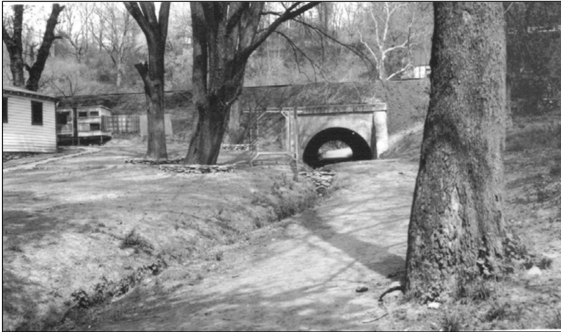
Figure 2-20. Photograph of area near mill site showing house at left, 1939 (Thomas C. Vint, Outline Report of Architectural Work on the Restoration of the Chesapeake and Ohio Canal for Recreational Use (Georgetown, DC, to Seneca, MD) (National Park Service, 1939), 15.
