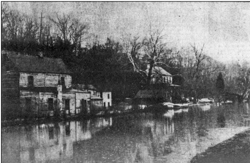
Figure 2-25. Photograph showing some of the homes along the canal demolished in 1958. Near the middle of the photograph is the Abner Cloud House, which was spared from demolition (Evening Star, March 6, 1958). Reprinted with permission of the DC Public Library, Star Collection © Washington Post.
