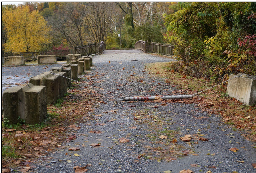
Figure 3-64. Concrete bin blocks separating vehicular and pedestrian areas in the Canal Corridor (Quinn Evans, 2021).
