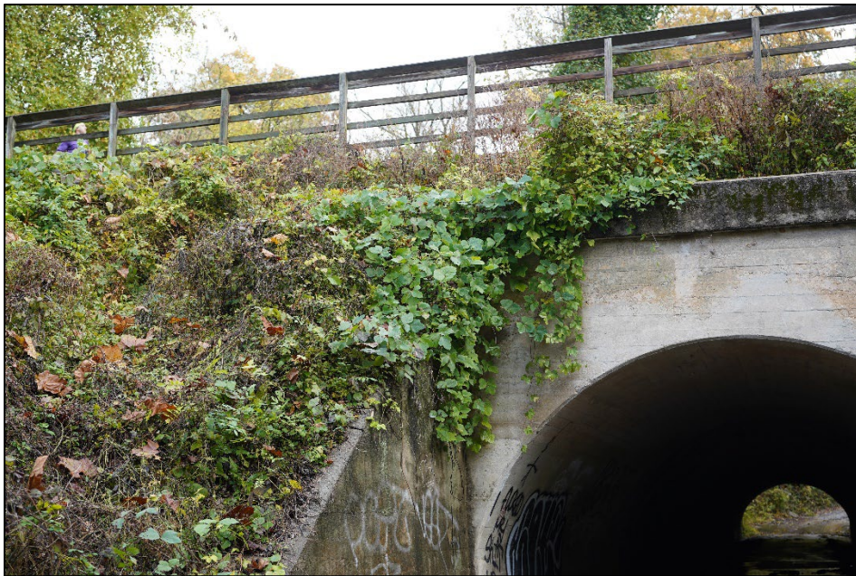
Figure 3-17. Board-formed concrete extension of the Fletcher's Road culvert (Quinn Evans, 2021).
