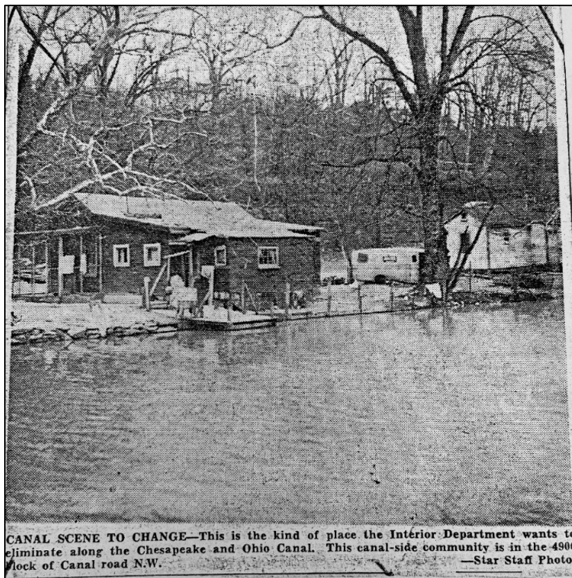
Figure 2-26. Photograph showing some of the homes along the canal demolished in 1958 (Evening Star, 1953). Reprinted with permission of the DC Public Library, Star Collection © Washington Post.
