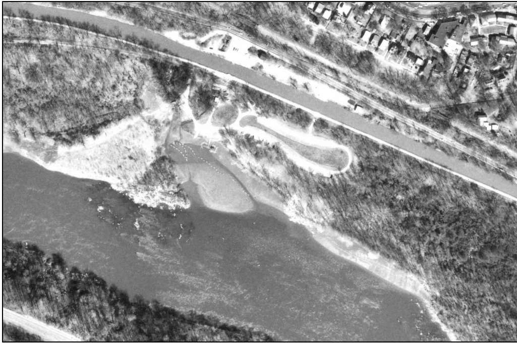
Figure 2-30. Aerial photograph showing new parking area, 1971 (National Park Service).
