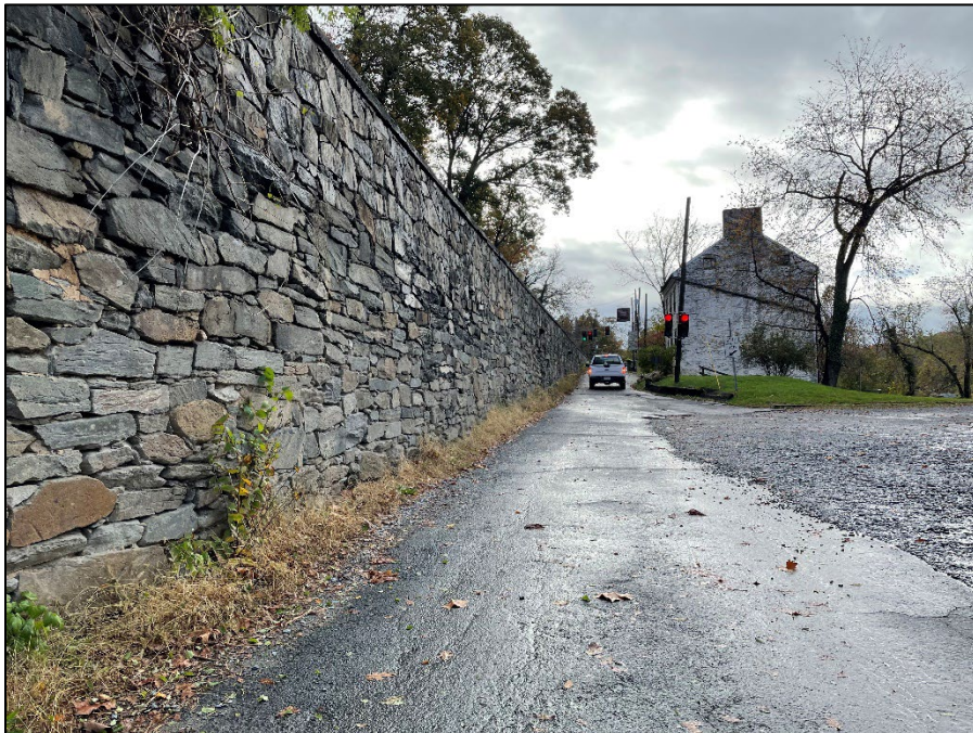
Figure 3-53. The stone retaining wall negotiates the change in grade between Canal Road and Fletcher's Road (Quinn Evans, 2021).
