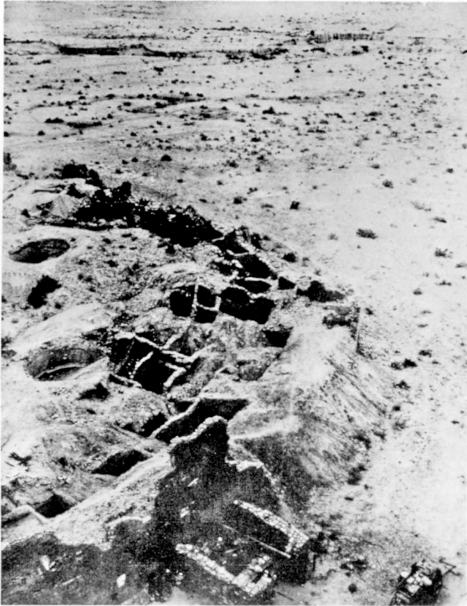
West end of Pueblo Bonito during excavation by Wetherill and Pepper in the 1890's
