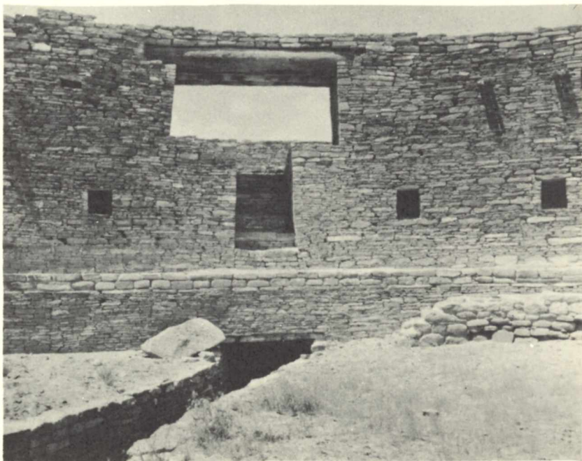
Casa Rinconada, north entrance and subterranean passageway leading to antechamber room.
