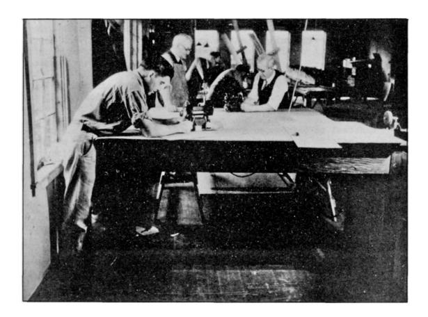
Using a Cutawl to Shape Cardboard Sheets for a Relief Model.
