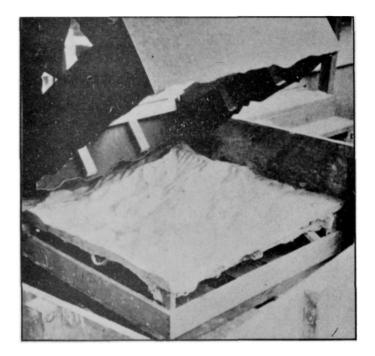
Setting the Frame for the Final Casting. Note construction of frames for casting and mold.
