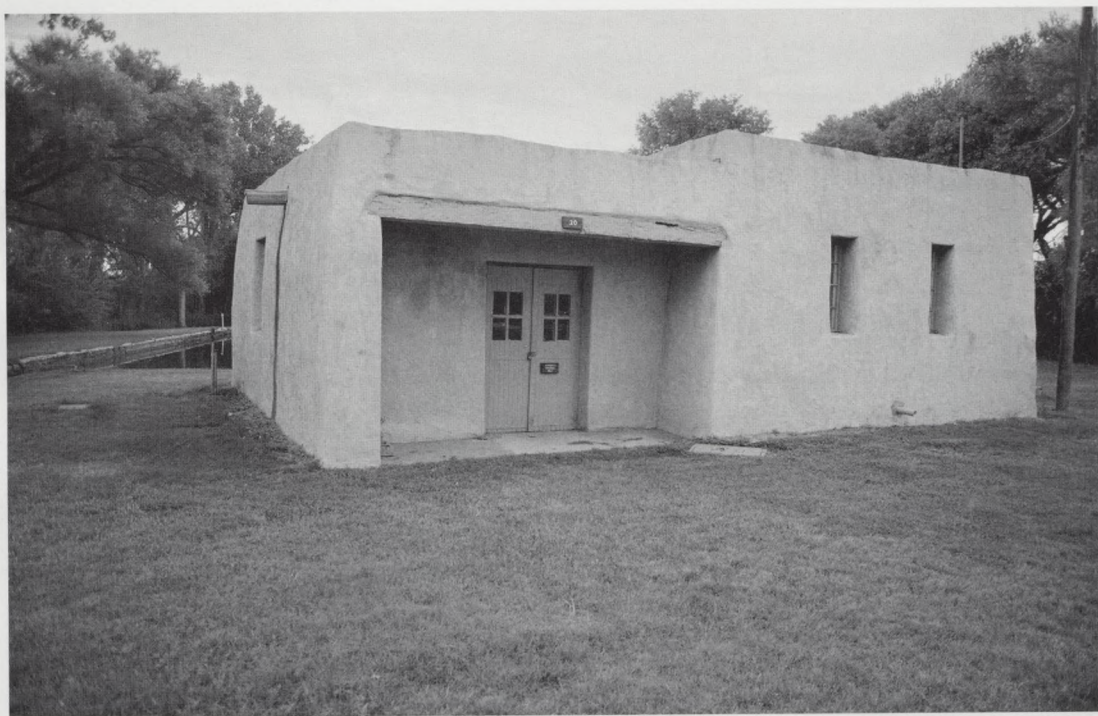
Fig. 26. Pump house next to Rattlesnake Spring. During summer months, fecal droppings from night-roosting bats can be observed on the floor and walls of the front porch (photograph taken 4 August 1996).
