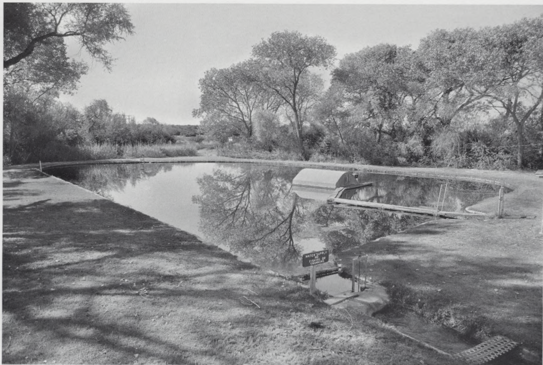
Fig. 24. This rock-lined storage pond is named Rattlesnake Spring. The limestone-block wall surrounding the pond was constructed in 1941. Woodlots are established on both sides of the pond. The west woodlot can be seen in the background on the right side (photograph taken 23 October 1999).
