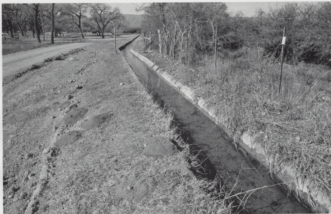
Fig. 25. Cement aqueduct at Rattlesnake Springs. This portion of the aqueduct is near the picnic area. Earthen mounds formed by pocket gophers can be seen in the grass next to the aqueduct. The fence on the right runs along the northern boundary of the park and separates the park from property owned by Washington Ranch. Part of the picnic area and gravel road can be seen in the upper left-hand corner (photograph taken 31 December 1998).
