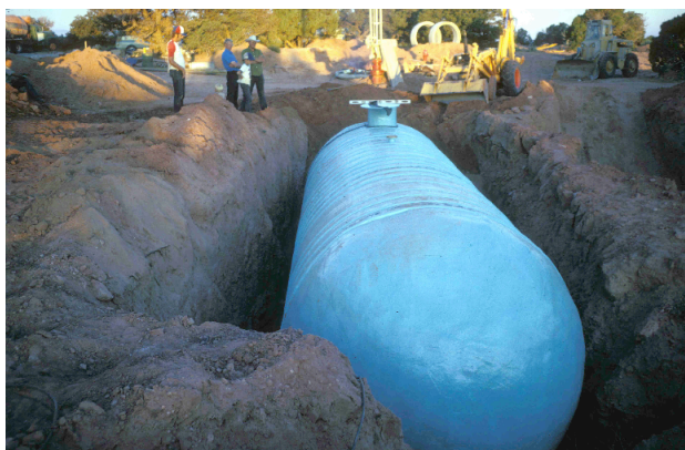
Water tank installation
