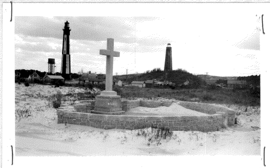
The Cape Henry Memorial Cross, Showing Its Relation to the Old and New Lighthouses at Cape Henry. Note How the Encircling Stone Wall Acts As a Sand Trap.
