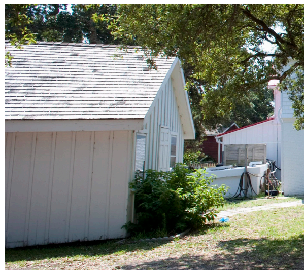
FIGURE 2-146. Storehouse after addition of edging, 2010. (NPS/CAHA Collection)
