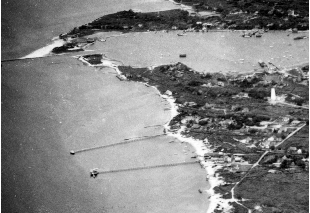
FIGURE 4-4. Aerial showing vegetation around the station, 1936. (NPS/CAHA Collection)
