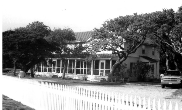
FIGURE 2-85. Double keepers' quarters, 1990. (NPS/CAHA Collection)
