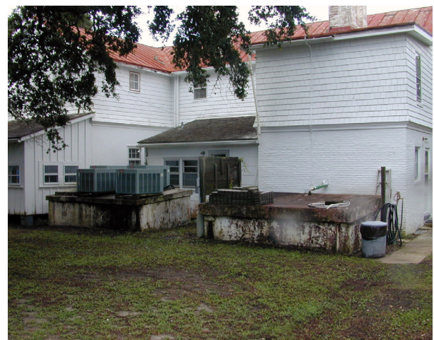
FIGURE 2-95. Cisterns, 2005. (NPS/CAHA Collection)
