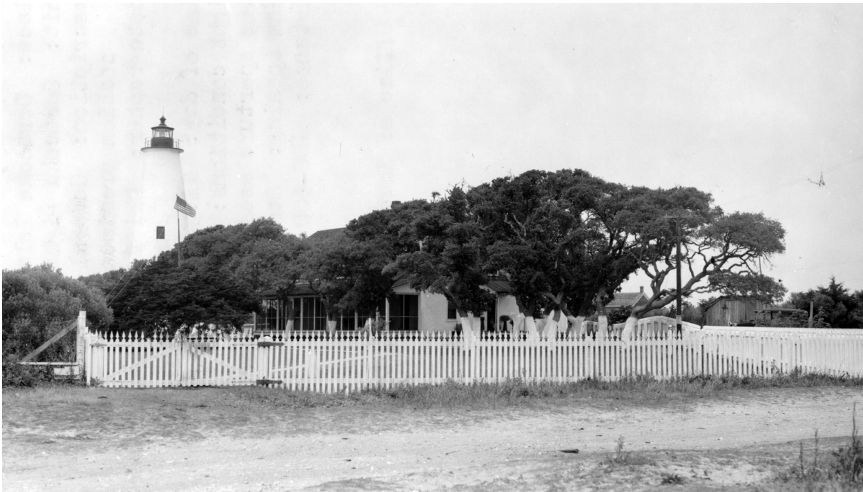
FIGURE 2-117. Gate into the light station with walkway beyond, 1941. (NPS/CAHA Collection)
