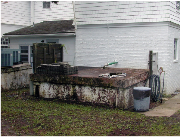
FIGURE 3-28. Cisterns, 2005. (NPS/CAHA Collection)
