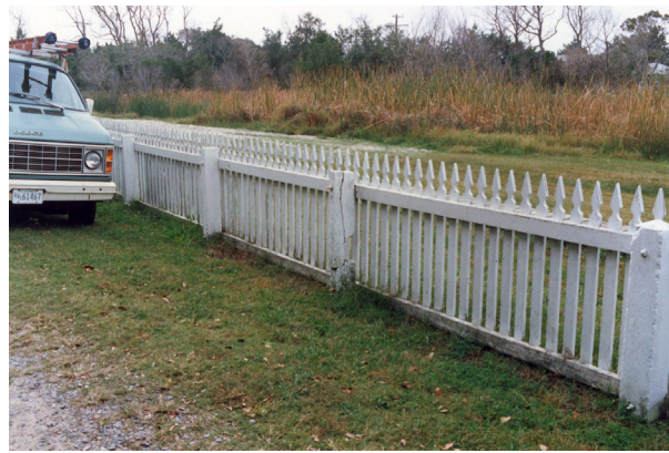
FIGURE 2–139. Picket fence (west), 1985. (NPS/CAHA Collection)
