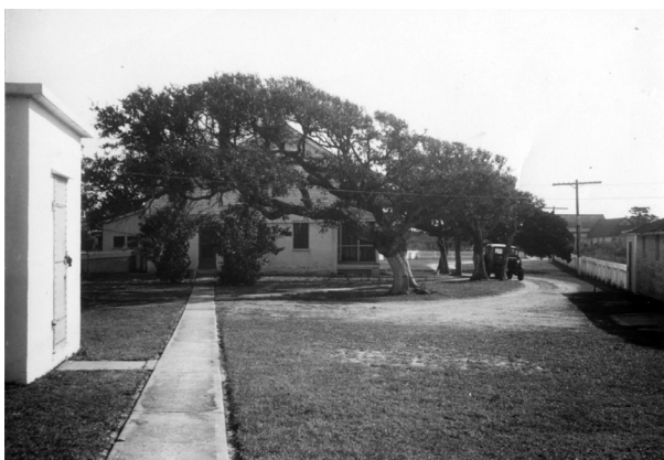
FIGURE 2-115. Walkway from dwelling to lighthouse, with other walkways in the background, 1955. (NPS/CAHA Collection)
