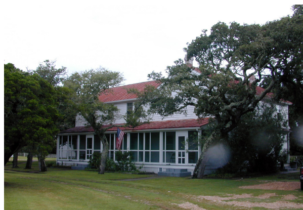
FIGURE 2-86. Double keepers' quarters, 2005. (NPS/CAHA Collection)
