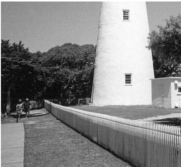
FIGURE 2-123. After construction of the boardwalk, 1994. (NPS/CAHA Collection)
