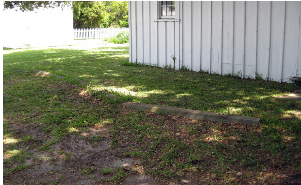
FIGURE 5-14. Concrete parking blocks north of the double keepers' quarters, 2013. (NPS/SER-CRPS Collection)
