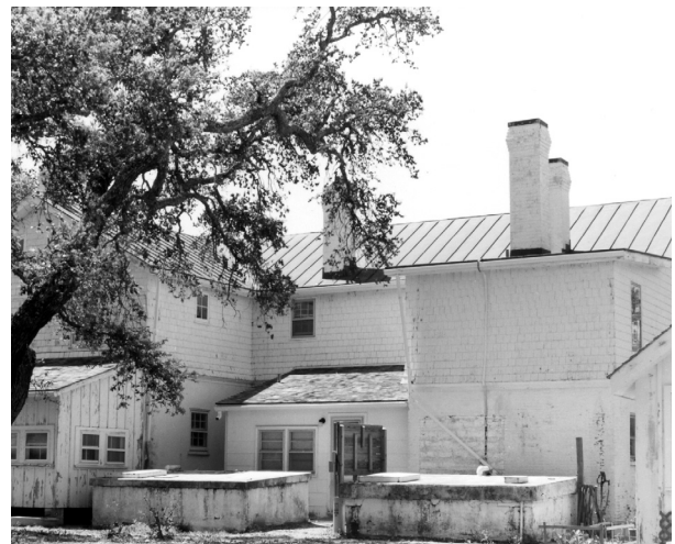
FIGURE 2-94. Cisterns, 1990. (NPS/CAHA Collection)
