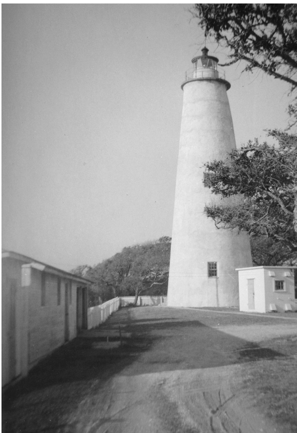
FIGURE 2-100. Garage and shed along the fence, n.d. (NPS/CAHA Collection)
