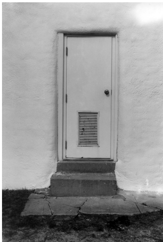
FIGURE 2-73. Exterior view of flat metal door, 1990. (NPS/CAHA Collection)
