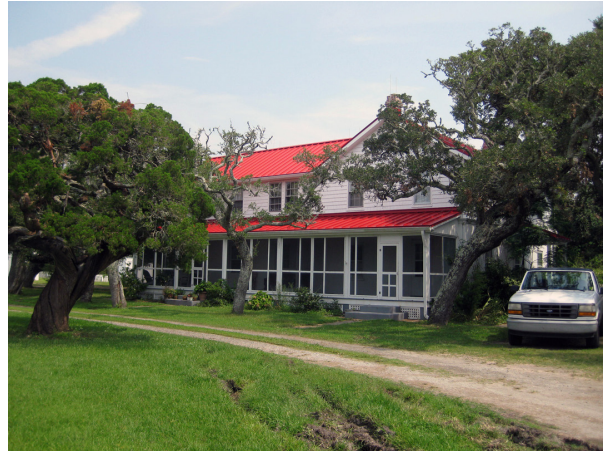
FIGURE 3–26. Double keepers' quarters, 2014. (NPS/SER-CRPS Collection)
