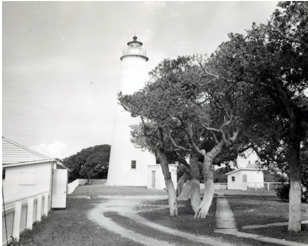
FIGURE 2-45. Ocracoke Light Station, 1954, with garage in the foreground and chicken house in the background. (NPS/CAHA Collection)
