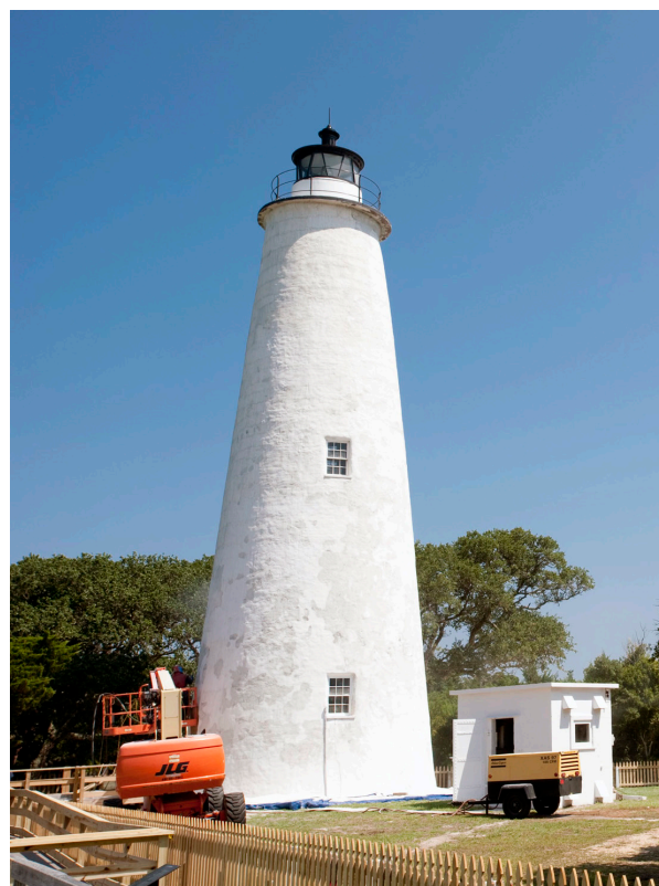
FIGURE 2-78. Work on the lighthouse, 2010. (NPS/CAHA Collection)
