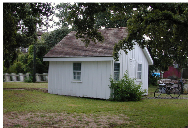
FIGURE 2-145. Storehouse before addition of edging, 1995. (NPS/CAHA Collection)
