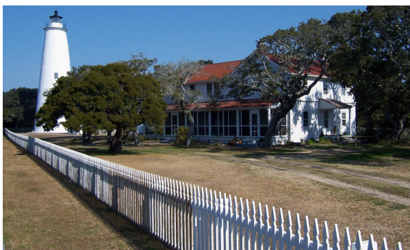
FIGURE 2-143. Picket fence (west), 2005. (NPS/CAHA Collection)
