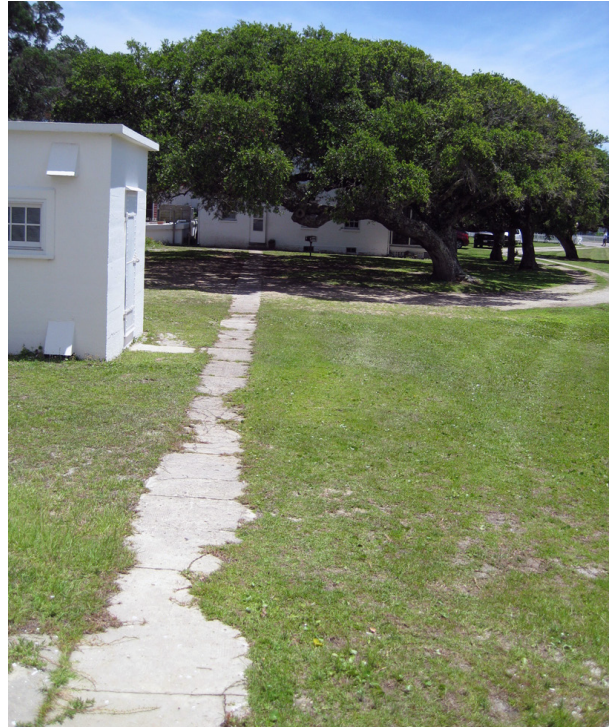
FIGURE 5-8. Concrete walkway linking the double keepers' quarters and the lighthouse, 2013. (NPS/SER-CRPS Collection)
