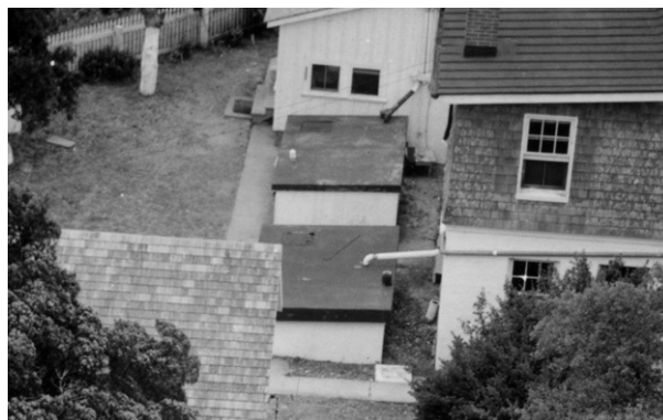
FIGURE 2-92. Cisterns, 1941. (NPS/CAHA Collection)
