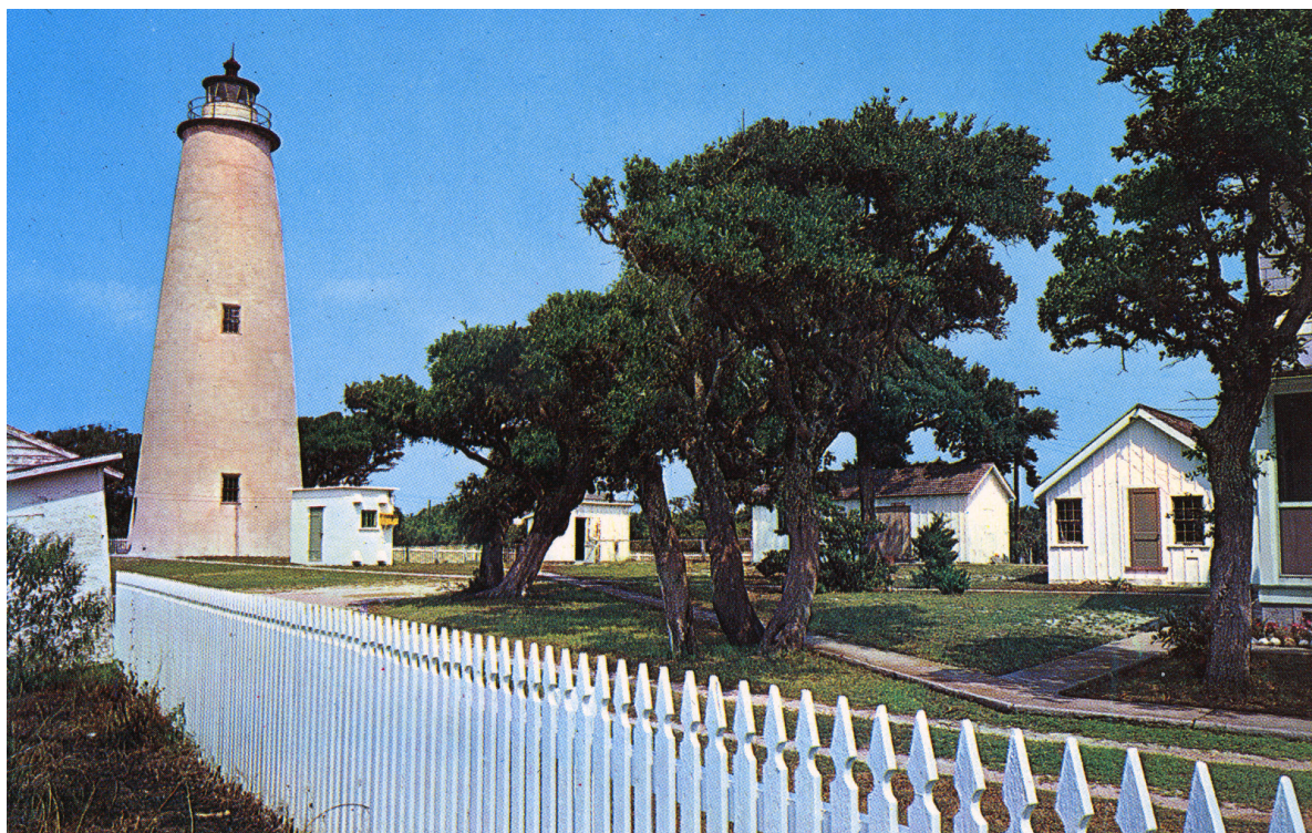
FIGURE 2–25. Ocracoke Light Station with garage, concrete oil house, chicken house, carpenter shop, and storehouse, ca. 1960s. (The Outer Banks History Center, Manteo, NC/Aycock Brown Collection)
