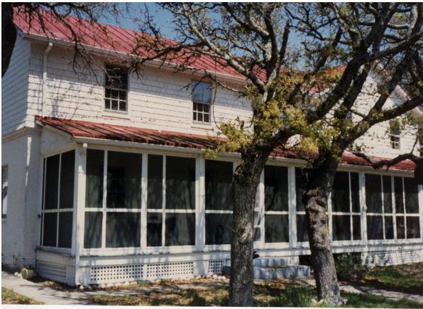
FIGURE 3–21. Double keepers' quarters before the addition of ornamentals, 1987. (NPS/CAHA Collection)
