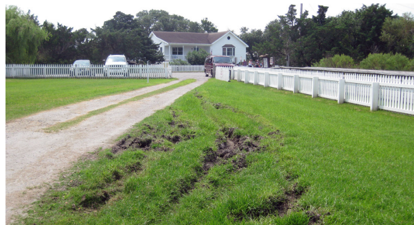
FIGURE 3–36. Deep ruts along entry road, 2014. (NPS/SER-CRPS Collection)
