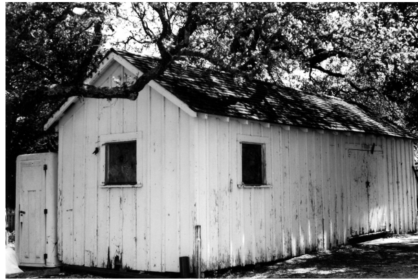
FIGURE 2–102. Carpenter shop, 1990. (NPS/SER-CRPS Collection)
