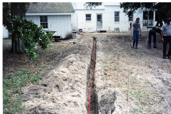
FIGURE 2-51. Utility trench excavation, 1987. (NPS/CAHA Collection)
