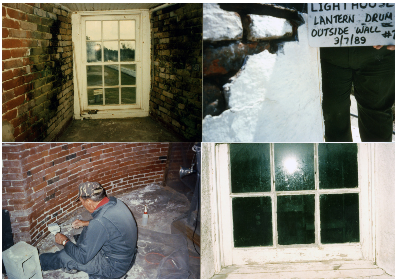
FIGURE 2-33. Work on the lighthouse, 1989. (NPS/CAHA Collection)
