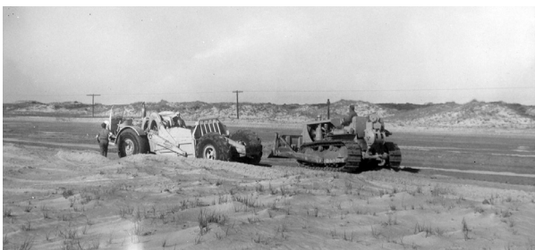
FIGURE 2-131. Building the road on Ocracoke, 1956. (NPS/CAHA Collection)
