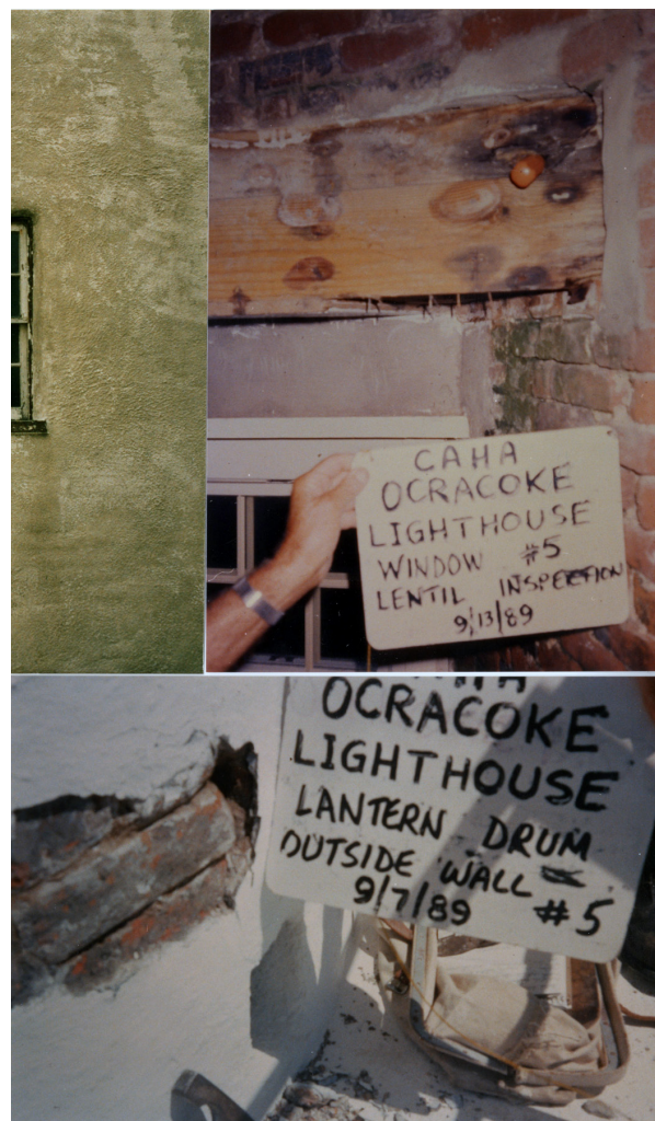
FIGURE 2-75. Crews inspecting the lighthouse, 1989. (NPS/CAHA Collection)
