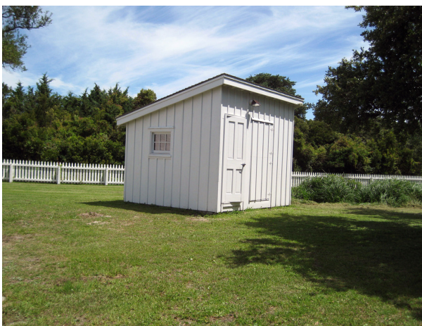
FIGURE 3–33. Generator house, 2013. (NPS/SER-CRPS Collection)
