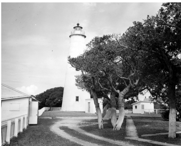
FIGURE 2-113. Series of walkways linking the buildings on site, 1954. (NPS/CAHA Collection)
