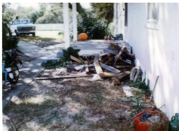
FIGURE 2-27. Condition of the site, ca. 1986. (NPS/CAHA Collection)
