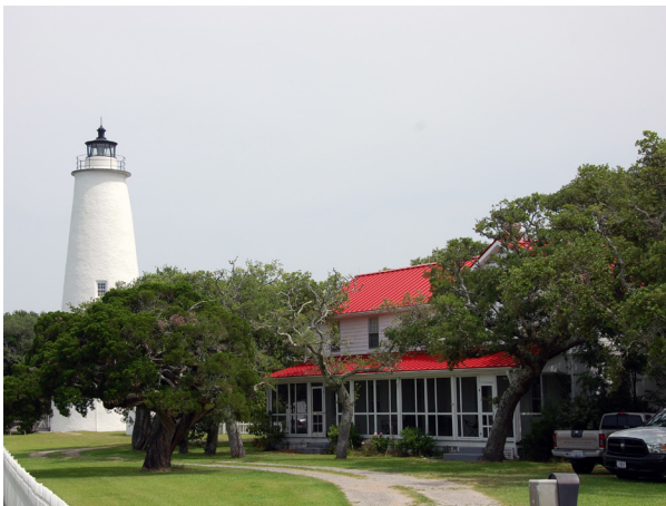
FIGURE 3–18. Live oaks and cedars looking towards the double keepers' quarters, 2014. (NPS/SER-CRPS Collection)
