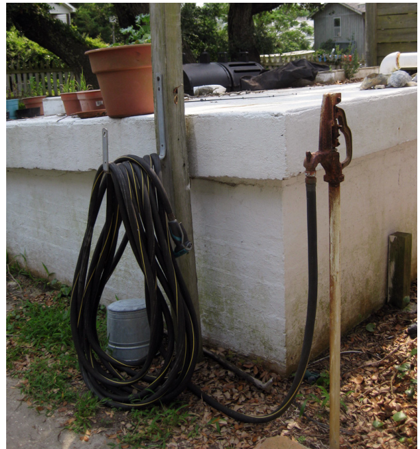
FIGURE 3-60. Yard hydrant attached to garden hose, 2014. (NPS/SER-CRPS Collection)
