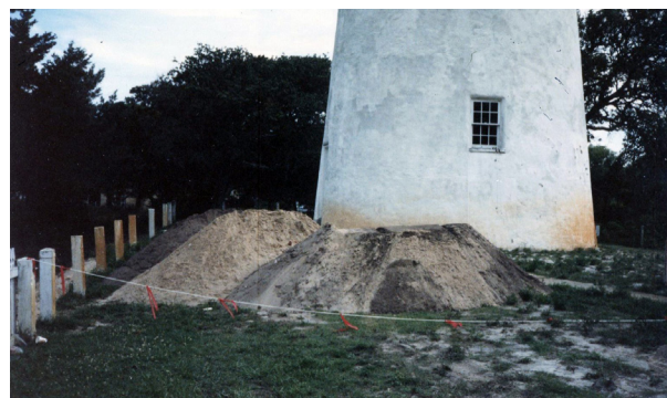
FIGURE 2–142. Picket fence (west), 1987. (NPS/CAHA Collection)
