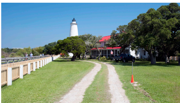
FIGURE 2-144. New pickets installed in 2010. (NPS/CAHA Collection)
