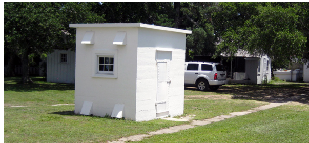
FIGURE 3–27. Concrete oil house, 2013. (NPS/SER-CRPS Collection)
