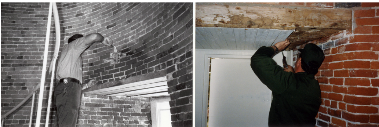
FIGURE 2-76. Crews completing Phase III work on the lighthouse, 1991. (NPS/CAHA Collection)
