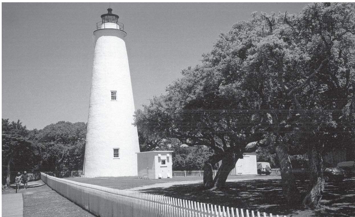
FIGURE 2-35. Lighthouse tower with boardwalk in the foreground and new generator building in the background, 1994. (NPS/CAHA Collection)
