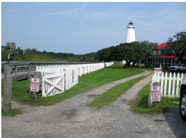
FIGURE 3-5. Front entry gate, 2014. (NPS/SER-CRPS Collection)
