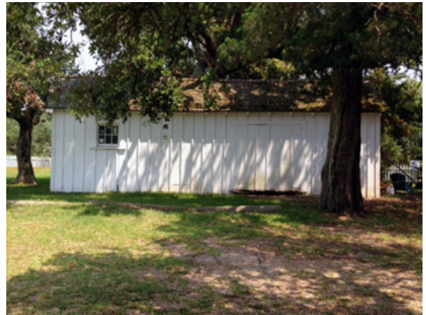
FIGURE 3-31. Carpenter shop, 2014. (NPS/SER-CRPS Collection)
