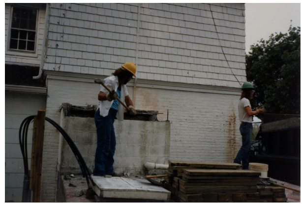
FIGURE 2-93. Cistern repair, 1987. (NPS/CAHA Collection)
