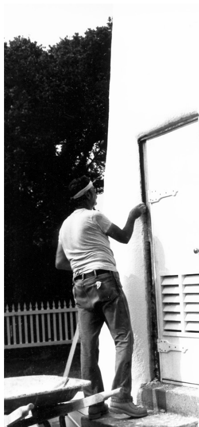
FIGURE 2-74. Newly installed historic character door, 1990. (NPS/CAHA Collection)
