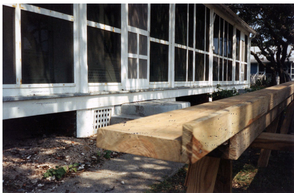
FIGURE 2-84. Rehabilitation work, 1987. (NPS/CAHA Collection)
