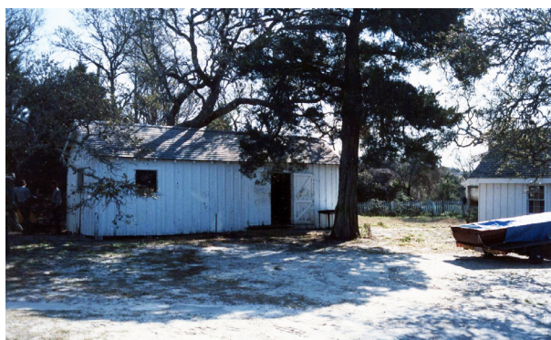
FIGURE 2-66. Sandy conditions of the site with carpenter shop in the background, 1987. (NPS/CAHA Collection)
