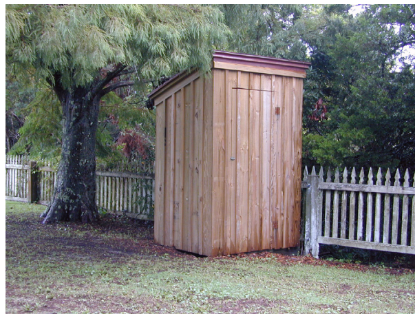
FIGURE 2-108. Privy, 2005. (NPS/CAHA Collection)
