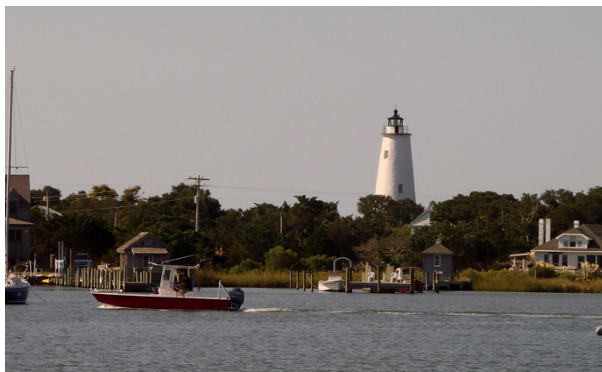
FIGURE 3-54. View of the lighthouse from the harbor, 2013. (© Joseph K. Oppermann - Architect)
