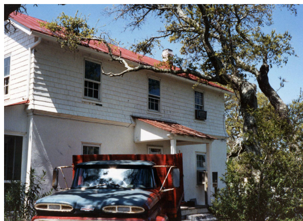
FIGURE 2-29. Phase I rehabilitation, 1987. (NPS/CAHA Collection)
