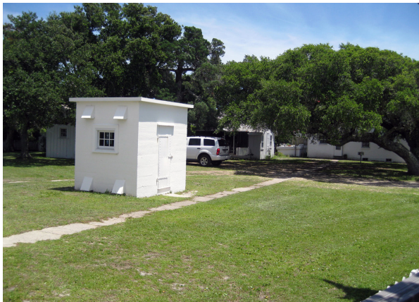
FIGURE 3-9. Looking south toward the storehouse, carpenter shop, and cisterns, 2013. (NPS/SER-CRPS Collection)
