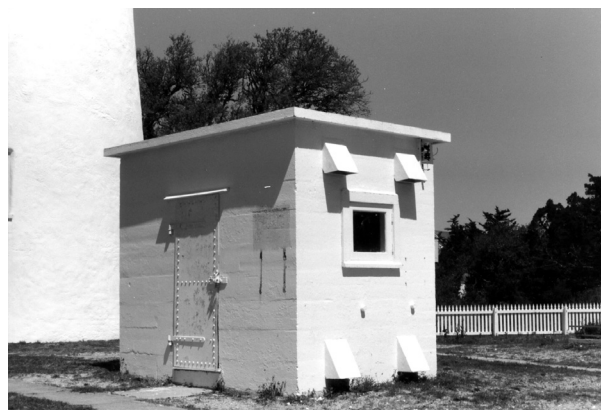
FIGURE 2-90. Concrete oil house, 1990. (NPS/SER-CRPS Collection)
