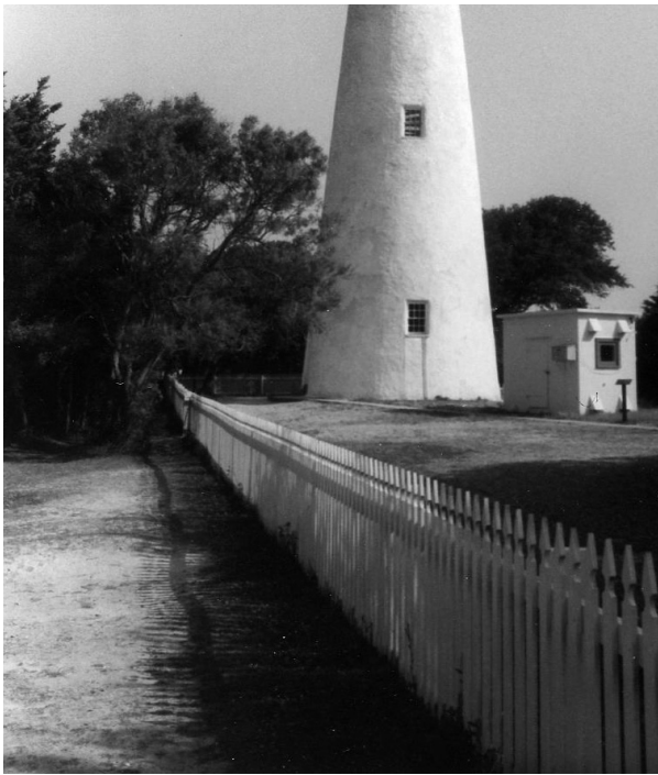
FIGURE 2-122. Prior to the construction of the boardwalk, 1984. (NPS/CAHA Collection)
