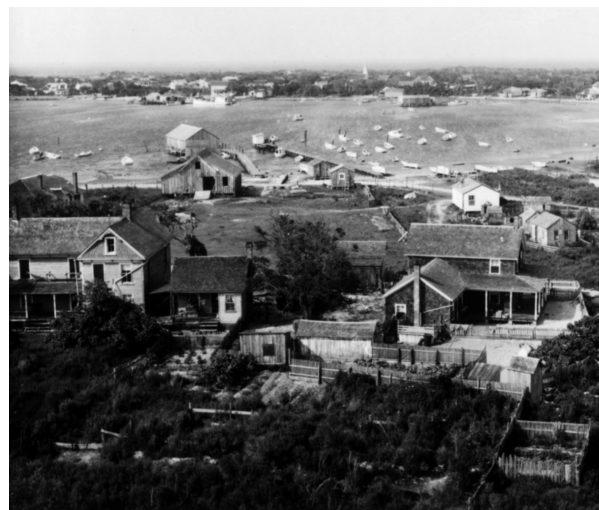
FIGURE 2-137. Aerial view of fence types seen from the lighthouse, 1936. (NPS/CAHA Collection)
