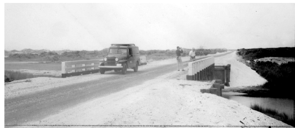
FIGURE 2-132. Bridge construction on Ocracoke, 1957. (NPS/CAHA Collection)
