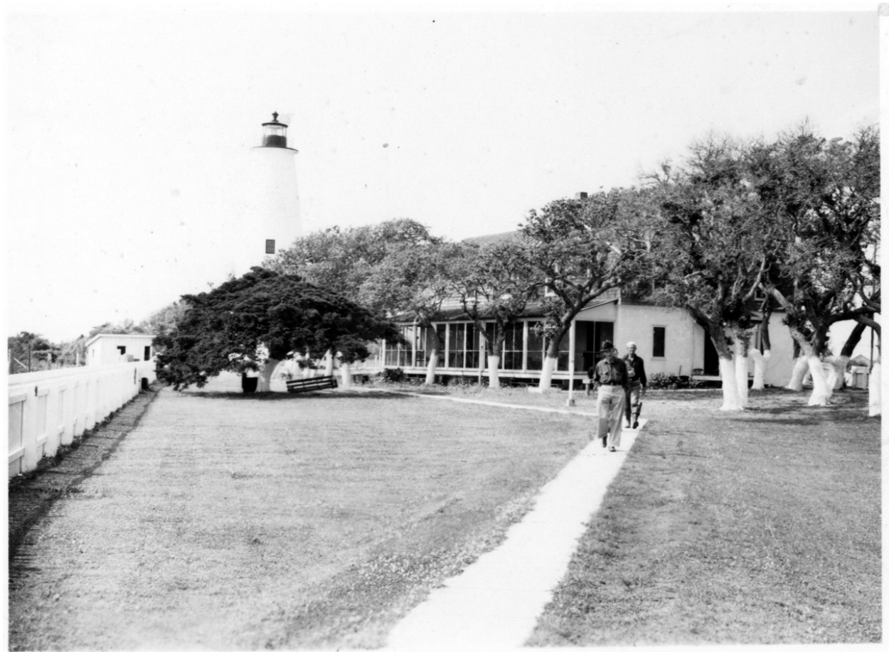
FIGURE 2-118. Walkway into the light station, 1936. (NPS/CAHA Collection)
