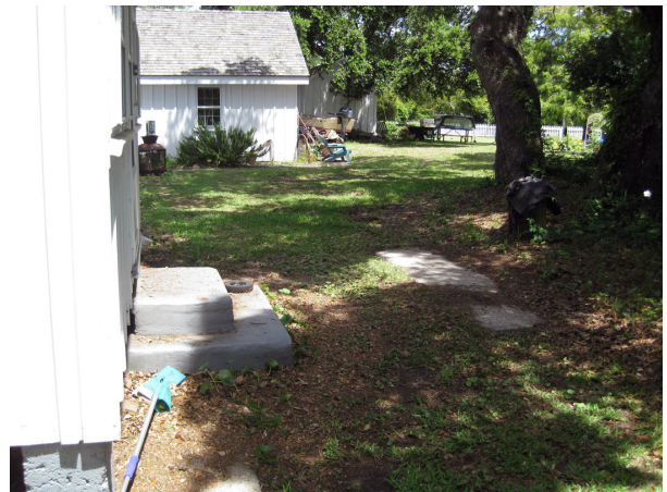
FIGURE 5-9. Section of concrete walkway on the east side of the double keepers' quarters disappearing into the grass, 2013. (NPS/SER-CRPS Collection)
