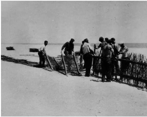
FIGURE 2-53. Fencing being erected, 1938. (NPS/CAHA Collection)
