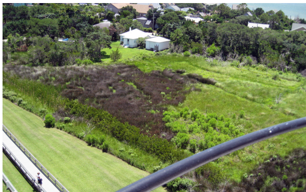
FIGURE 3-53. View to the west, 2013. (NPS/SER-CRPS Collection)
