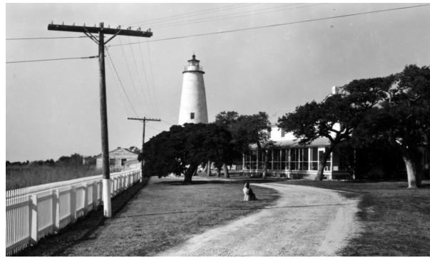
FIGURE 2–148. Telephone poles, 1960. (NPS/CAHA Collection)
