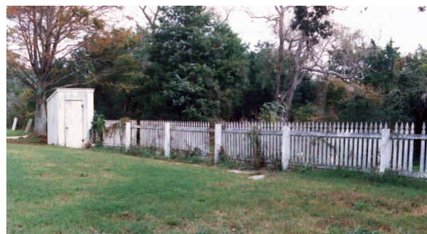
FIGURE 2-105. Privy, 1985. (NPS/CAHA Collection)
