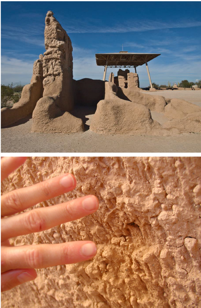
Figure 7. Photographs of caliche walls. Structures at the monument were built using a technique referred to as “English cob” or “puddled adobe” where stiff caliche mud is piled up by hand to form a wall. When the mud dries, it becomes like concrete. Top: NPS photograph (from National Park Service 2017, p. 6). Bottom: Photograph by Katie KellerLynn (Colorado State University).
