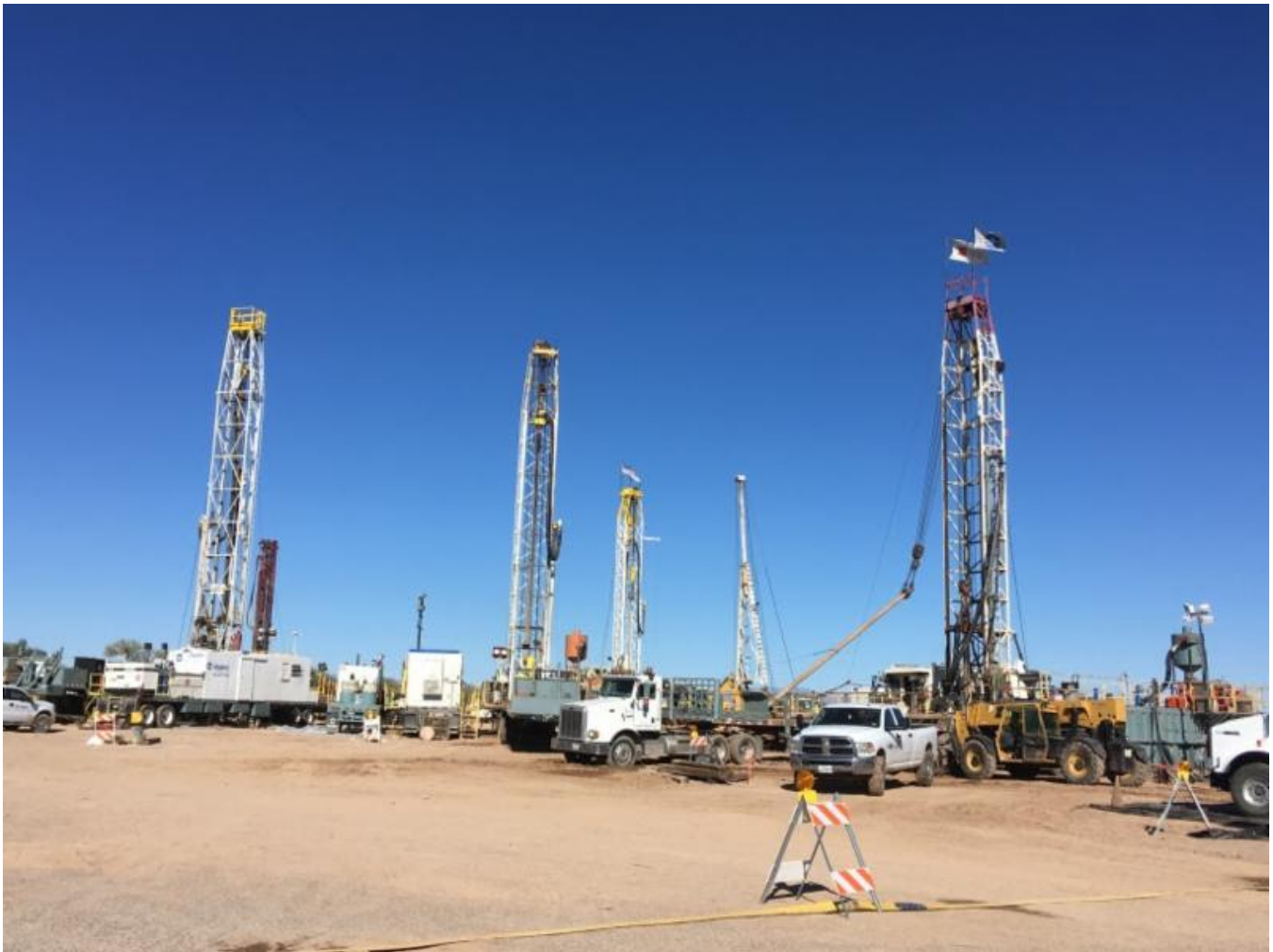
Figure 12. Photograph of drill rigs at Florence Copper. The Florence Copper production test facility is 12 km (7 mi) northeast of the monument (see fig. 3). The operation, which is presently under construction, is for in situ copper recovery (ISCR). As of March 2018, five drill rigs were working 24/7 to install injection and recovery wells, monitoring wells, and replacement irrigation wells. Florence Copper Inc. photograph available at https://www.florencecopper.com/media/photo-gallery (accessed 7 August 2018). Used by permission.
