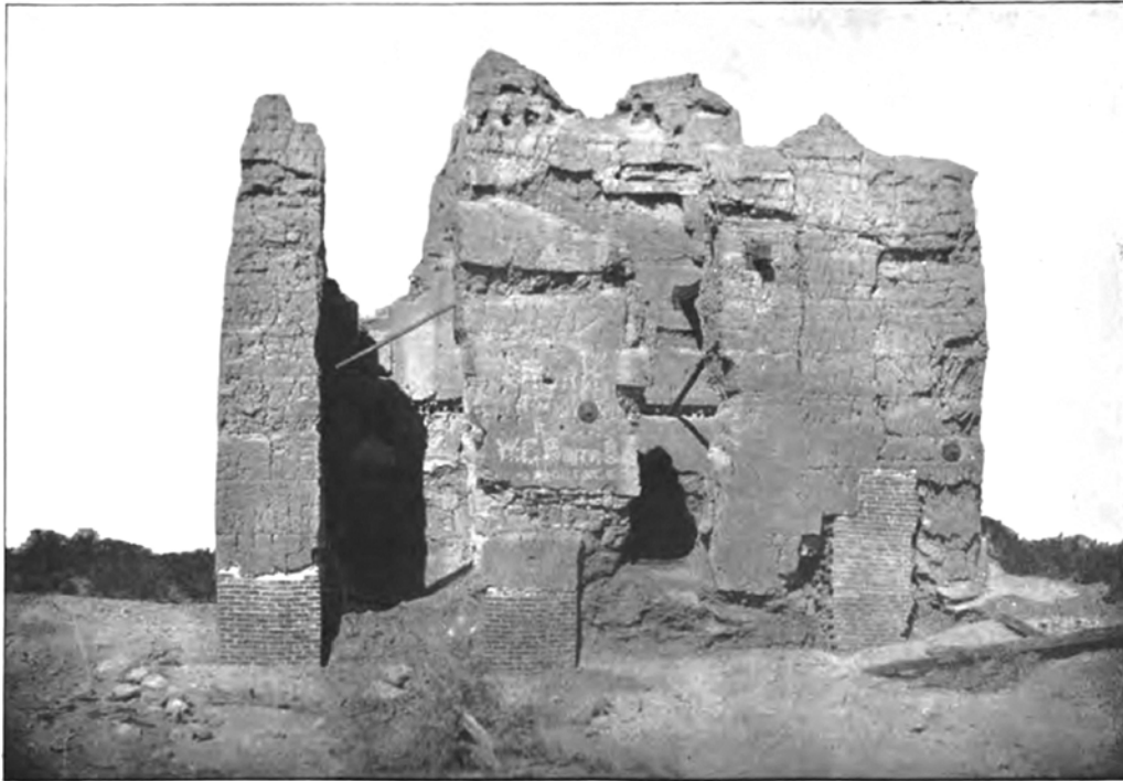
Figure 49. South façade of the Casa Grande Ruin in 1891, showing new brick underpinning and tie-rods. Image taken before cement coping applied. Photographer H. H. Burrell. Mindeleff (1897).
