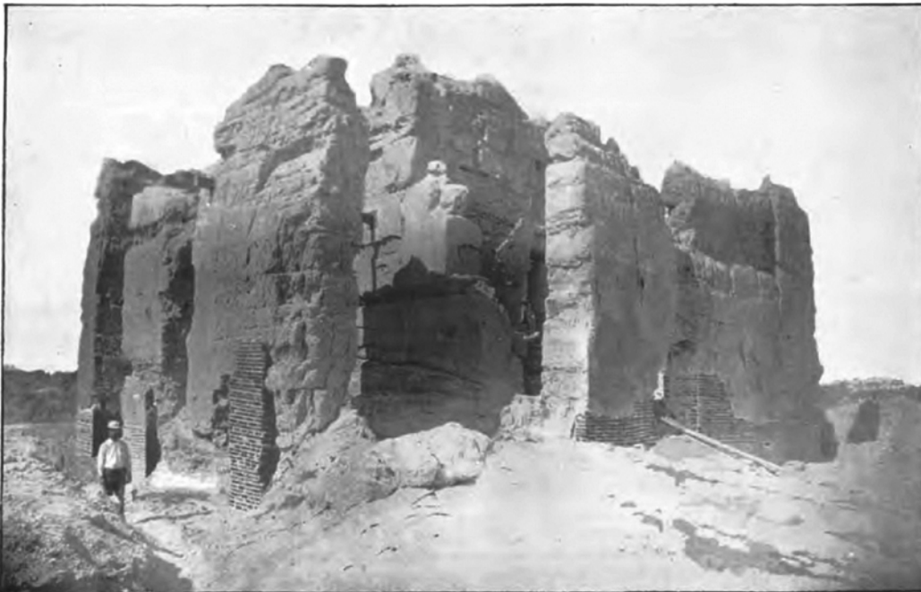
Figure 50. Southeast corner of the Casa Grande Ruin in 1891, showing repair work. Photographer H. H. Burrell. Mindeleff (1897).
