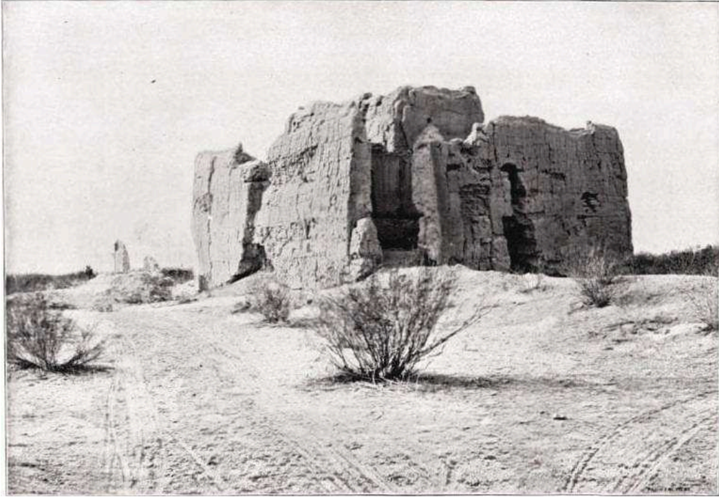
Figure 60. General View of Casa Grande from the northeast, showing stagecoach ruts, 1890-91. Mindeleff (1896).
