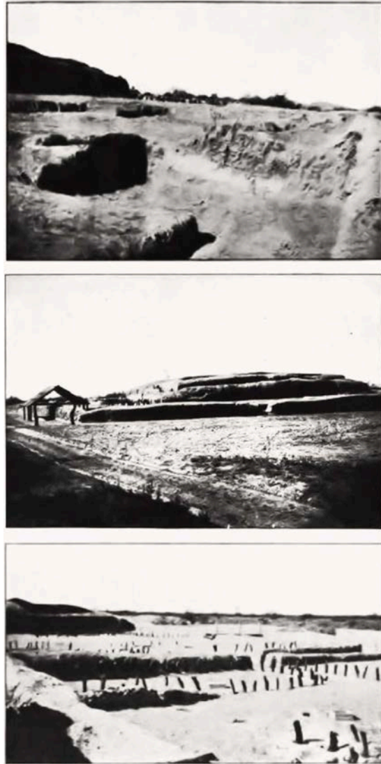
Figure 110. Compound B rooms. (Top) Subterranean rooms in the northeast corner. (Middle) Protective roof over excavated subterranean room in northeast corner of Compound B. (Bottom) Rooms west of Pyramid A in Compound B. Fewkes (1912).
