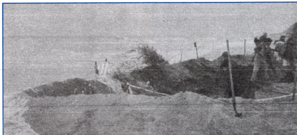
Storm waves break through the protective berm at the Carns site excavation, 1991.
