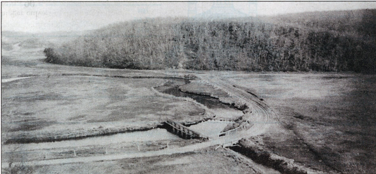
Open salt marsh, 1903. View from Bound Brook Island across the Herring River flood plain to Merrick Island, Wellfleet.
