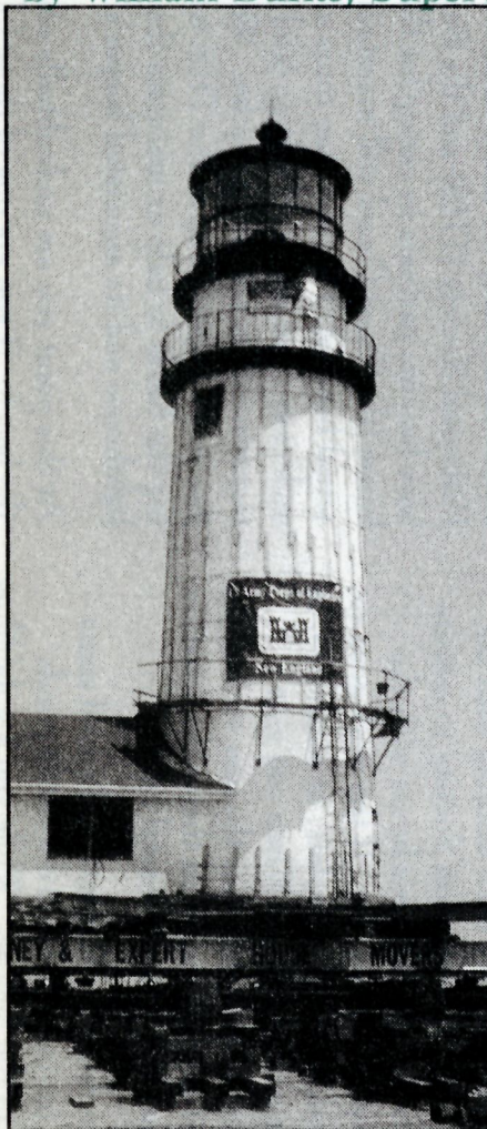
Highland Lighthouse move
