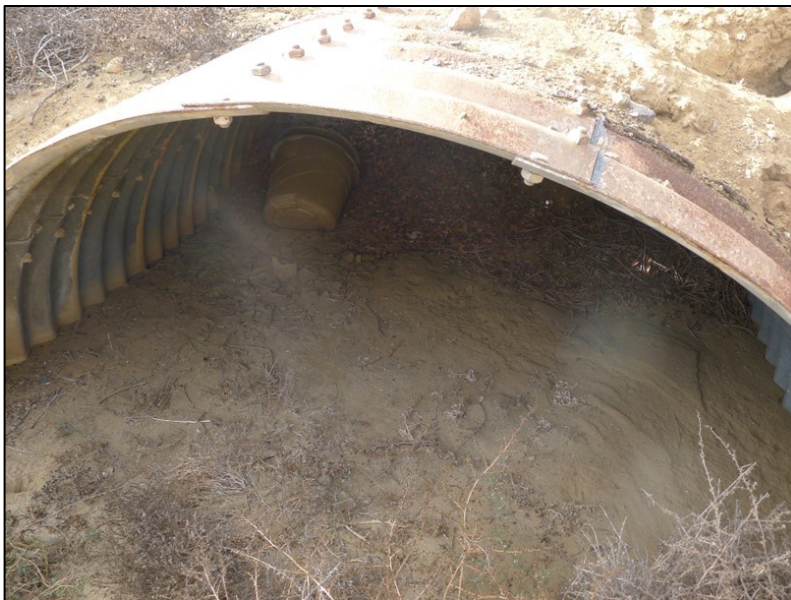
Buildings and Structures #12. One of six smaller, earth covered corrugated metal, barrel vaulted bunkers at Battery Point Loma. View of the filled interior of the southernmost of the small bunkers (PWRO, November 2017).
