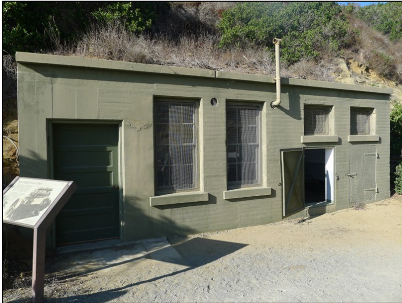
Buildings and Structures #5. View of the Generator Station for Searchlight No. 18 & 19, looking northwest (PWRO, November 2017).
