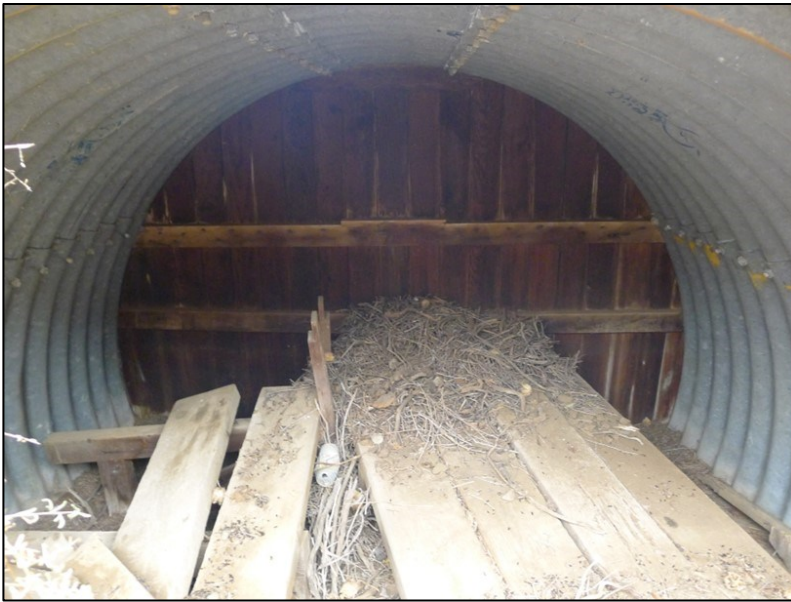
Buildings and Structures #10. One of six smaller, earth covered corrugated metal, barrel vaulted bunkers at Battery Point Loma. View of the interior of the northernmost bunker of the Battery Point Loma Bunker Complexes (for all four gun mounts) (PWRO, November 2017).
