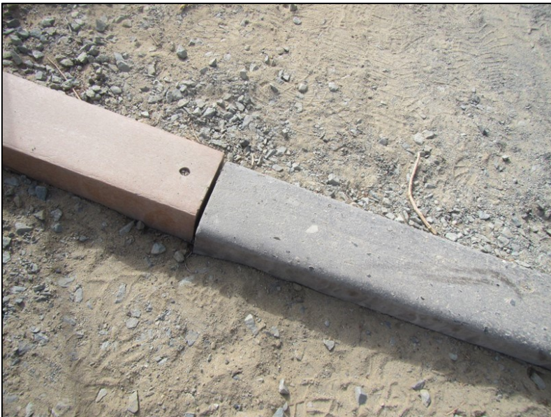
Circulation #4. Precast concrete and composite water bars along Bayside Trail (PWRO, November 2017).
