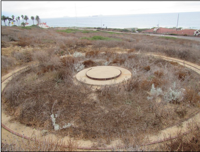
Buildings and Structures #13. View of the Battery Point Loma Panama Gun Mount 4, looking southwest (PWRO, November 2017).
