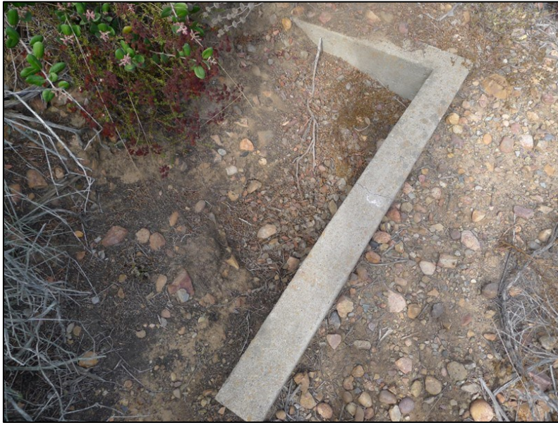
Buildings and Structures #15. An example of the historic culvert headwalls found along Bayside Trail, with a wing wall (PWRO, November 2017).
