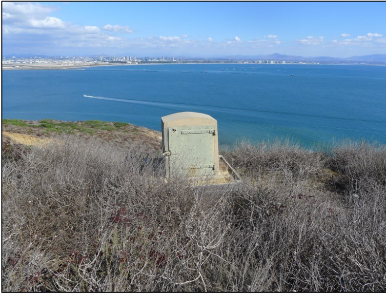
Buildings and Structures #3. View of the Electrical Connection Box, looking northeast (PWRO, November 2017).
