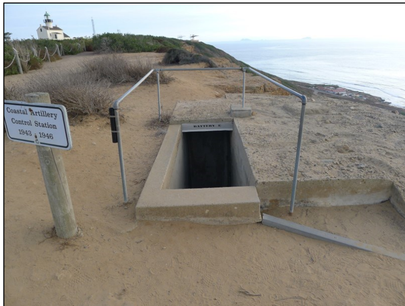
Small-Scale Features #4. Building marker sign located by the entrance to Battery Command and Base-End Station, Battery Ashburn (PWRO, November 2017).).
