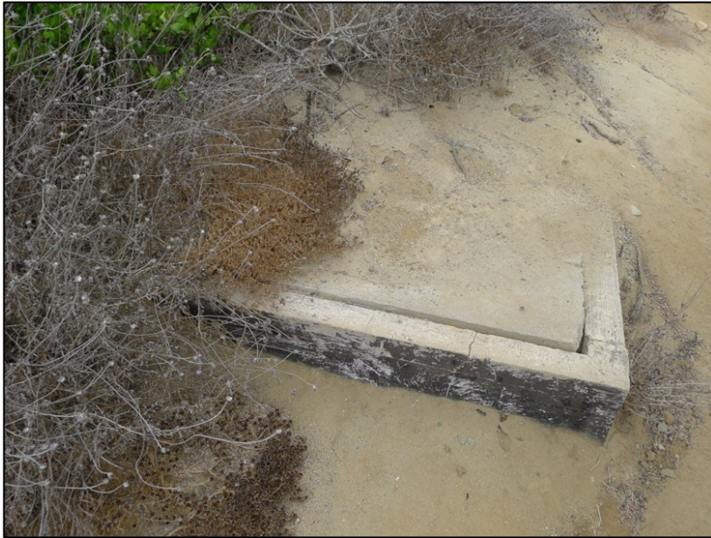
Archaeological Sites #1. The exposed corner of the Generator Station for Searchlight No.15 (PWRO, November 2017).
