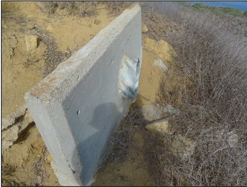
Buildings and Structures #17. An example of the modern culvert end wall found along Bayside Trail (PWRO, November 2017).
