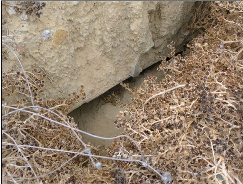
Buildings and Structures #11. A sample of the smaller, earth covered bunkers at Battery Point Loma Bunker Complexes. View of the almost completely buried bunker, the third structure from north (PWRO, November 2017).
