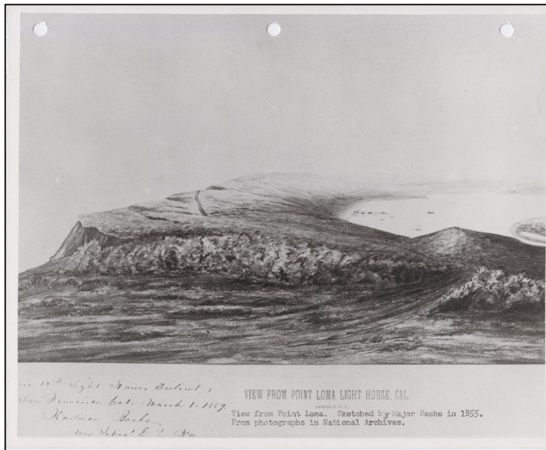
Physical History #3. View northward from the approximate location of the old Point Loma lighthouse. Major Hartman Bache, March 1, 1859. From: F. Ross Holland, Old Point Loma Lighthouse Historic Structures Report, US Department of the Interior, National Park Service, 1964.
