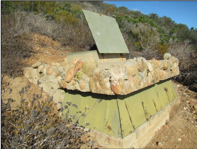
Buildings and Structures #7. One of five World War I-era pillbox base-end stations at the monument. View of Base End Station, Batteries Calef and Wilkeson, looking northwest. The other four of such structures are: Battery End Station, Batteries Calef and Wilkeson, Upper and Lower Base-End Stations at Billy Goat Point, and Base End Station, Battery McGrath. All five of these structures are located on the eastern side of Point Loma (PWRO, November 2017).
