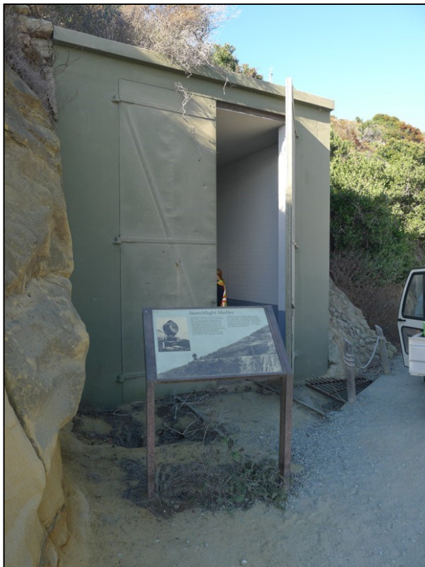
Buildings and Structures #4. View of Searchlight Shelter No. 18, looking northwest from the Bayside Trail (PWRO, November 2017).
