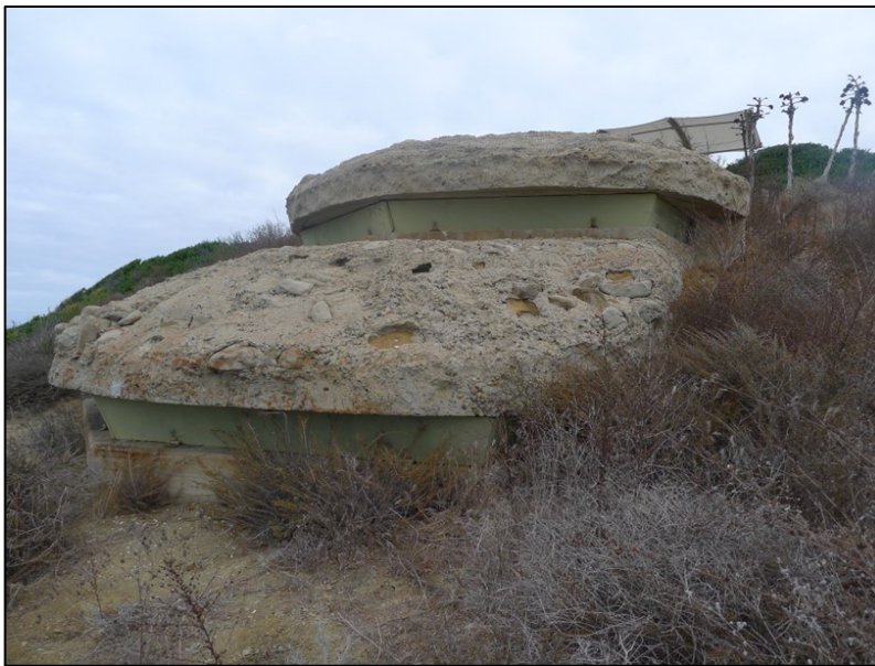
Buildings and Structures #2. A sample of the three split-level domed observation stations at CABR. View of the Base-End Station, Batteries Woodward and Grant, looking northeast. The other two stations of this style are Battery Commander and Base-End Station, Battery Ashburn and Battery Commander Station, Battery Humphreys. All three of these stations are located on the western side of Point Loma (PWRO, November 2017).
