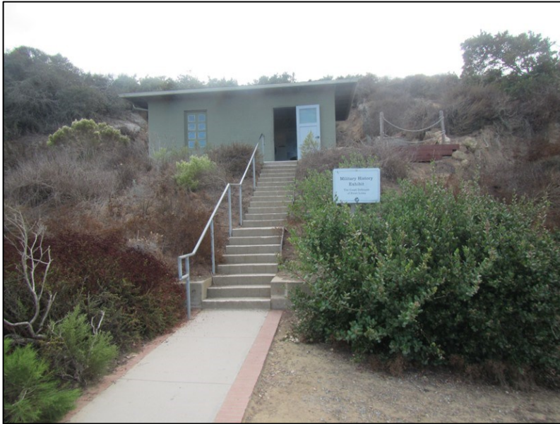
Buildings and Structures #1. View of the of the Army Radio Station façade, looking southwest from the Catalina Blvd. alignment (PWRO, 2017).
