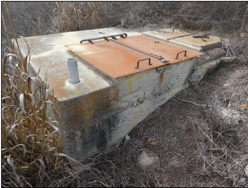
Buildings and Structures #18. View of Manhole 104, looking southwest (PWRO, November 2017).
