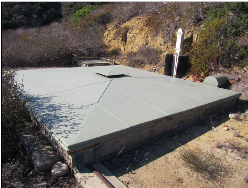
Buildings and Structures #6. One of two subterranean searchlight shelters at the monument. View of Searchlight Shelter No.19, looking southwest. The other subterranean searchlight shelter is Searchlight Shelter No.15 (PWRO, November 2017).
