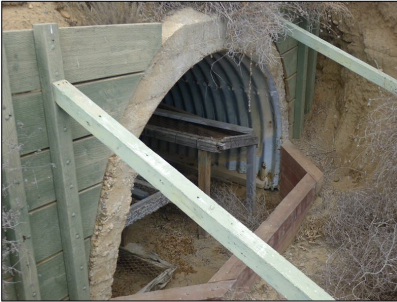
Buildings and Structures #9. One of two concrete covered corrugated metal, barrel vaulted bunkers of the Battery Point Loma. View of Battery Point Loma Bunker Complex Gun 1 & 2, south end (PWRO, November 2017).
