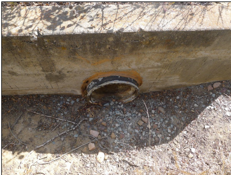
Buildings and Structures #16. An example of the corrugated metal culverts found along Bayside Trail (PWRO, November 2017).
