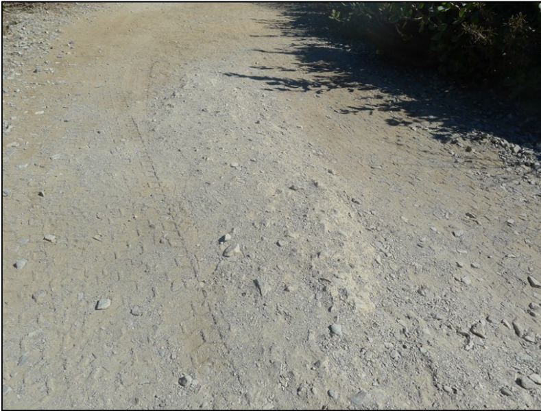
Circulation #3. Remnant road surface along Bayside Trail (PWRO, November 2017).
