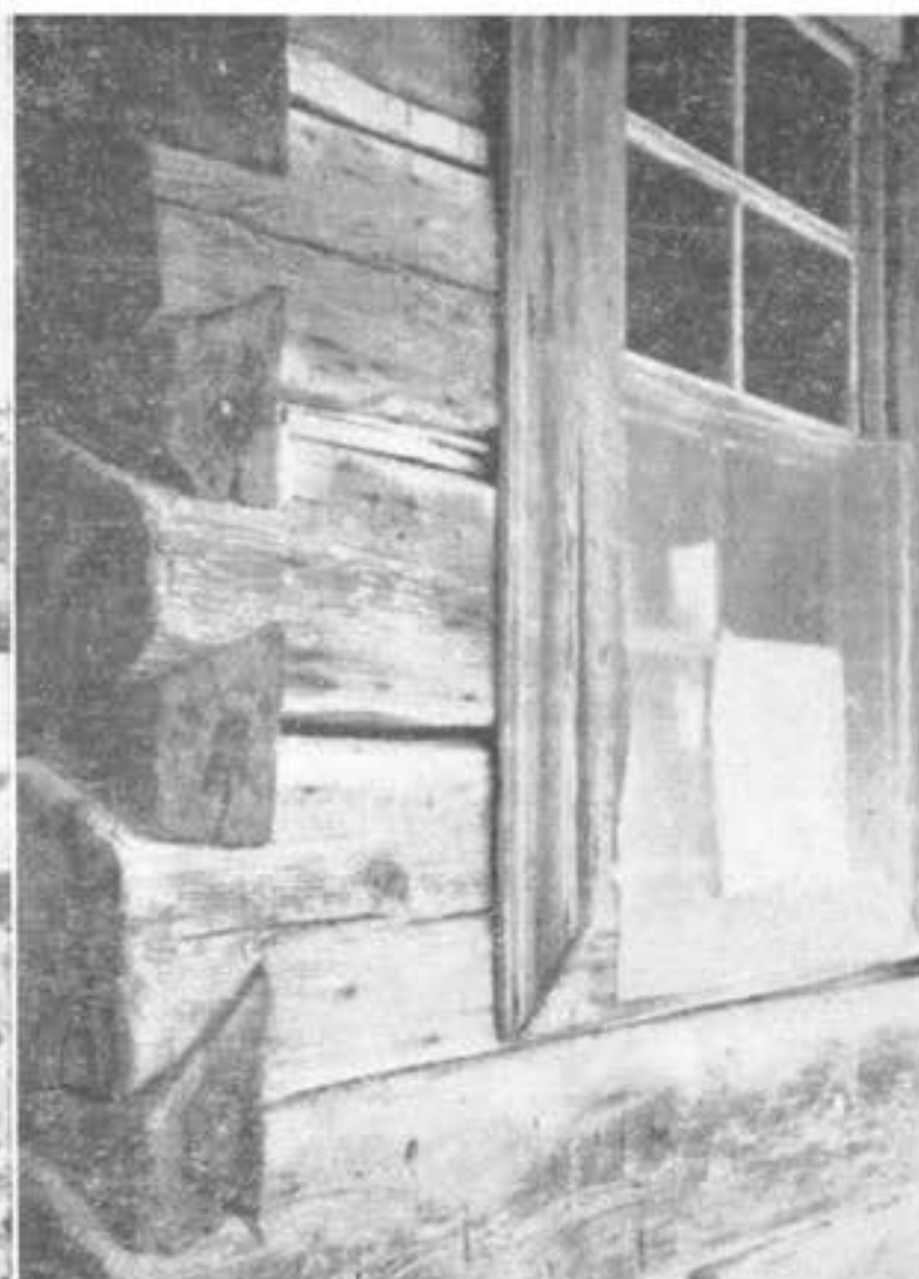
Carefully notched and fitted logs of the original house, Edwards' Store.
