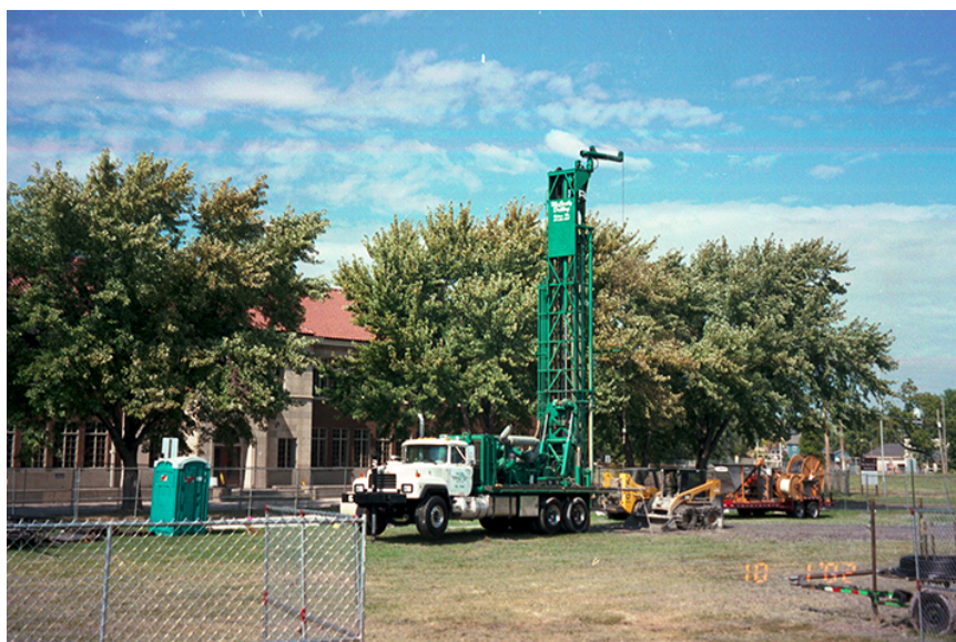
Figure 22. Digging a well for the geothermal system, 2001. Photograph in files of Brown v. Board of Education NHP.
