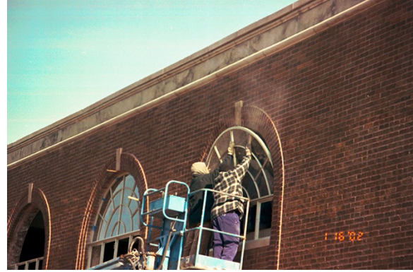
Figure 20. Installation of restored windows, 2001. Photographs in files of Brown v. Board of Education NHP.
