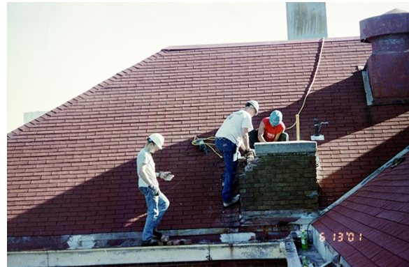
Figure 21. Rebuilding the brick chimney, 2001. Photographs in files of Brown v. Board of Education NHP.
