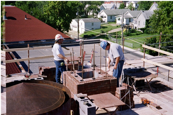
Figure 21. Rebuilding the brick chimney, 2001. Photographs in files of Brown v. Board of Education NHP.
