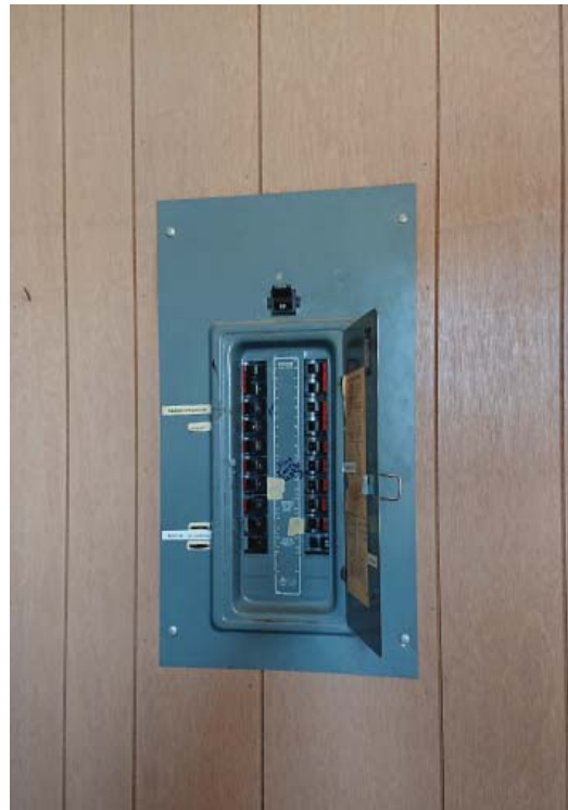
Relocate electrical panel.
