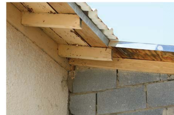
2 Roof deck board in this area has been replaced.
