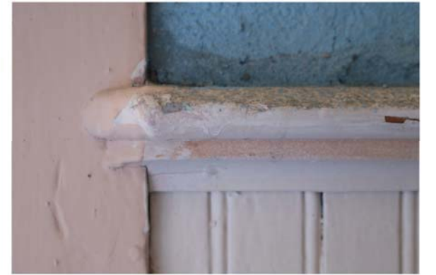
4 The cap and molding of the beaded board wainscot wraps the casing and is still visible in some areas.
