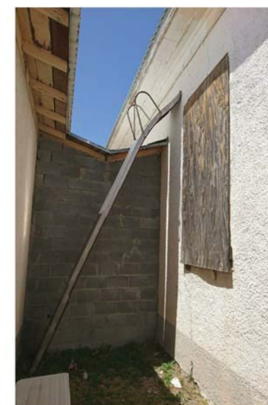
3 Plywood covers the window opening.
