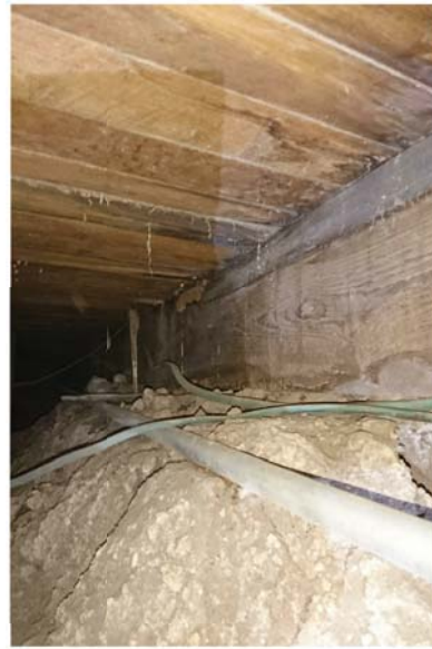
2 Rubble wall foundation has been modified and partially removed in this location for installation of indoor restrooms.
