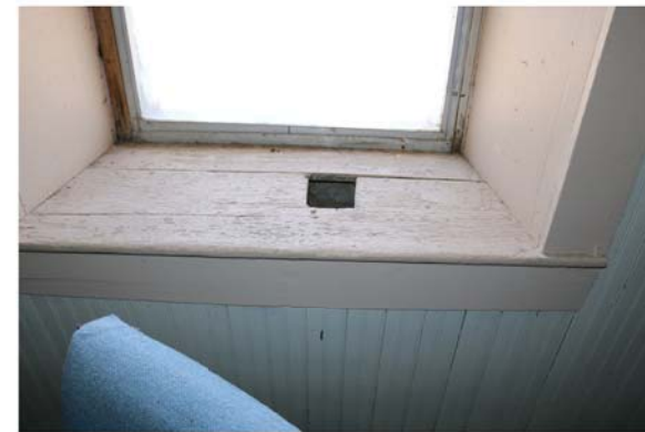
5 The deep window sill, or stool, is rounded and sits above the window apron. The stool has been cut for an unknown reason.
