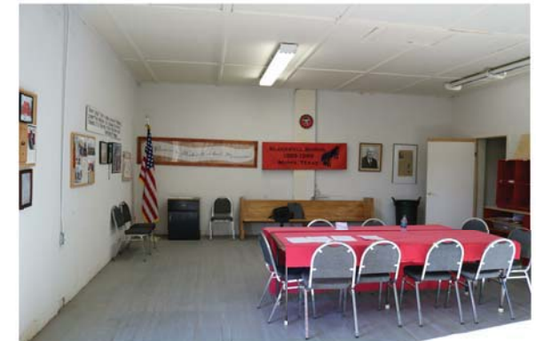
5 band hall interior elevation looking north. A wood nailer is seen at 33" above the floor for a possible chair rail.
