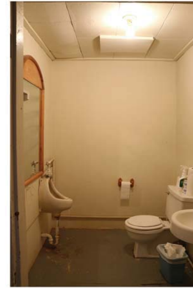
3 Ceiling in the boys and girls restroom is non-original 16" x 32" acoustical tile panels.
