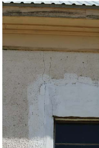
4 Modifications to the original window openings are visible at the stucco patching.
