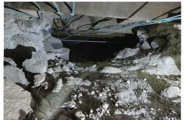
6 Portion of the foundation wall has been removed for access between the classroom and vestibule area.
