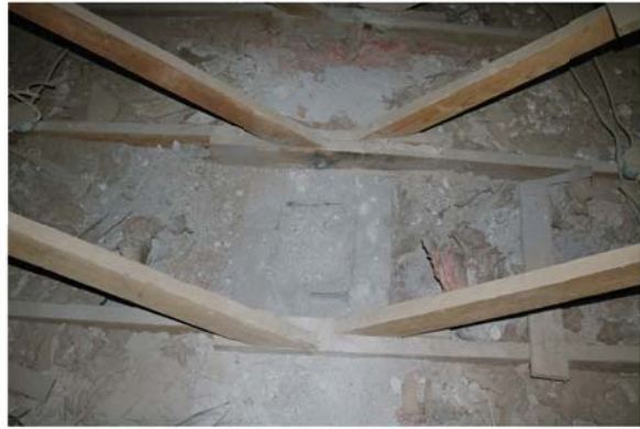
1 Embedded into the top of the adobe wall is the remains of an old brick chimney that has been removed.
