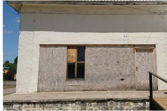
2 Infill wall at loading dock shows many modifications.
