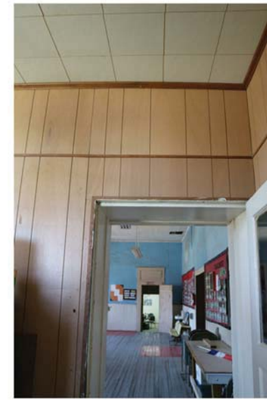
5 Wood veneer paneling covers original transom which is still intact and can be seen from other side.
