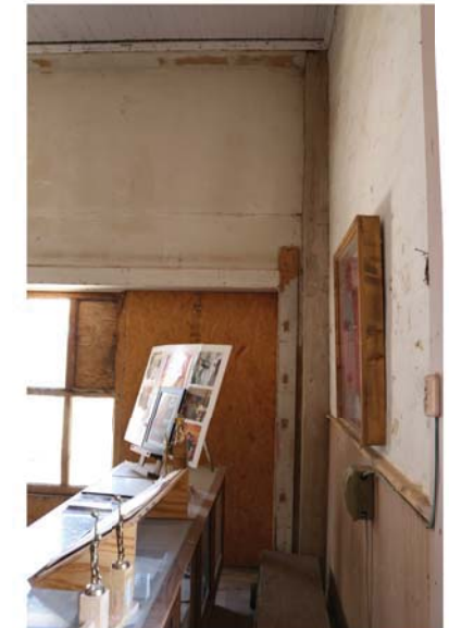
6 Concrete columns support the roof structure above, but do not bond with the adobe construction.
