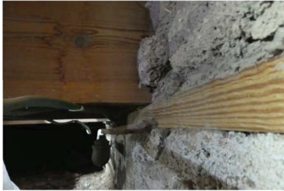
1 Rubble fondation wall with a wooden ledger embeded below the floor joists.
