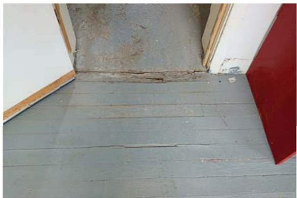
3 A roof leak in the connecting hallway has caused deterioration and rotted wood where the concrete ramp connection slopes toward the band hall.
