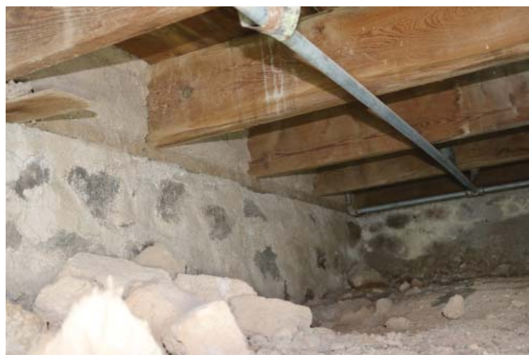
Evaluate under floor crawlspace plumbing and electrical lines.
