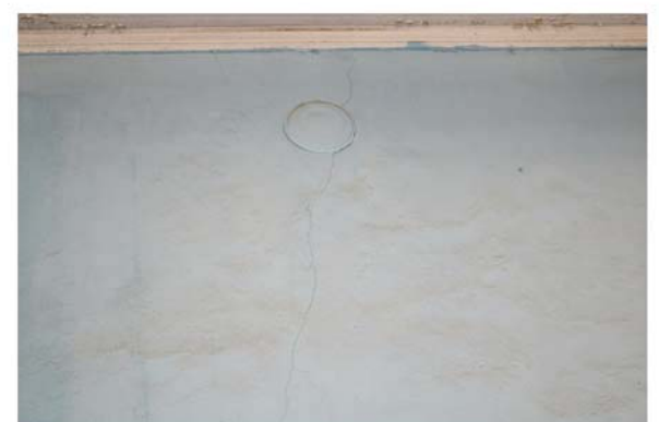
7 Metal plate caps opening for flue.
