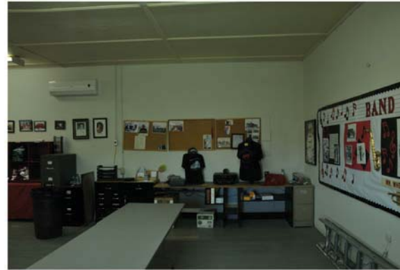
2 Ceiling In the band hall area has a series of 4' X 8' wood sheets with battens.
