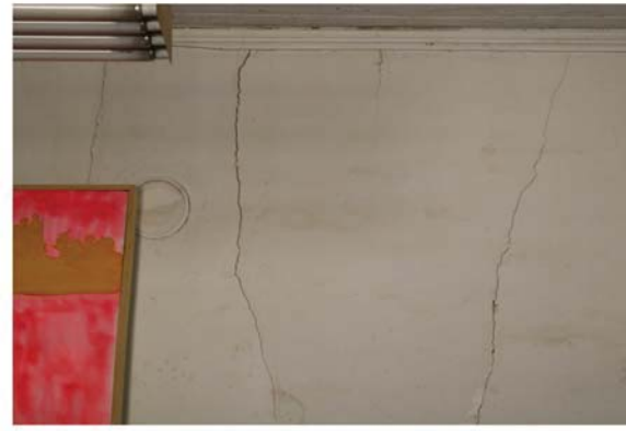
4 Metal plate covers opening for flue pipe to chimney which has been dismantled.
