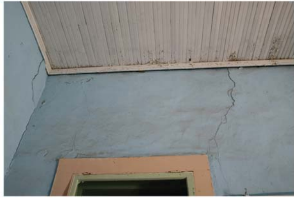
6 Numerous cracks and patched plaster above the door indicates movement has taken place in this wall. The direction of the crack at the upper right corner of the door indicates the center wall may have moved north after the removal of the original wall at the boys restroom.
