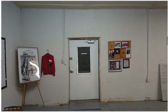
5 Non-original hollow metal door installed near the location of previous window.
