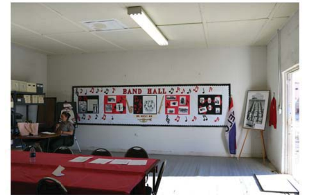
6 Another line indicated a wood base board was previously installed in the band hall.
