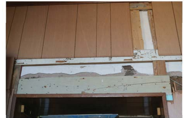
4 concrete lintel above blocked opening between office / storage area and south classroom.
