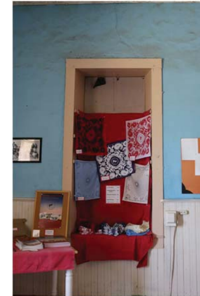
5 Window looks to band room and is blocked.
