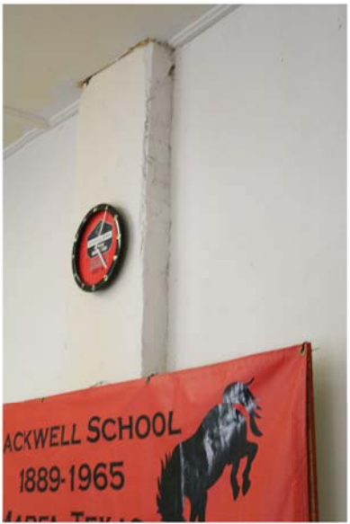
3 A brick chimney projects from face of clay tile wall.
