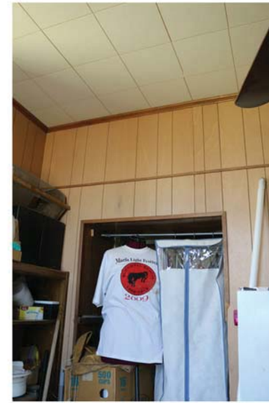
4 Ceiling in office is non-original acoustical ceiling tiles.
