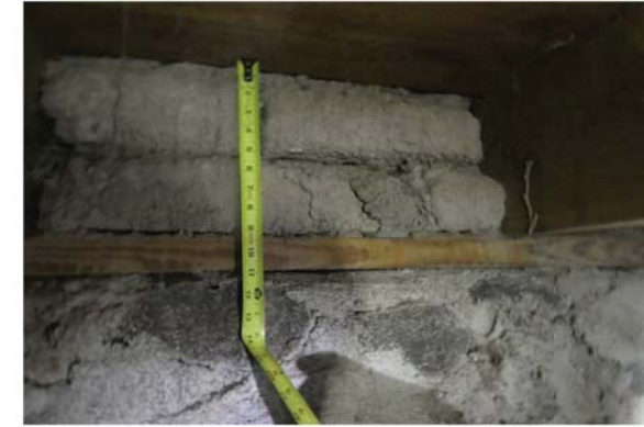
3 Adobe wall, wood ledger, and adobe brick units.
