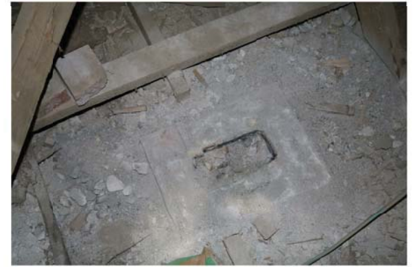
5 Embedded into the top of the adobe wall is the remains of an old brick chimney that has been removed.
