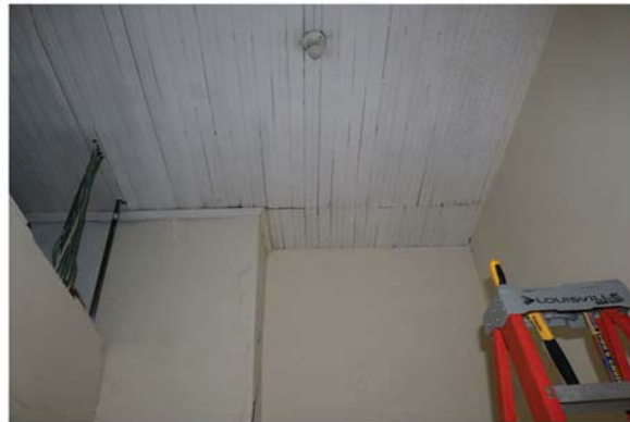
1 The beaded board tongue-and-groove ceiling boards in the vestibule are patched in where abobe wall was removed.
