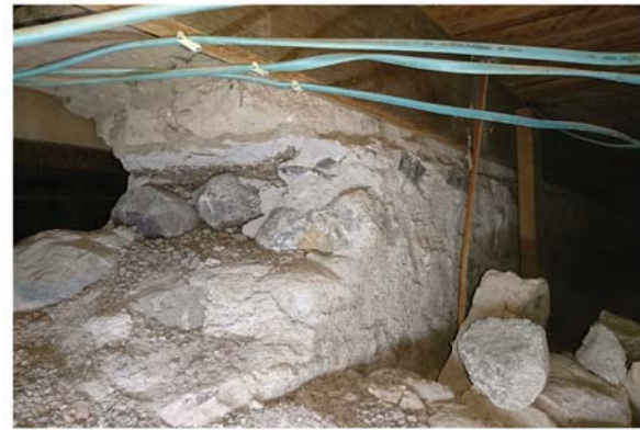
5 Portion of the foundation wall has been removed for access between the classroom and vestibule area.
