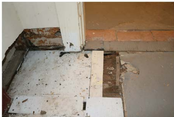
2 Numerous layers of plywood have been installed where excessive water damage has occurred.
