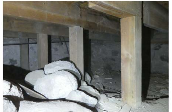
5 Secondary supports placed under the floor joists where the floor has been modified.
