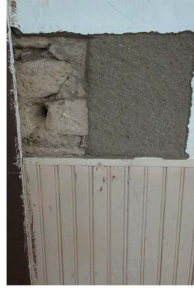
3 A previous investigation by Cornerstones Community Partnerships, 2008, reveals layers of construction.
