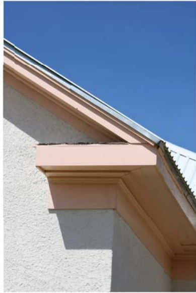
2 Remnants of original wood shingles still exist at soffit returns
