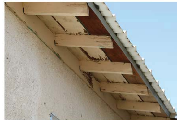
1 Rafter tails are deteriorated and exposed roof deck boards have been replaced.
