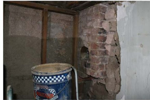
2 Brick chimney for flu was constructed at top of adobe wall which was dismantled and replaced with stud wall. Chimney no longer penetrates roof.
