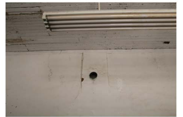
5 The bulge in the wall defines the location of the brick chimney constructed in the adobe wall and now dismantled at top of wall. Borings were done to verify location of brick to adobe construction.
