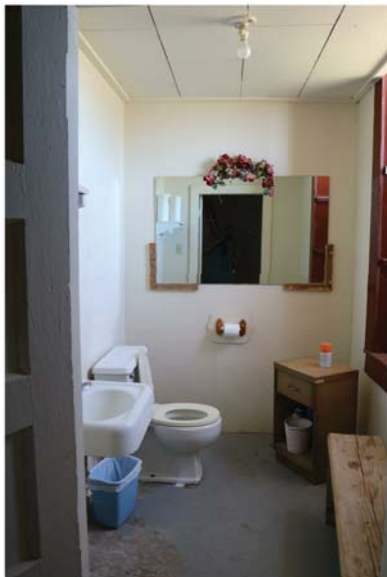
4 The toilet room floors are concrete.
