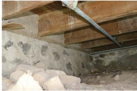
1 Rubble foundation wall with adobe blocking in-between support joists.
