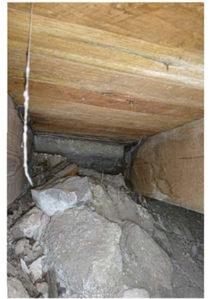
4 A concrete slab has been poured on top of the demolished rubble foundation at restrooms.
