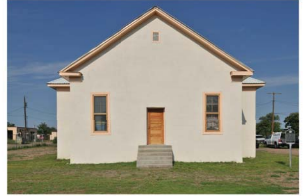
5 East elevation has been modified from original arch entry.
