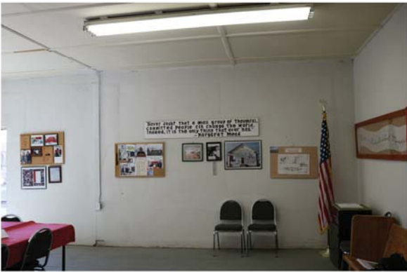
4 Five windows were previously blocked. The ghost of the openings is visible.
