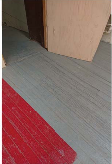
5 The original threshold has been removed and replaced with concrete as a transition to the concrete ramp to the band hall.
