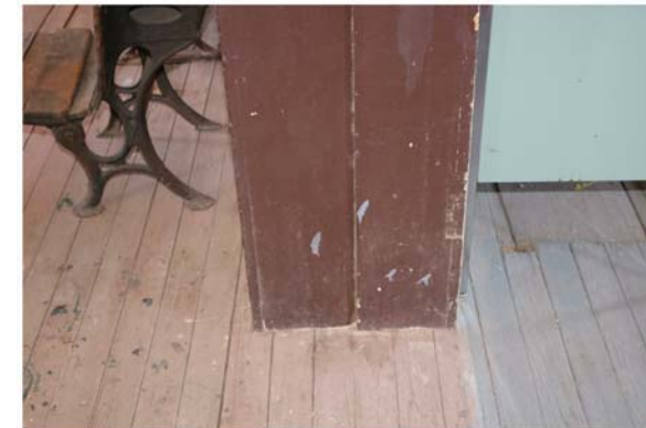
3 crawl space access panels have been cut on both sides of the center adobe wall.
