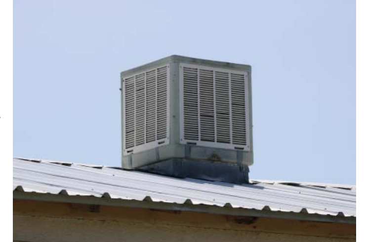
Remove rooftop swamp cooler.
