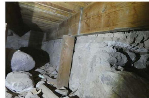
6 Secondary support has been placed under the floor joist which is positioned adjacent to the rubble foundation wall.
