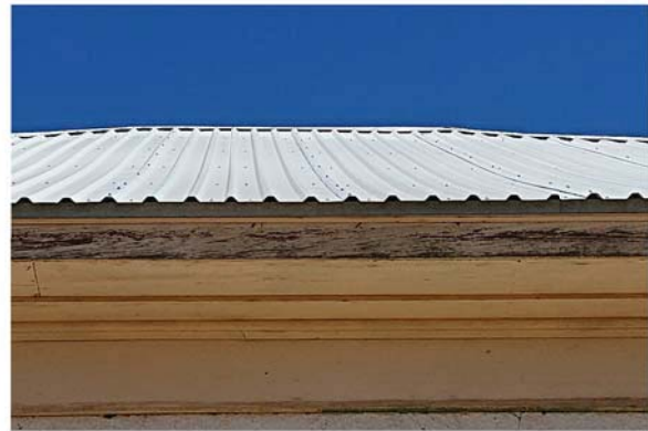
1 Ridge is out of true and sloped plane bows downward.
