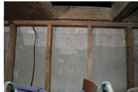
3 Non-original wood stud wall with expanded metal lath and cement plaster comprises the west wall of the boys restroom.
