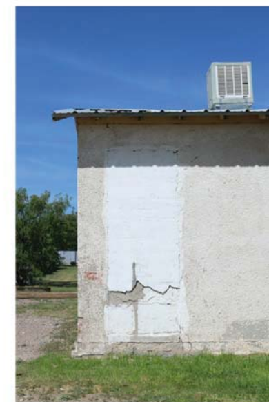
4 Cracked Stucco reveals location of previously in-filled doorway.
