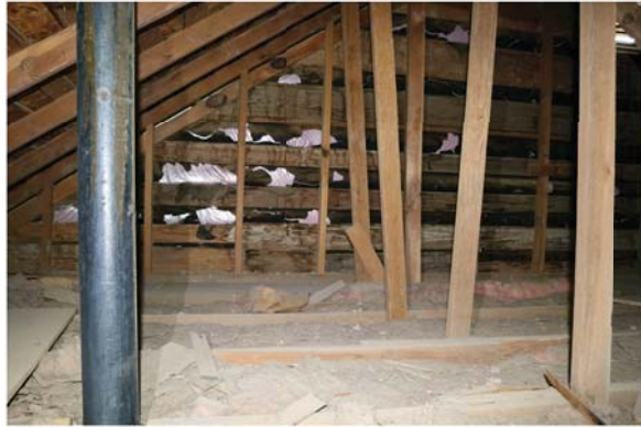
2 Wood structure at interior face of gable.
