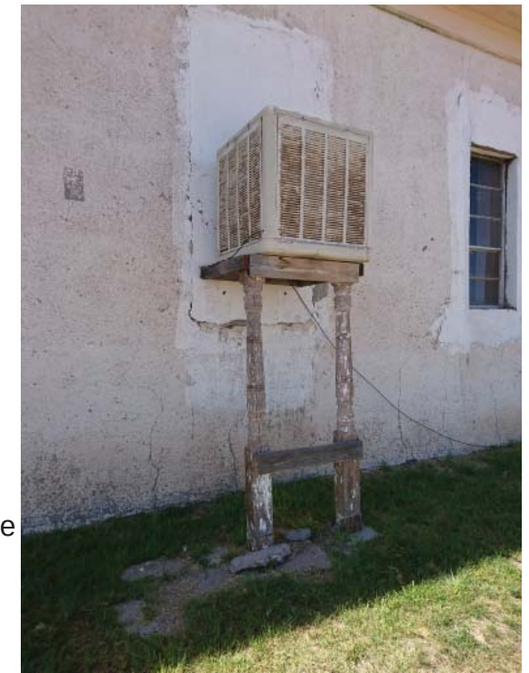
Remove existing swamp cooler, restore window opening.
