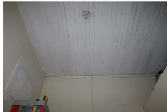
4 The beaded board tongue-and-groove ceiling boards in the vestibule area run East / West the full width of the interior space.
