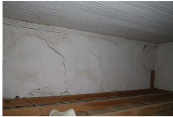
1 South wall above dropped ceiling at office area. Wall shows numerous cracks not seen below the ceiling due to the installation of paneling on lower portion of wall.
