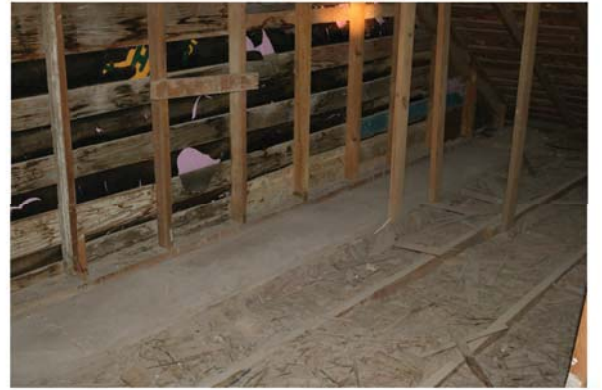
4 A reinforced concrete beam was installed along the top portion of the adobe wall on the east façade at the gable.
