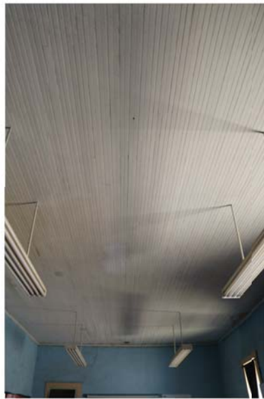
2 The beaded board tongue-and-groove ceiling boards are in relatively good condition in this area.
