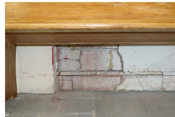
6 Brick chimney abuts structural clay tile wall. a wood nailer indicated a wood baseboard was previously installed.
