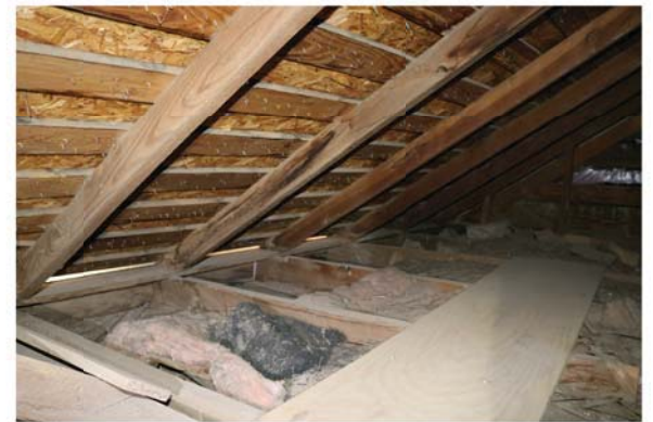
6 Spaced sheathing used for wood shingles is covered with oriented strand board, presumably installed at time of metal roof.
