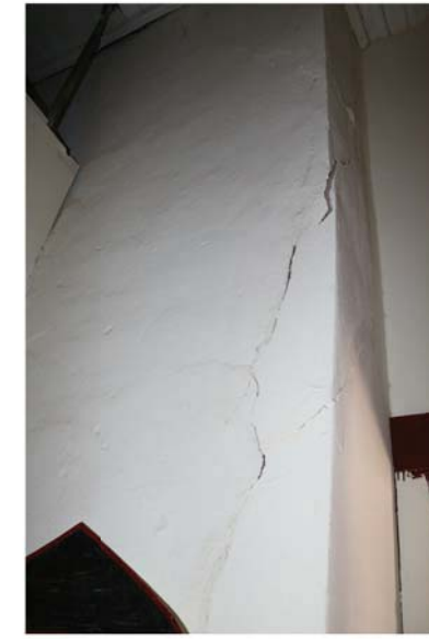
6-A This corner was created when the adobe wall was removed for the construction of the stud wall. Plaster was badly cracked and loose. Plaster was not installed on metal lath on this wall.
