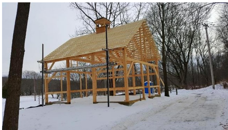
The replica barn at the Kelly House under construction this January.
