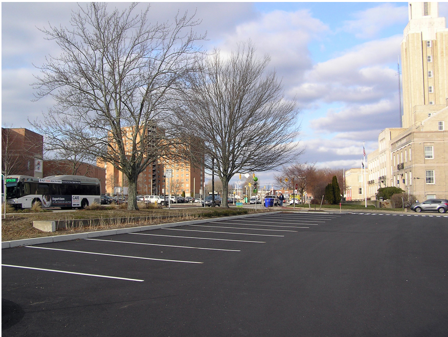
Figure 32. View looking north at a portion of the parking lot concrete retaining wall in the North Lot. The entrance to the lot is in the background at image right. (OCLP 2021, P1010001)
