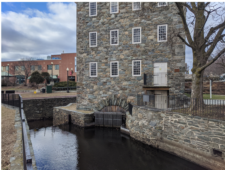
Figure 41. View looking northwest at part of the restored Great Flume as it enters the Wilkinson Mill. (OCLP 2020, IMG-20200105-120440)
