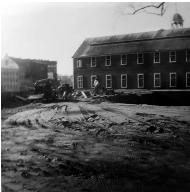
Figure 17. View looking southwest at construction of the boiler house on the former peninsula, 1954. (OSMA Archives, from HSR 2018: D-109)
