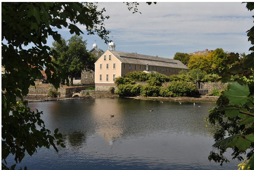
Figure 25. View looking west at the Slater Lot, 2019. The Old Slater Mill's stone foundation, stone retaining walls, and earthen banks define the river edge. (OCLP 2019, DSC-5478)
