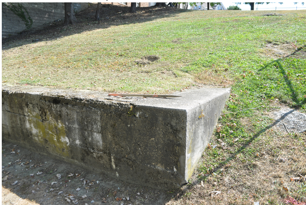
Figure 36. View looking southeast at part of the remnant foundation wall in the East Lot. (OCLP 2019, DSC-5338)
