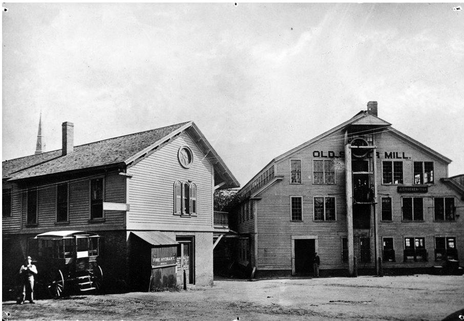
Figure 10. View looking south at the north and east sides of Old Slater Mill, c.1886. This is the first view showing the second and third story west addition and the rope pulley elevator. Note the fence that once bordered Slater Avenue is gone. (OSMA Archives, from HAER RI-1, 1991)
