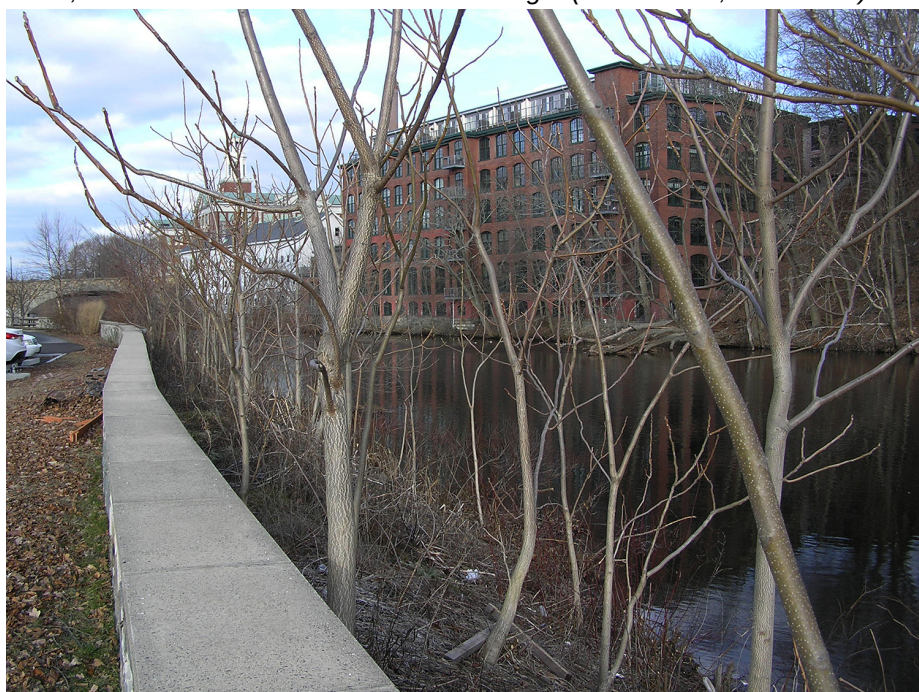
Figure 26. View looking north at invasive trees close to the stone retaining wall in the North Lot. (OCLP 2021, P1010007)
