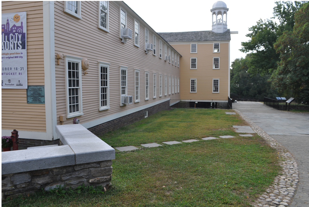
Figure 29. View looking southeast at the west side of Old Slater Mill. Note the retaining wall, steeping stone path, and two concrete pads that once supported benches. (OCLP 2019, DSC-5351)
