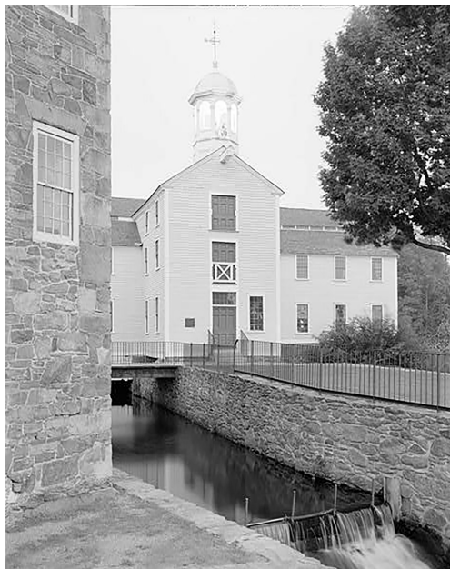
Figure 23. View looking east at the extension of the Great Flume and the small dam, 1991, around ten years after it was built. (Photograph by Joseph E.B. Elliott, HAER RI-1, 1991)
