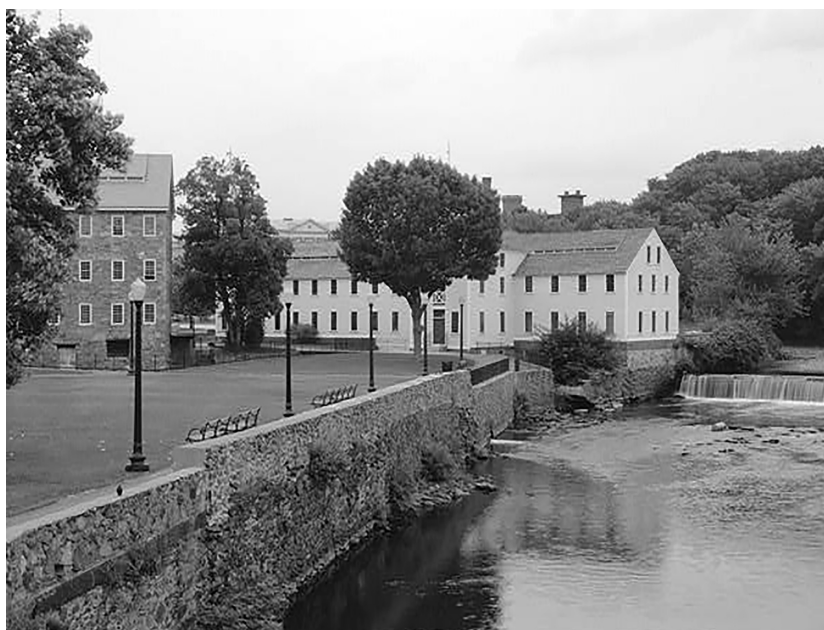
Figure 24. View looking northeast, 1991. Note the height of the river wall/old foundation blocks. In c.2016 the highest part of the wall was lowered and the benches were reoriented to the river. (Photograph by Joseph E.B. Elliott, HAER RI-1, 1991)
