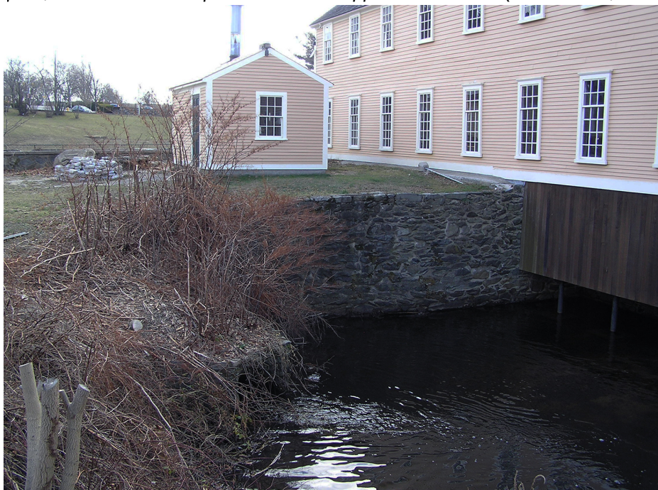
Figure 30. View looking southeast at woody vegetation in the Great Flume, the outlet of the penstock pipe, and the boiler house on top of the former island peninsula. (OCLP 2021, P1010020)
