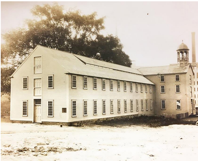
Figure 16. View looking east at the north and west sides of Old Slater Mill, c.1925, after the building's restoration but before landscaping was completed. (OSMA Archives, from HSR 2018: D-86)
