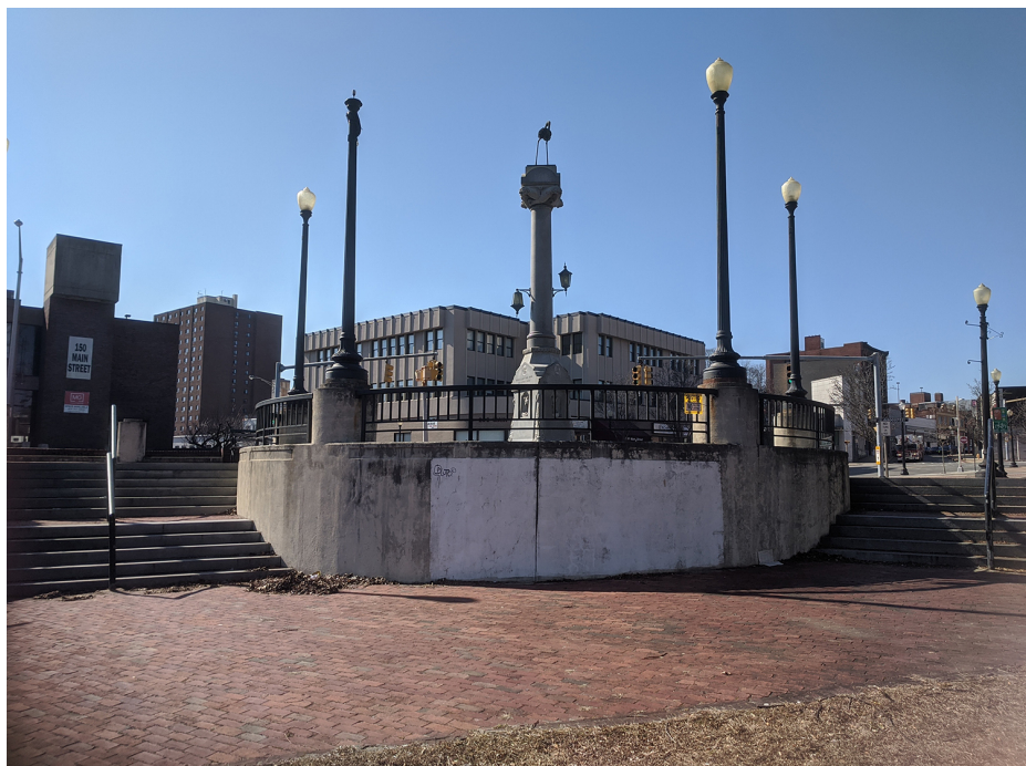
Figure 35. View looking west at the concrete retaining walls and steps at the Cogswell Monument. (OCLP 2020, IMG-20200223-130908)
