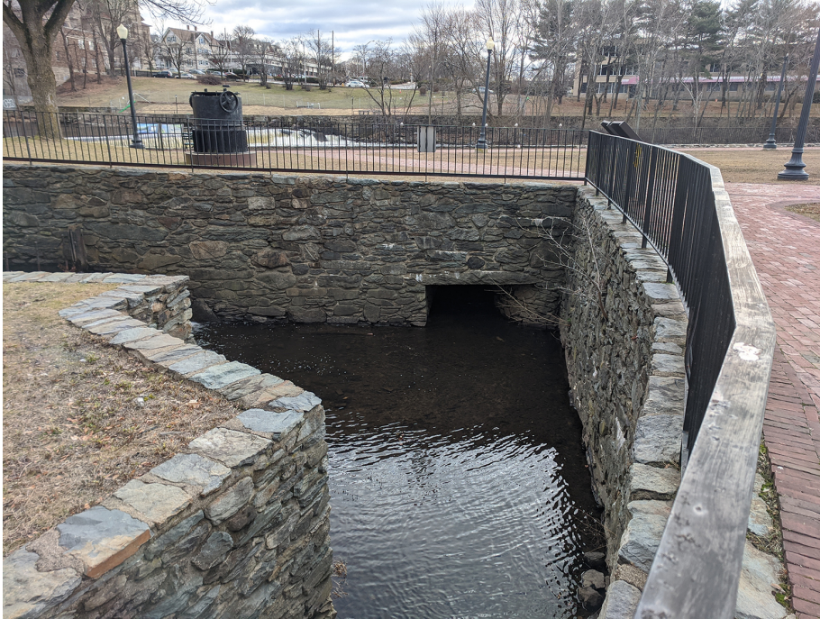
Figure 42. View looking southeast at the pipe inlet that carries water from the Great Flume and the Wilkinson Mill tailrace back to the river. (OCLP 2020, IMG-20200105-120816)
