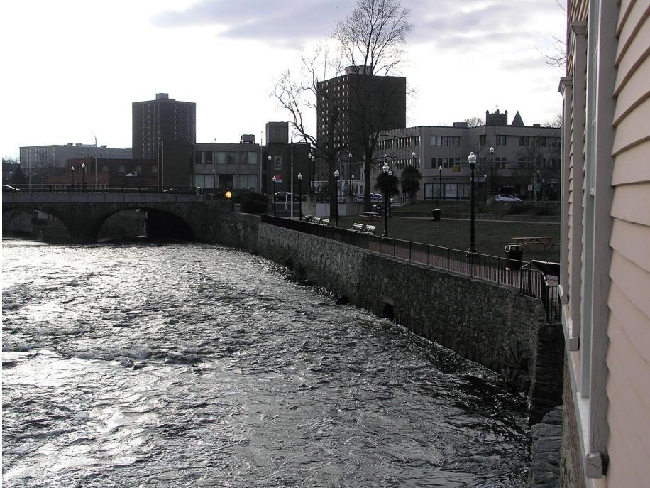
Figure 27. View looking southwest at the stone river wall / foundation walls that define the river's edge in the South Lot. (OCLP 2021, P1010011)
