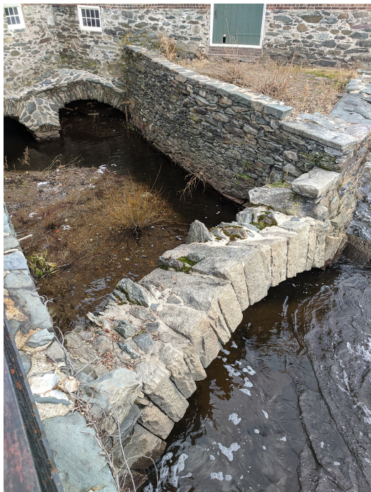
Figure 40. View of the tailrace stone walls and stone arch. (OCLP 2020, IMG-20200105-121104)
