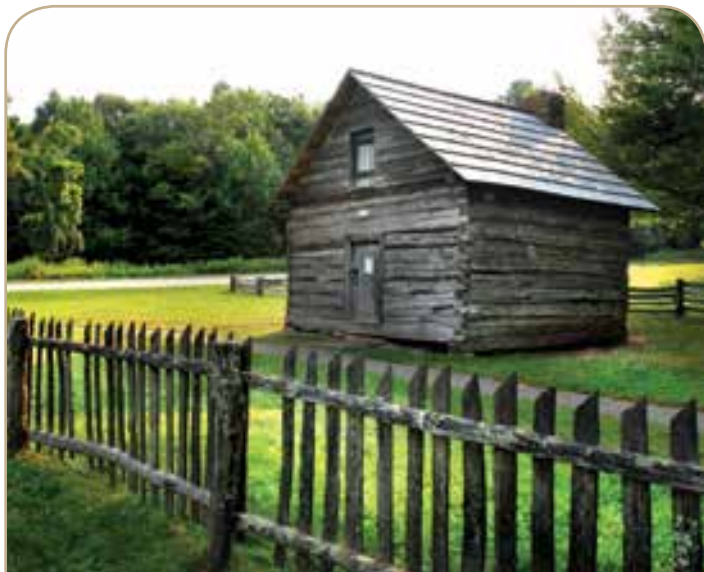
Puckett Cabin | Milepost 189.9
