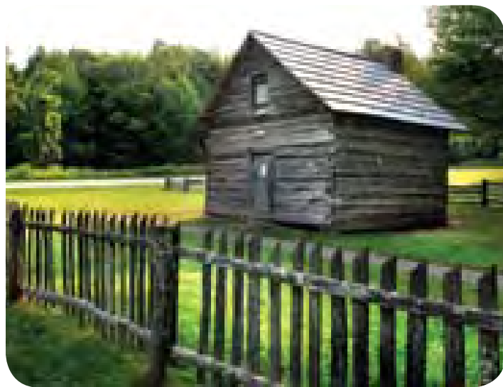
Puckett Cabin 1 Milepost 189.9
