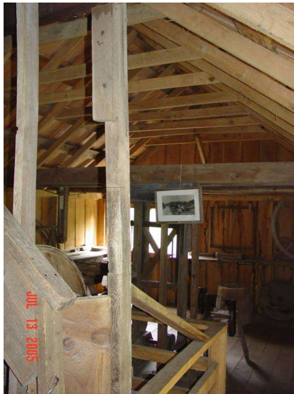
Viewing the woodworking shop standing near stairs in the loft section of the grist mill section of Mabry Mill.
