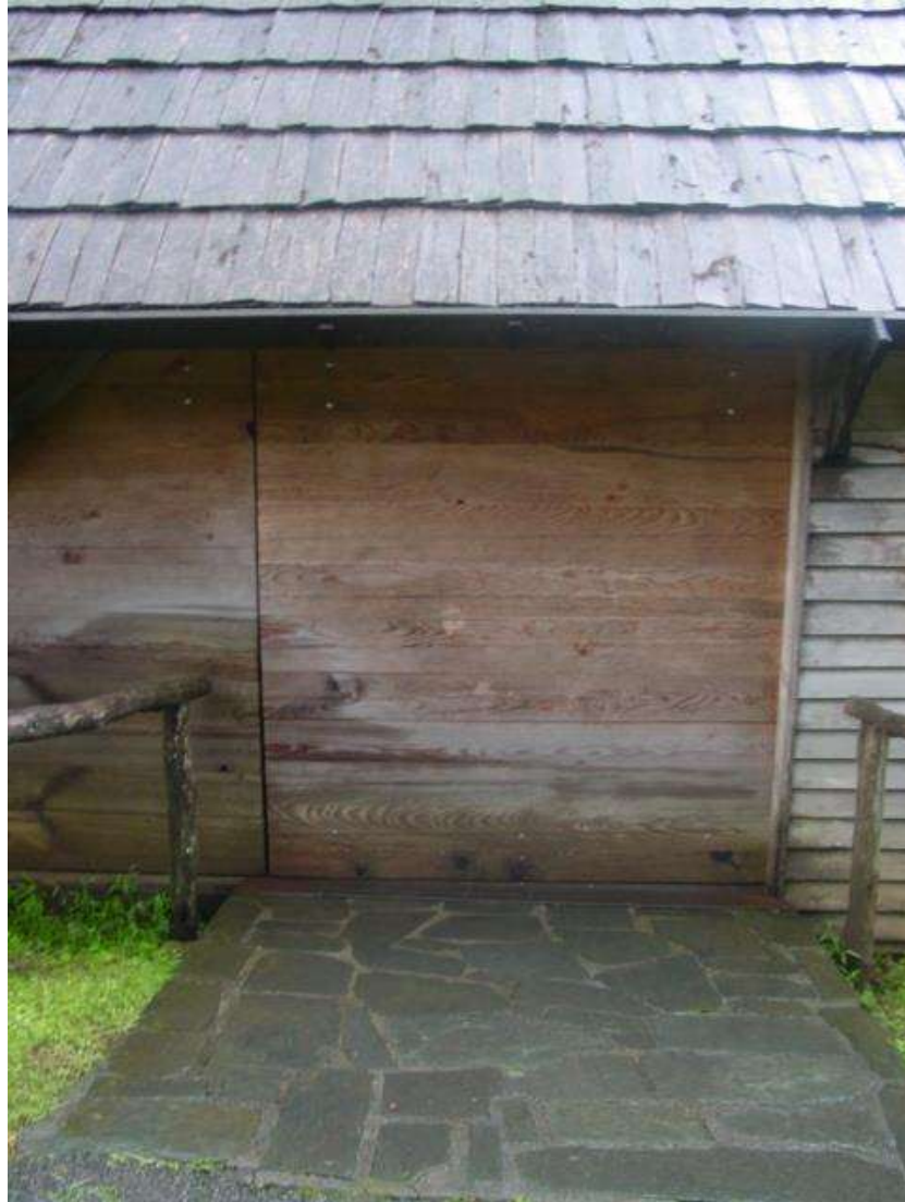
Viewing closed mill looking at sawmill section door and handicap paved walkway. This door is larger in order to comply with the materials used for the sawmill.
