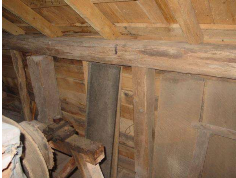
West wall in the upper loft section of the mill.
