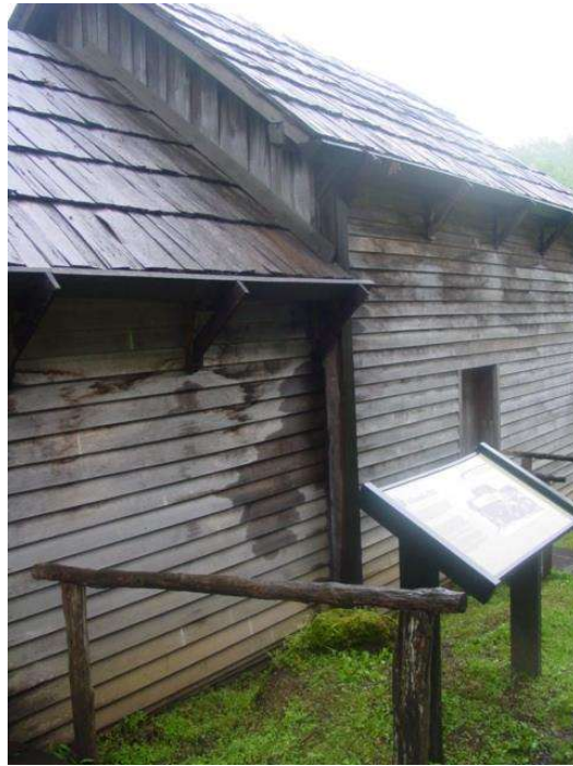
Viewing west elevation; note the information sign in front of the façade and handicap hand railing.
