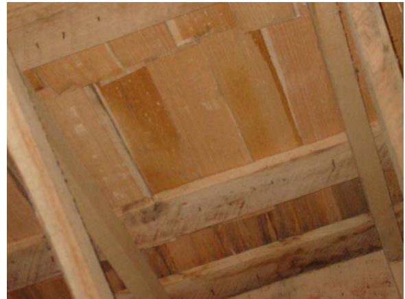
East elevation in the upper loft of the mill section of the structure.
