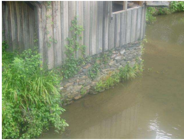
Stone foundation on the south elevation.
