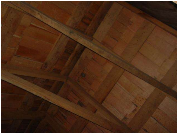
Ceiling in the loft section of the mill section of Mabry Mill. This photo shows the structure in the ceiling.
