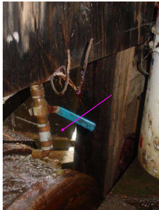
Hose that comes from the flume to the east elevation to the case opening for the wheel axle.
