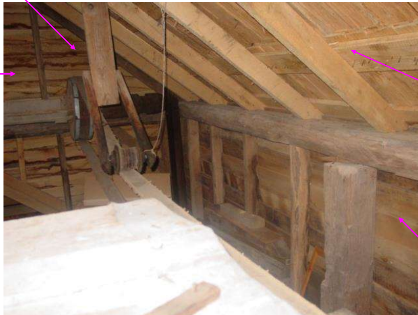
Ceiling and rafters
