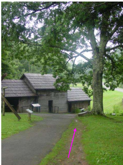
This is a diagram showing the path of the water that leads to erosion on the west elevation looking towards the woodworking shop entrance of Mabry Mill.
