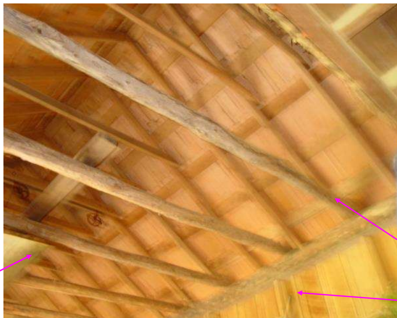
This is the ceiling in the saw mill section of Mabry Mill. View is from standing near the gristmill section of the mill facing the north interior wall, looking up.
