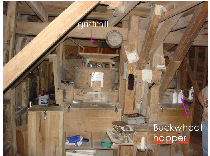
Gristmill: viewing from standing in the sawmill section looking towards the mill, the south interior wall, and the woodworking shop.
