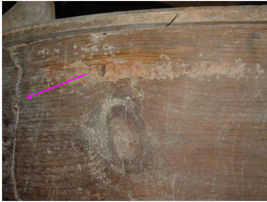
Cracks in buckwheat stone cover.
