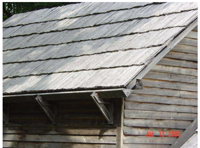
Viewing the roof shakes on the west elevation of the mill section of Mabry Mill.
