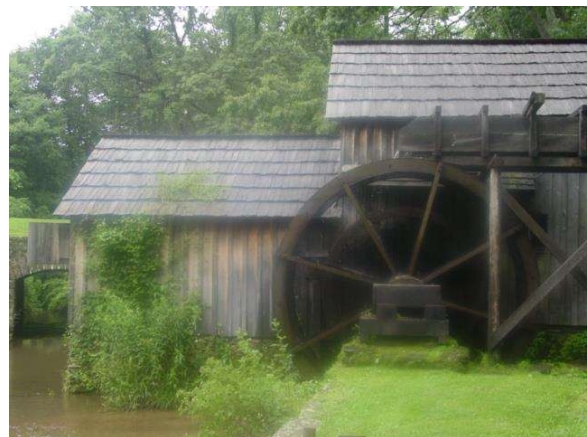
East Elevation; note the overgrown vegetation on the exterior.
