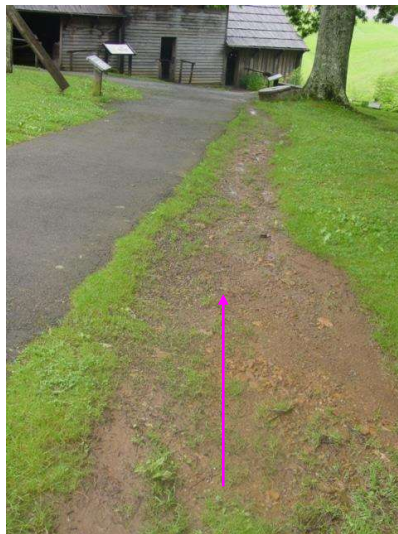
This is a diagram showing the path of the water that leads to erosion on the west elevation looking towards the woodworking shop entrance of Mabry Mill.
