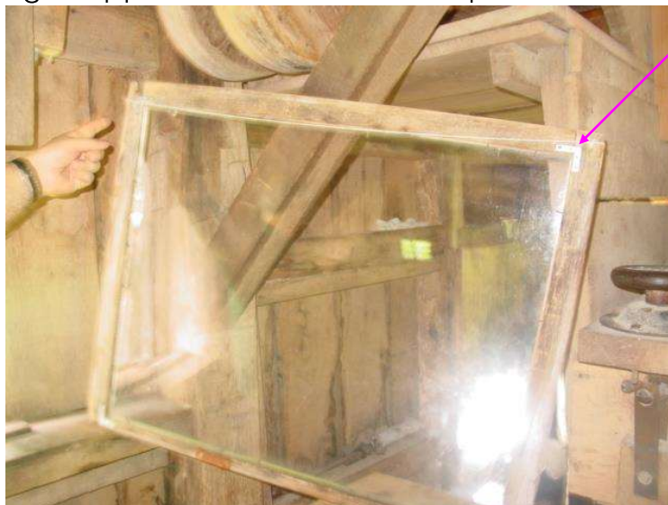
Window [sash] to the mill on the east elevation of the mill section.
