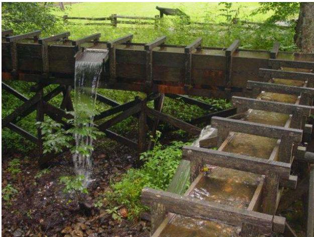
Viewing from the top of the flume, standing on the wooden handicap bridge/walkway; note that there are 2 overflow sections; mill is off to the left.
