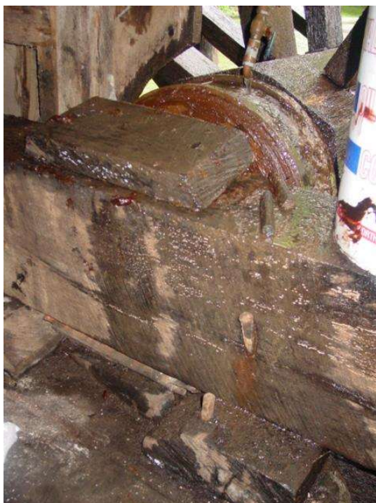
Viewing the wet axle, case opening and interior on the east wall of the interior.
