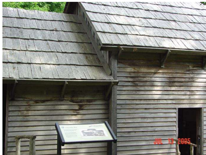
Viewing the connection on the west elevation of the sawmill shop and the gristmill shop.
