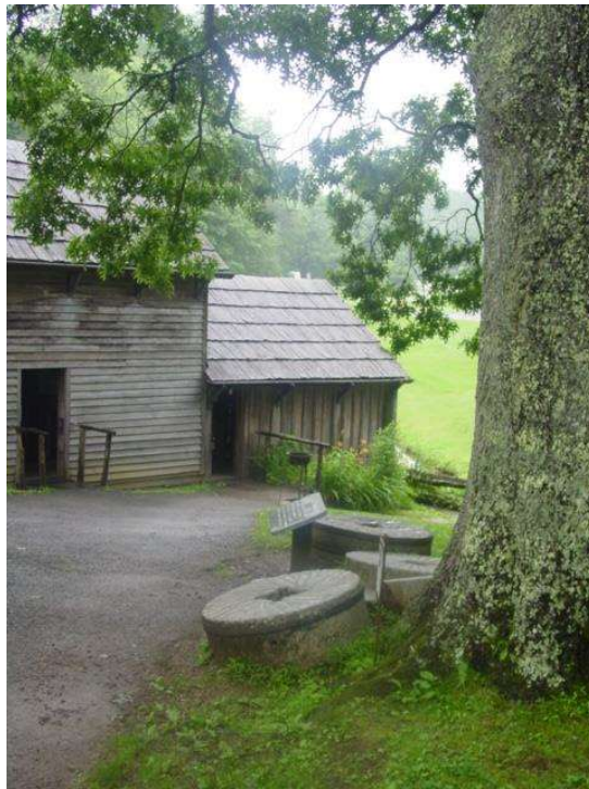
Old mill stones in front of the west elevation of the building.
