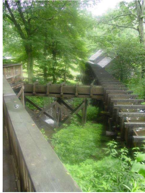
Connection of the flume and race looking south.
