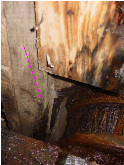
Water damage from splashes from water wheel through the case opening for the axle.
