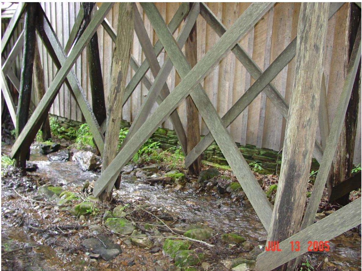
Water stream under the flume.
