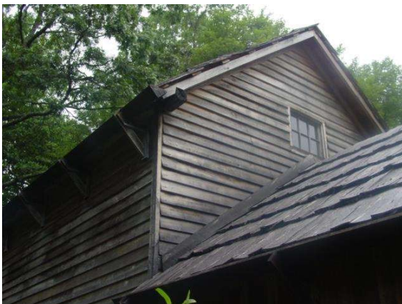
Exterior of upper loft of the mill section; southwest perspective.
