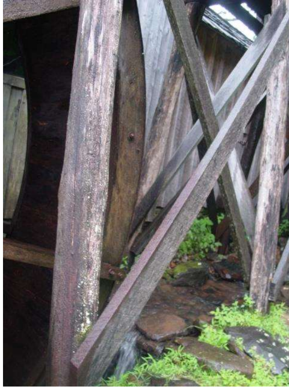
Flume structure, [which sits on underground concrete piers.
