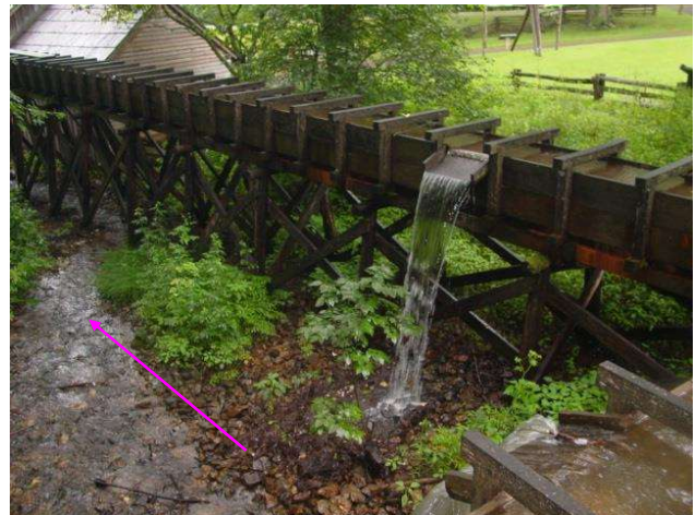
Water from the overflow goes under the flume and into the pond [near the east elevation].
