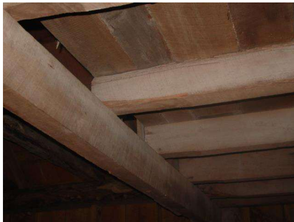
There are grooves in the wood in order for them to rest on the beams.
