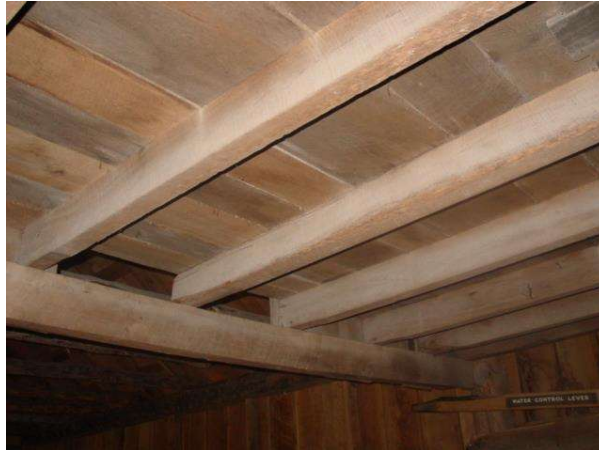
Ceiling structure in the gristmill section of the mill; this wood is original.
