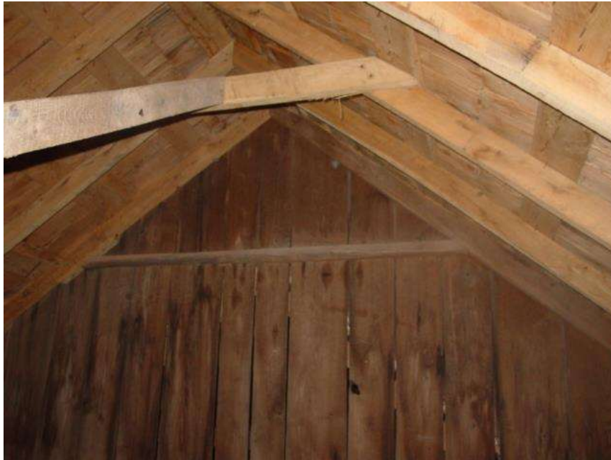
Ceiling in the upper loft section of the grist mill section in Mabry Mill; this photo shows roof structure.
