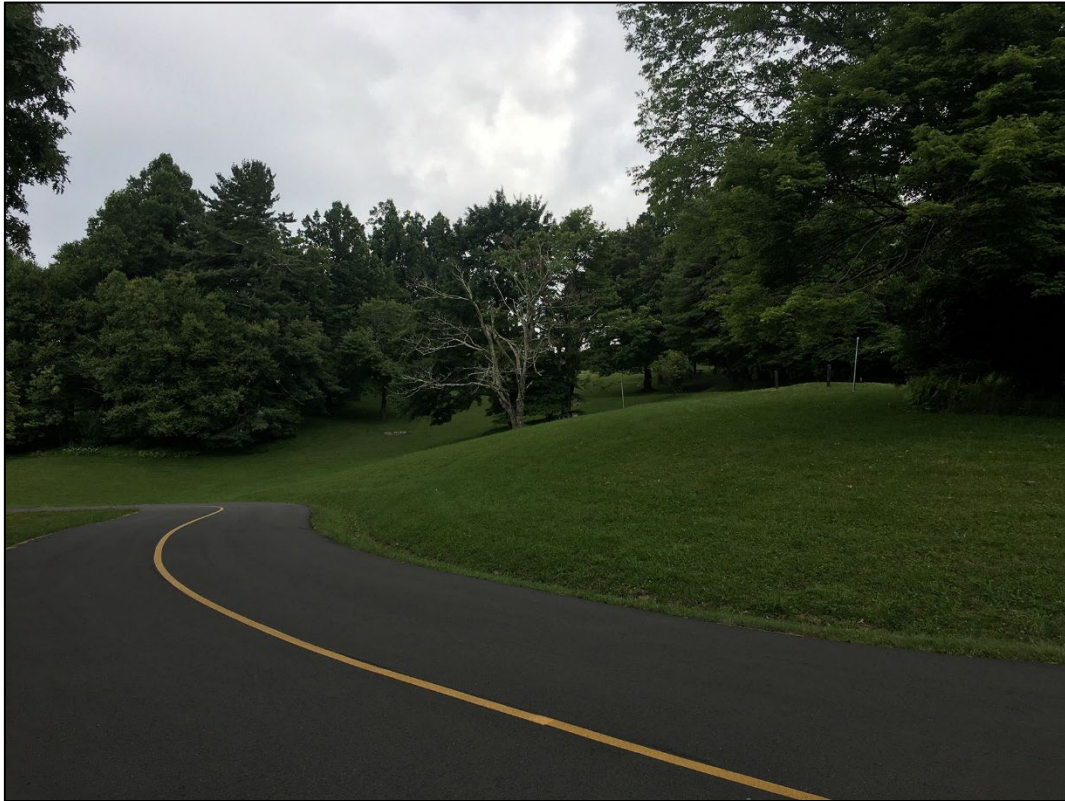
Fig 8-11. Outer Loop A road in good condition with new paving and fresh paint. Camera facing southeast (2021)
