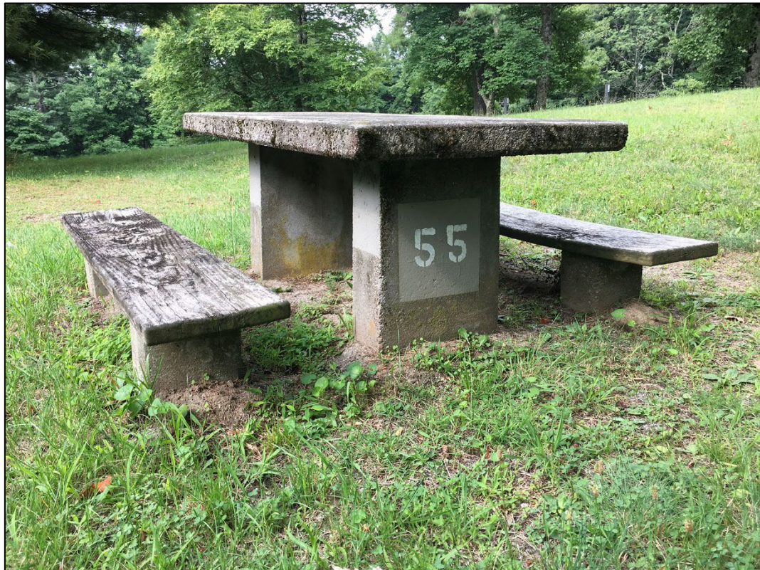
Fig 8-28. Example of Mission 66 Era picnic table. Mission 66 Modern style, concrete block construction (2021)
