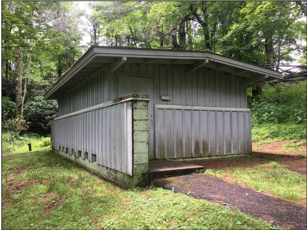
Fig 8-19. Oblique view of Comfort Station #370, north façade. Camera facing southeast (2021)
