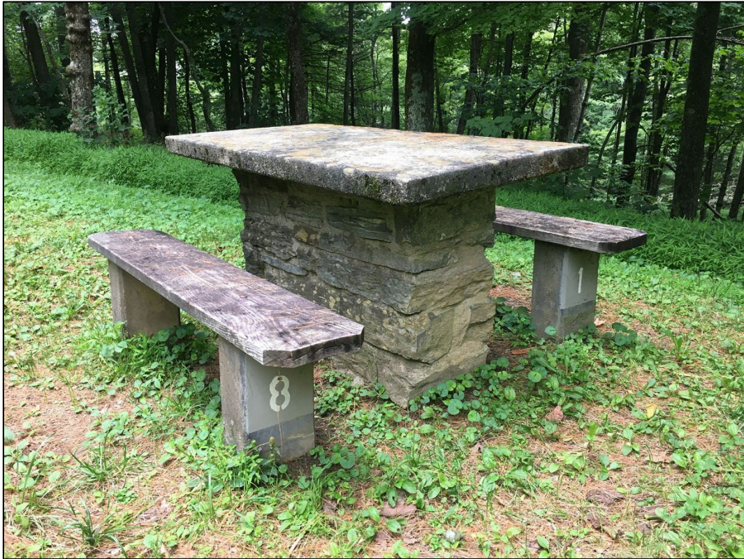
Fig 8-25. Example of Prewar Planning and Construction Era picnic table. Park Rustic style with concrete block replacement piers (2021)
