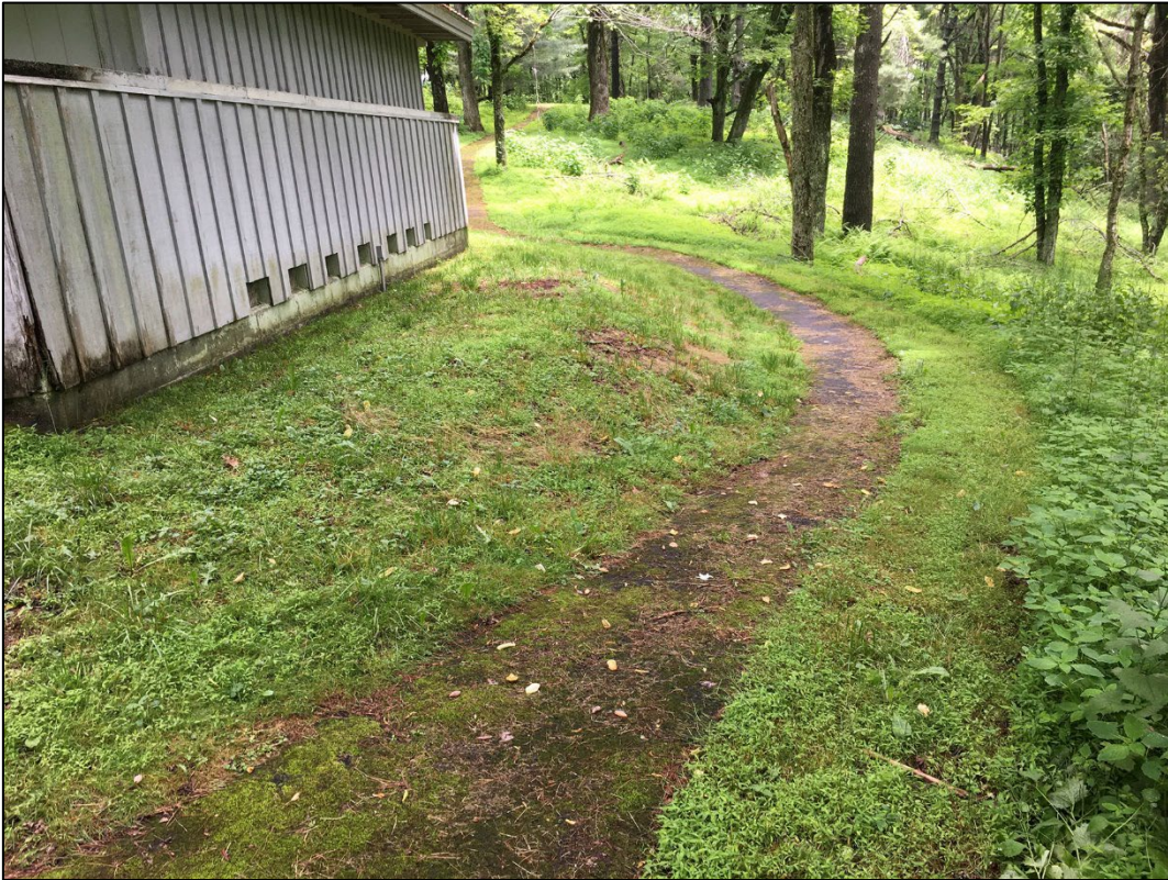
Fig 8-9. Paved asphalt pathway near Comfort Station #370. Moderate moss growth. Camera facing northwest (2021)
