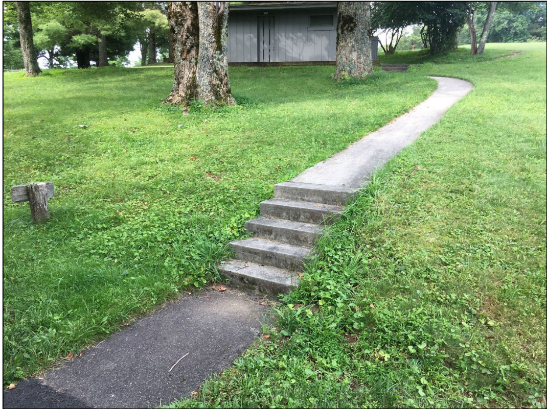
Fig 8-4. Concrete steps near Comfort Station #396. Camera facing southwest (2021)
