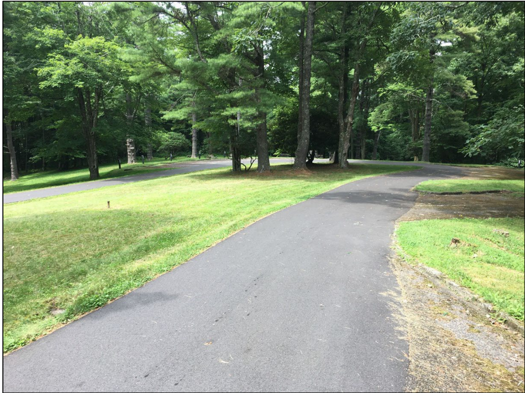
Fig 8-14. Loop D road in good condition, example #2. Camera facing north (2021)
