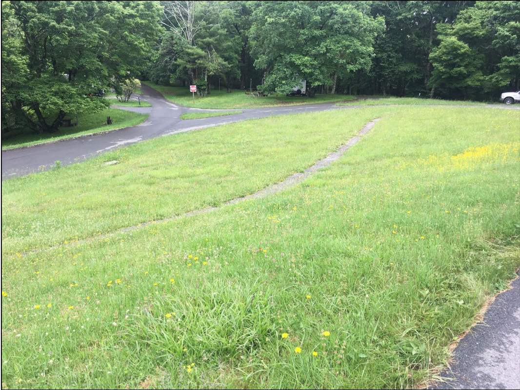
Fig 8-7. Paved asphalt pathway near Loop C (Trailer Campground). Camera facing south (2021)
