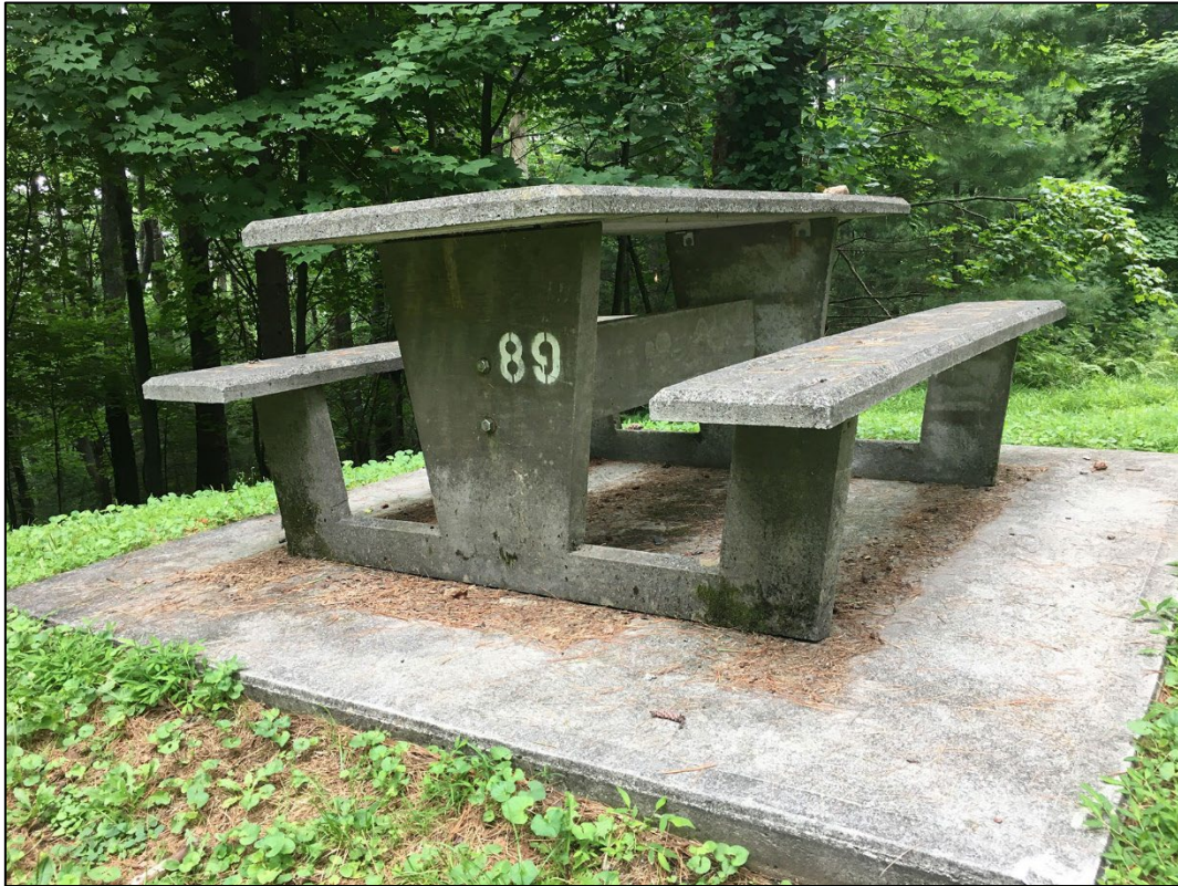
Fig 8-27. Example of Mission 66 Era picnic table. Mission 66 Modern style (Type II), precast concrete construction (2021)
