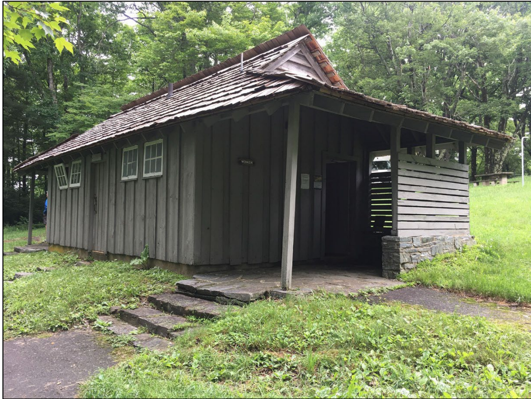
Fig 8-17. Oblique view of Comfort Station #97, south façade. Camera facing northwest (2021)
