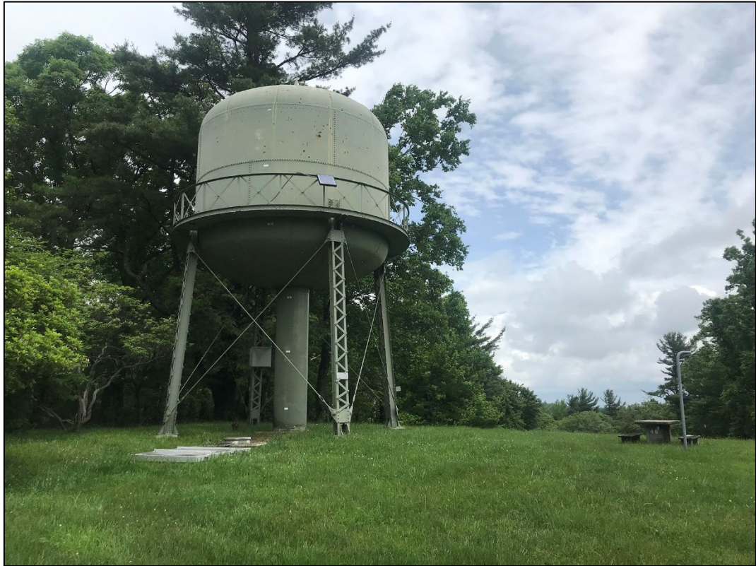
Fig 8-21. Oblique view of c. 1939 water tank. Camera facing northeast (2021)
