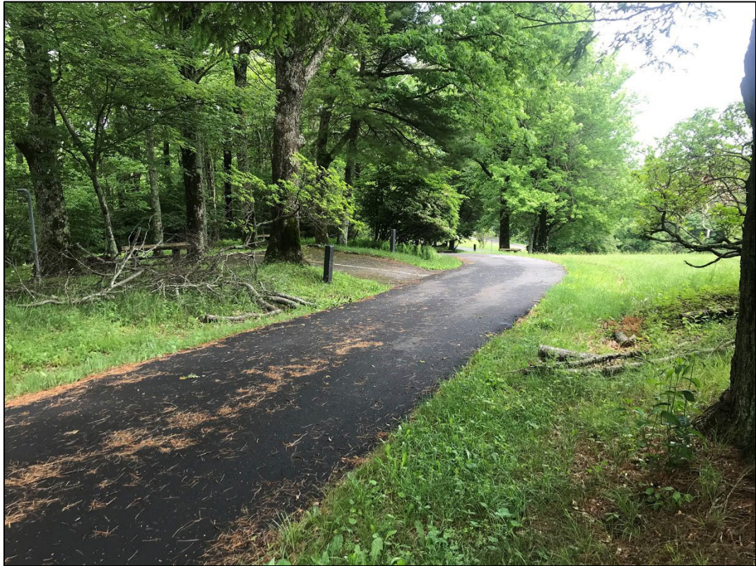
Fig 8-10. Inner Loop A entry road. Camera facing north (2021)
