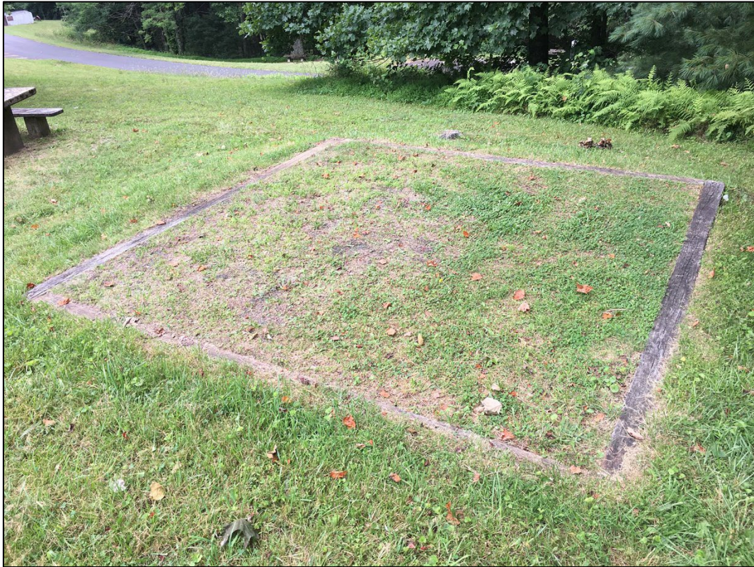
Fig 8-33. Tent pad lined with buried wood ties along Inner Loop A. Camera facing northeast (2021)
