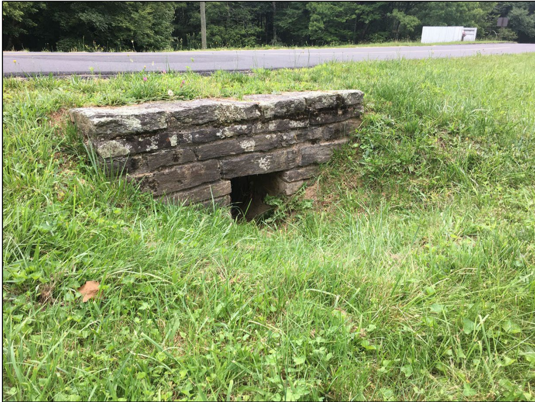
Fig 8-31. Stone headwall near Outer Loop A. Camera facing northeast (2021)
