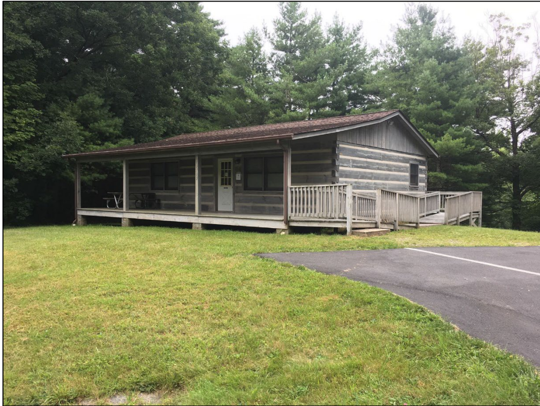
Fig 8-23. Oblique view of Host Cabin, north façade. Camera facing southeast (2021)
