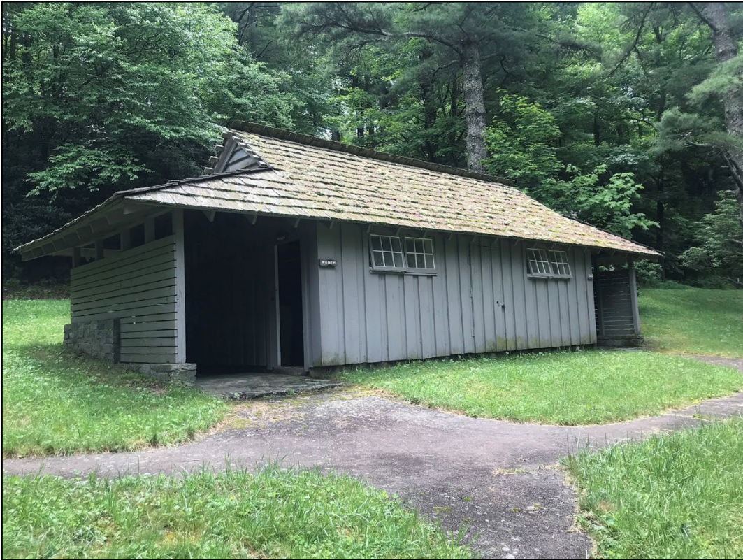
Fig 8-18. Oblique view of Comfort Station #98, west façade. Camera facing southeast (2021)
