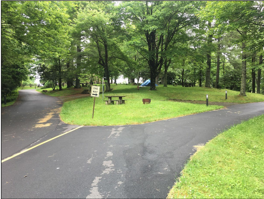
Fig 8-15. Fork in Loop E road. Road in good condition. Camera facing northeast (2021)
