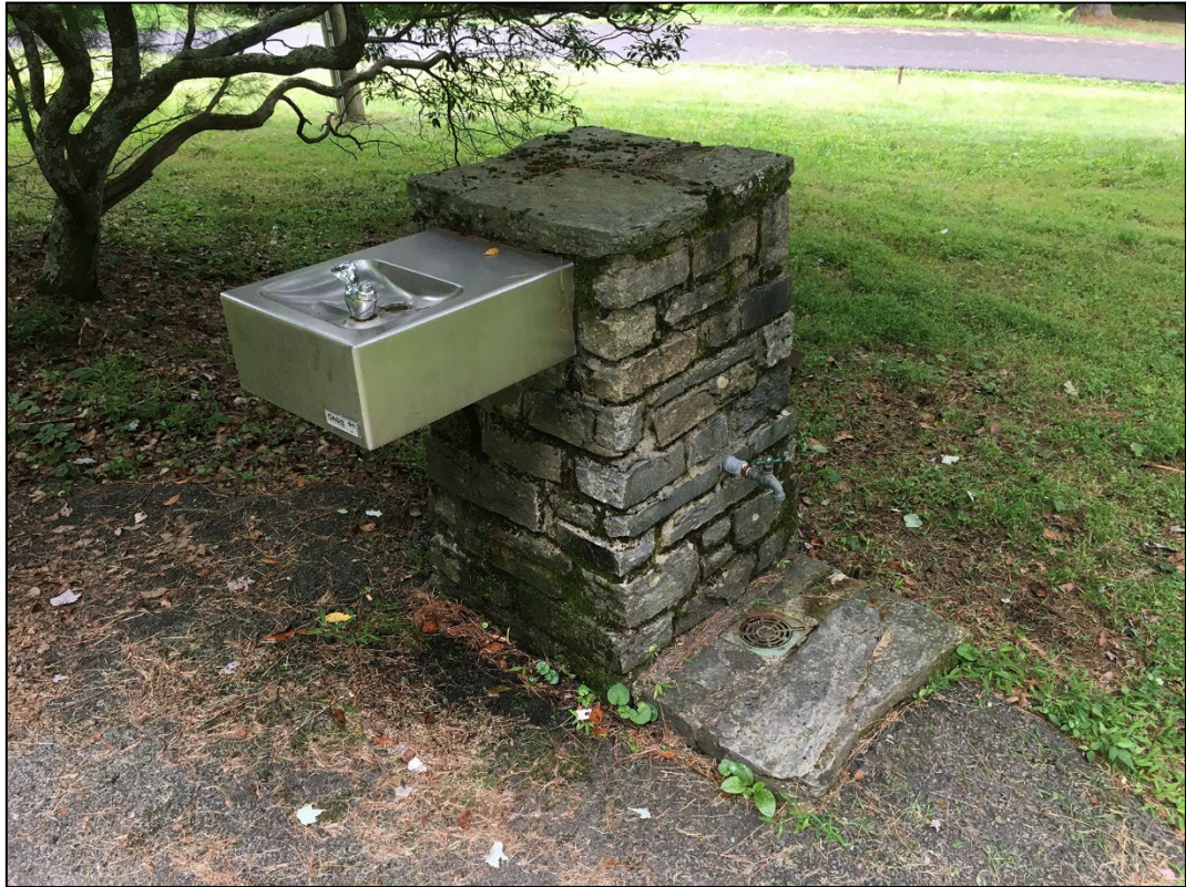
Fig 8-30. Stone drinking fountain with contemporary stainless-steel spigot near Loop D. Camera facing west (2021)
