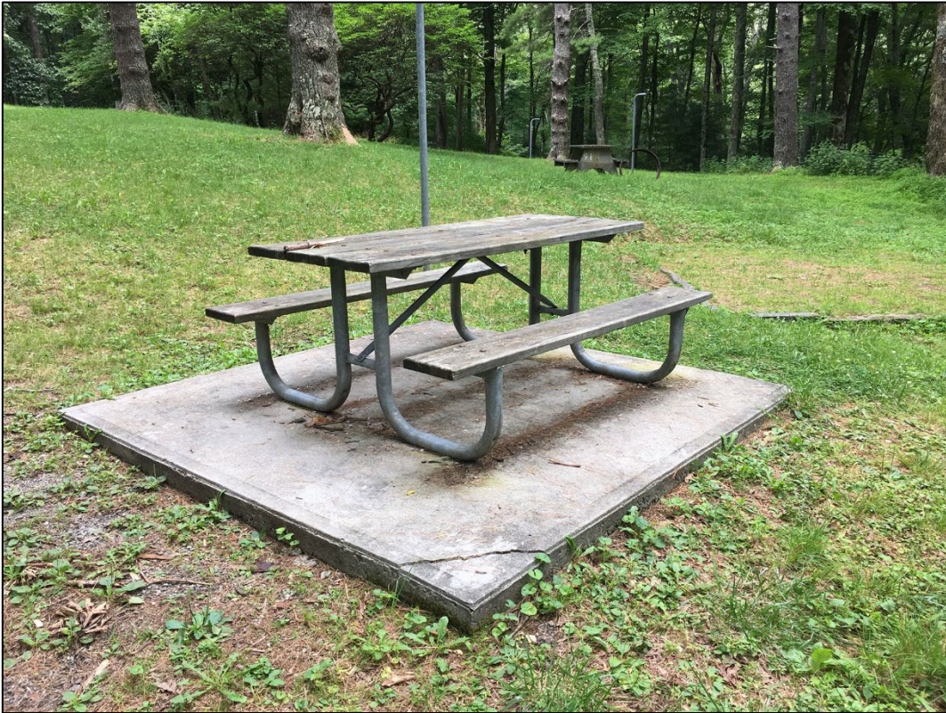
Fig 8-29. Example of Post-Mission 66 Era picnic table. Contemporary style, prefabricated steel construction (2021)
