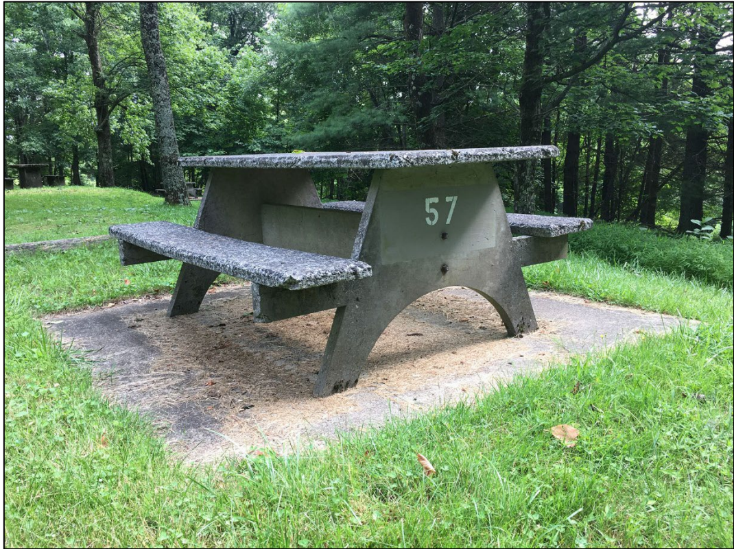
Fig 8-26. Example of Mission 66 Era picnic table\ Mission 66 Modern style (Type I), precast concrete construction (2021)
