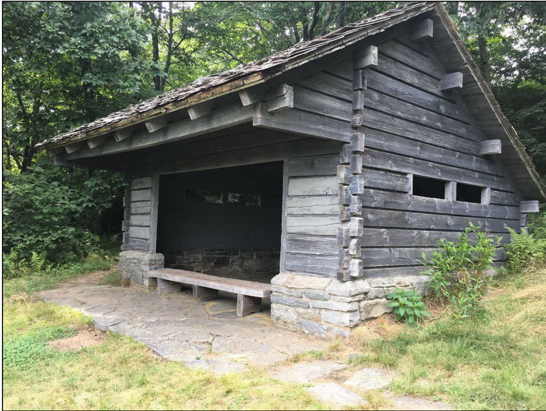
Fig 8-14. Oblique view of Bluff Ridge Shelter (2021)
