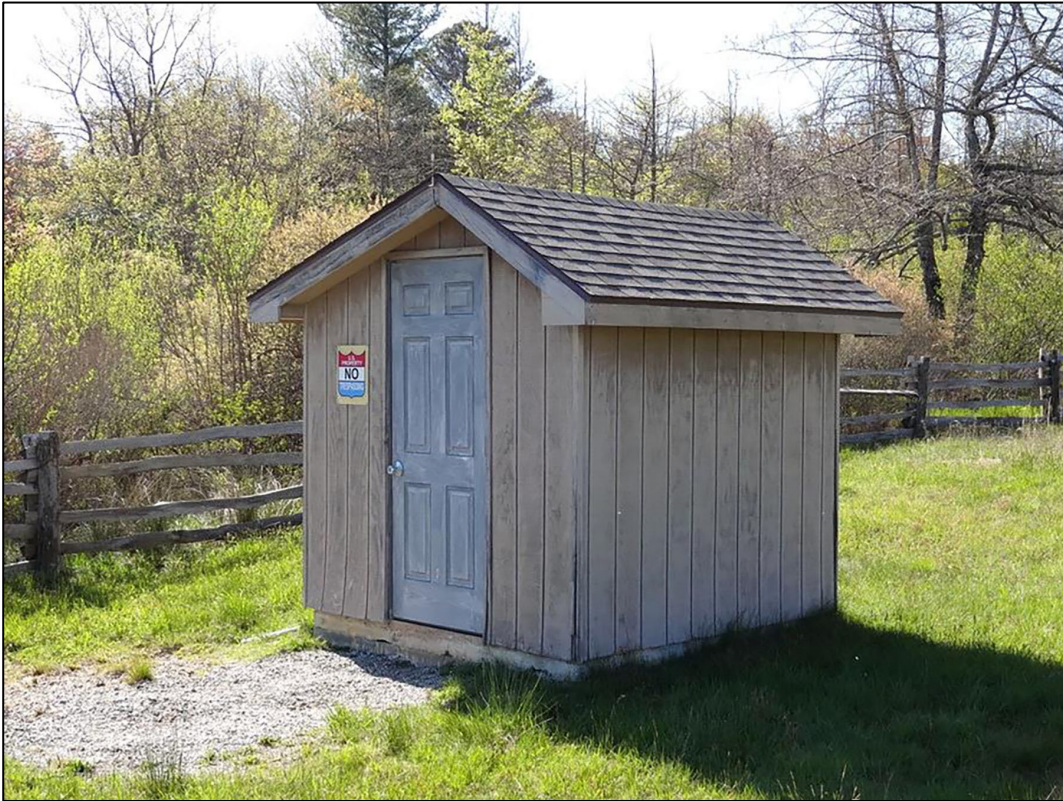
Fig 8-12. Cotemporary Pump House (2013)
