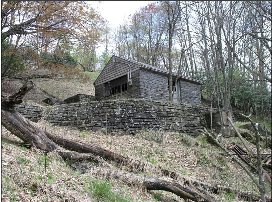
Fig 8-13. Fodder Stack Pump House (2013)
