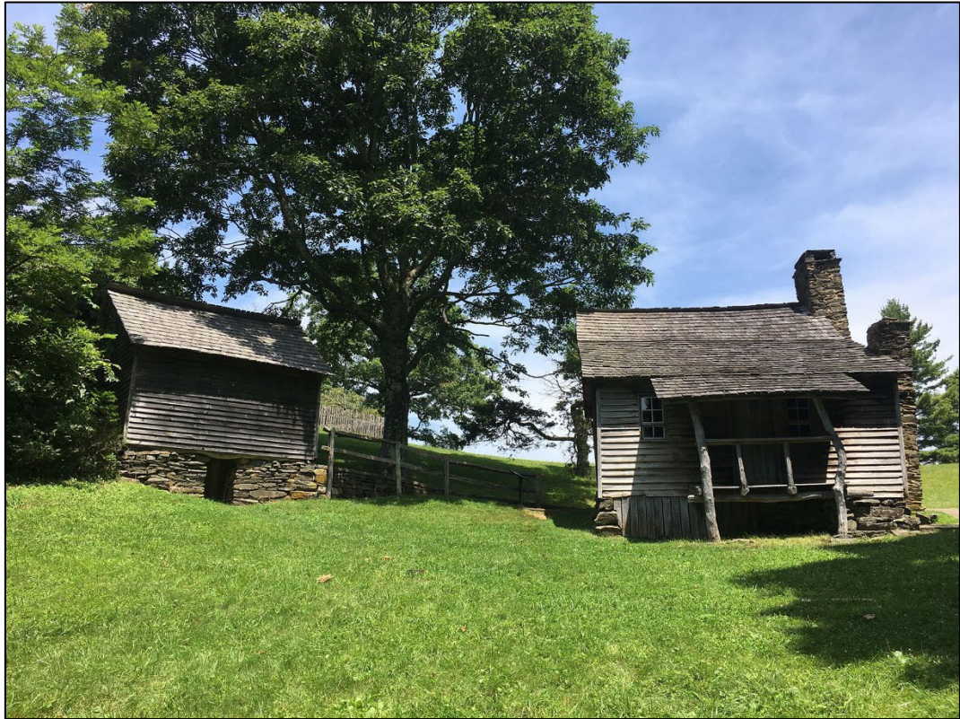
Fig 8-4. View of Brinegar Cabin and Shed illustrating spatial organization of original farmstead (2021)
