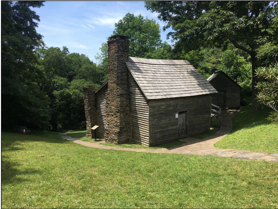
Fig 8-20. Brinegar Cabin, north façade (2021)
