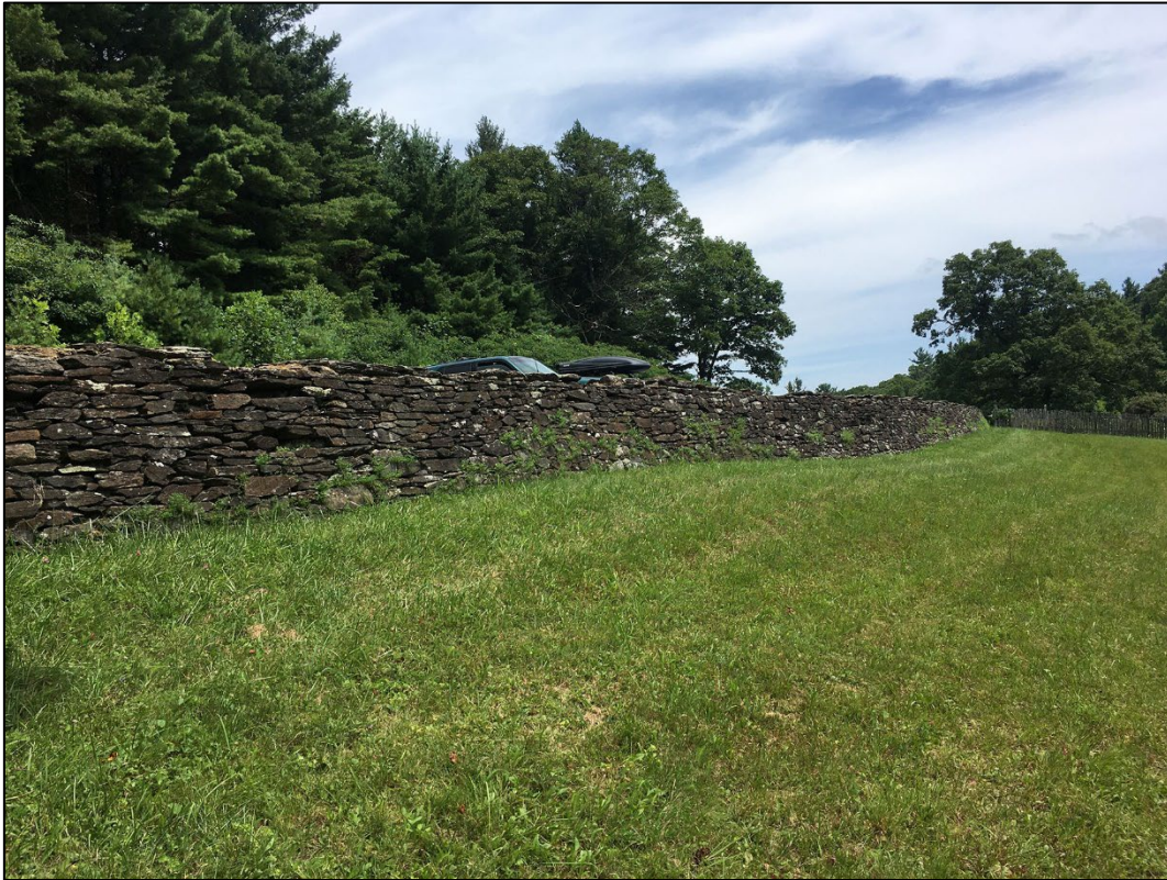
Fig 8-27. View of stone retaining wall from orchard site. Elevation view, facing northwest. (2021)
