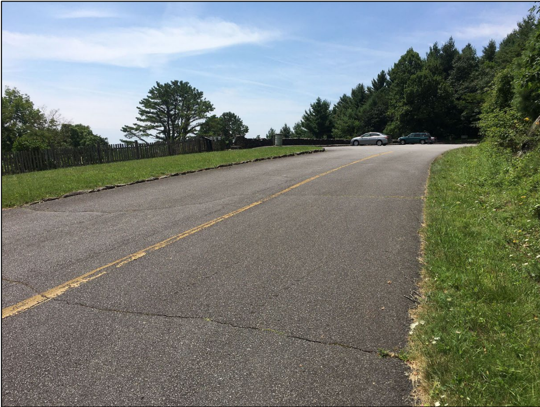
Fig 8-10. Brinegar Cabin entry road, view toward parking lot (2021)
