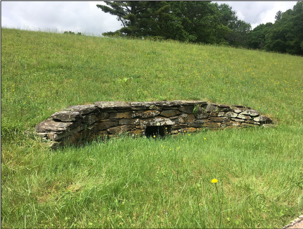
Fig 8-26. Stone tailwall at Brinegar Cabin (2021)
