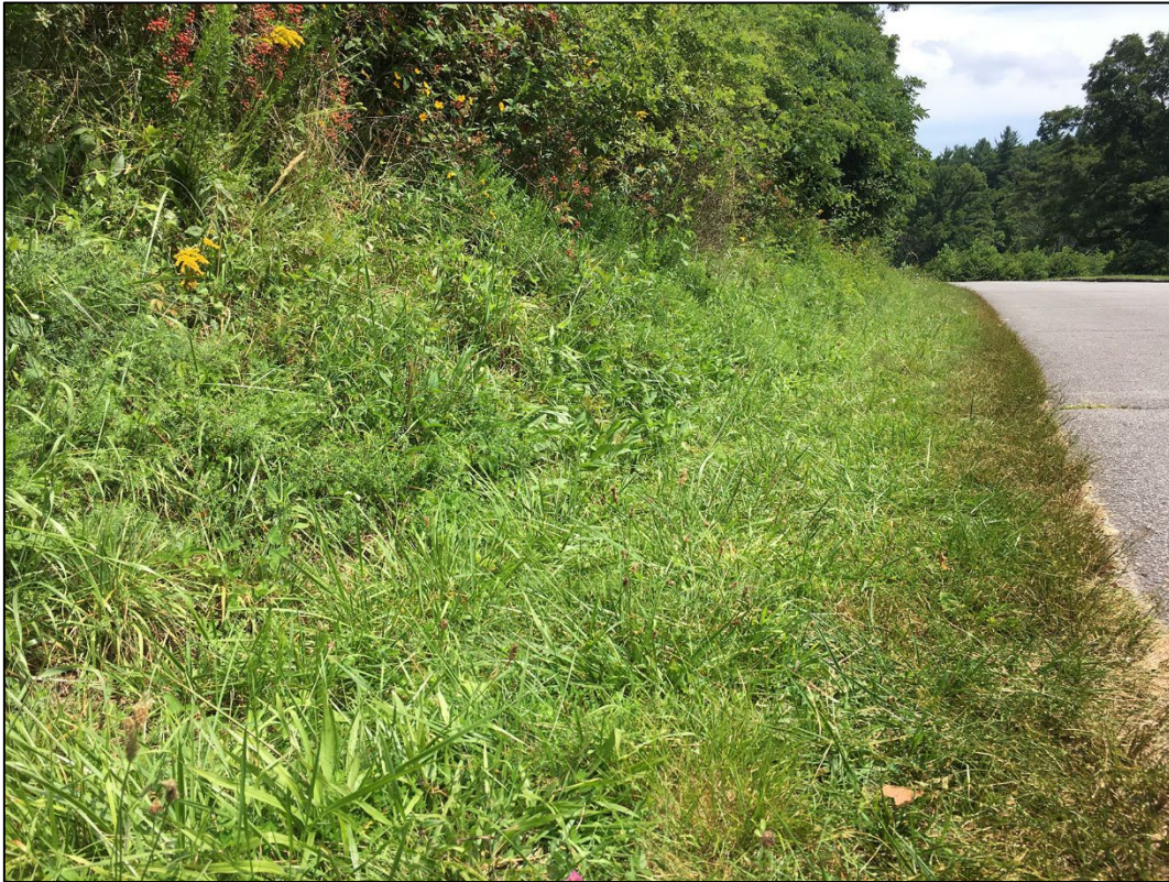
Fig 8-25. Stone gutter along Brinegar Cabin parking lot. Obscured by vegetation (2021)
